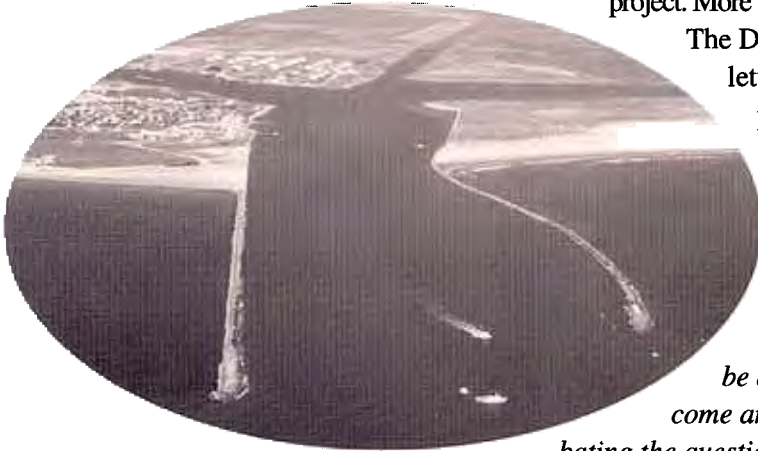
Harbor Island “Deeport” oil terminal proposal did not fare well and was later abandoned.
