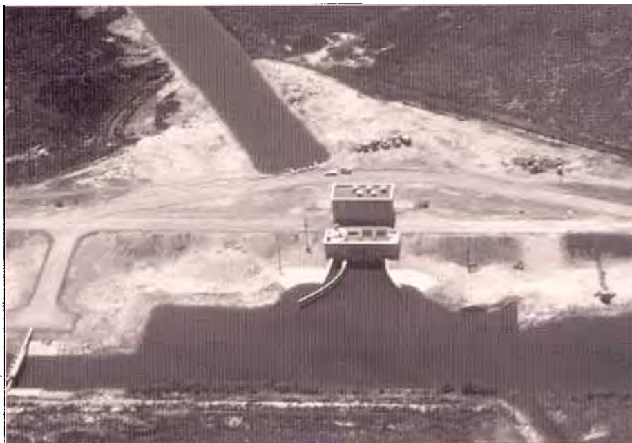
La Marque pump station drains floodwaters from areas behind the dikes.
