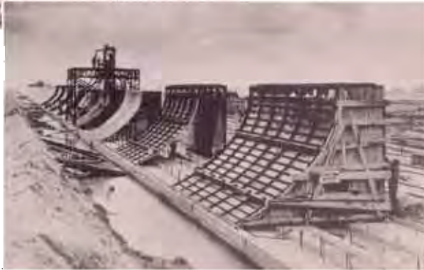
Right: The magnitude of the seawall sections is shown in this 1920 photo. Huge steel forms dwarf the workmen during the seawall's eastern extension.
