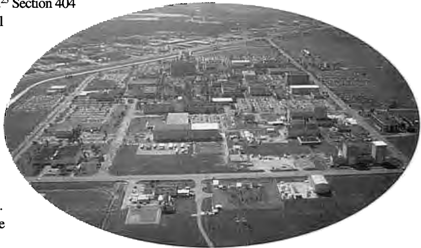
The Johnson Space Center (shown in a late 1980's photo) in Houston was constructed by the Fort Worth District, intensifying the rivalry between the two districts.
