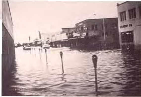
Right: Parking meters poke their heads above Hurricane Beulah's floodwaters in Edinburg, 1967.
