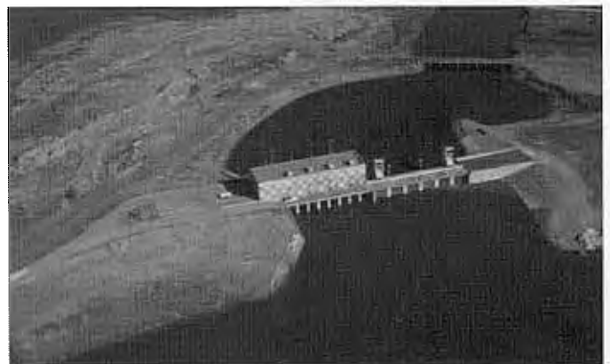
The pump station on Port Arthur Hurricane-Flood Protection System moves floodwaters out of Alligator Bayou.
