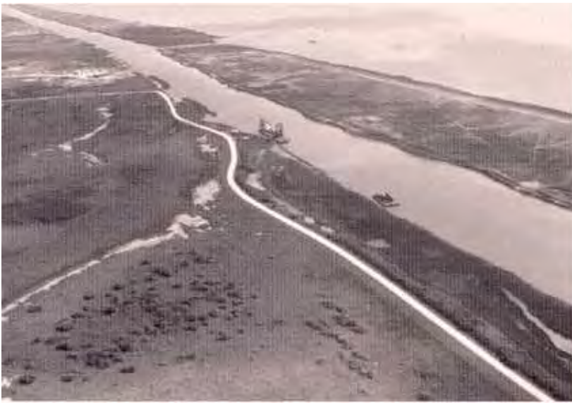
This photo shows dredging in East Matagorda Bay in 1983.
