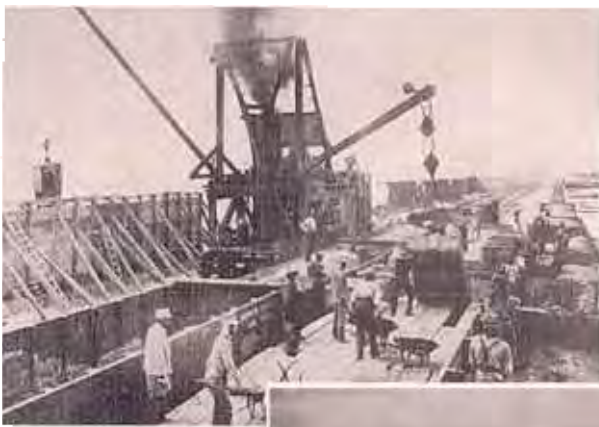
Above: An early photo shows seawall construction.
