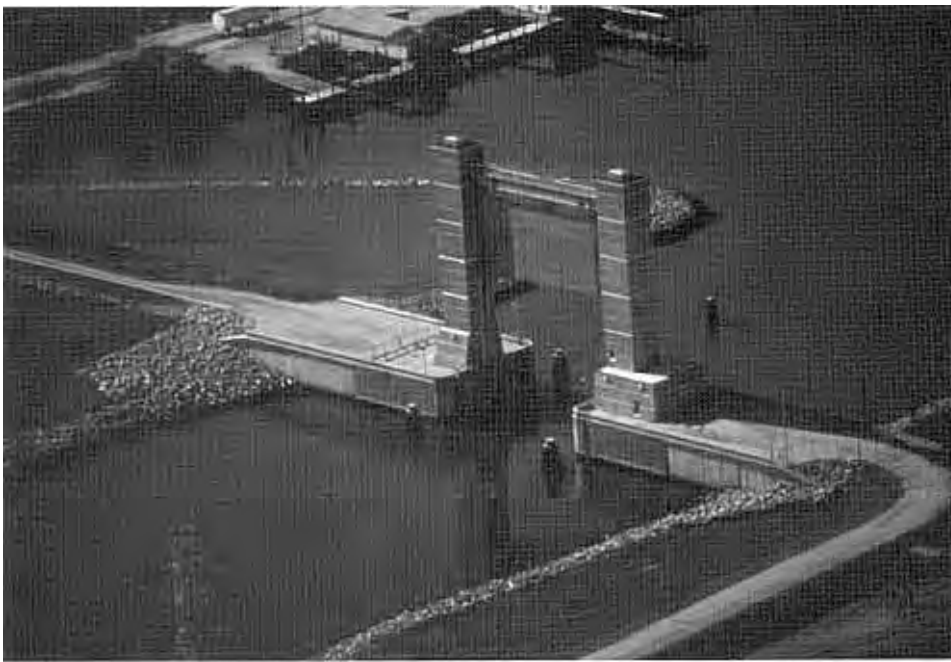
A “guillotine” tide gate is a landmark structure on the Freeport Hurricane-Flood Protection System.
