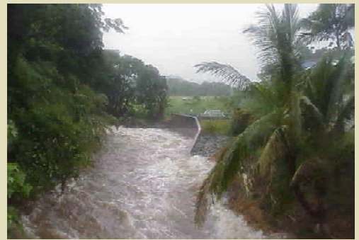
The Aleanio Flood Control Project on the Big Island, completed in 1997, nearly paid for itself in one flood event by preventing an estimated $12.2 million in damages in 2000.
