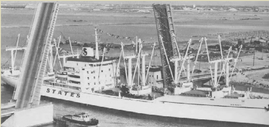
HED created the second entrance to Honolulu Harbor and built the bridge to join Sand Island and Honolulu. The bascule bridge, the first of its kind to be built in Hawaii, opened in April 1962 and was named for HED's first District Engineer, John R. Slattery.
