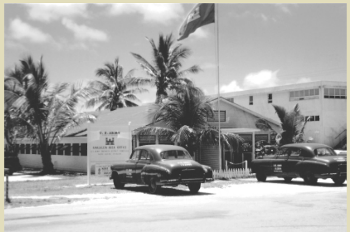
HED established the Kwajalein Resident Office in 1959. Kwajalein is now home to the Ronald Reagan Ballistic Missile Defense Test Site. HED has been instrumental in supporting the mission on Kwajalein as well as designing and building the facilities to house and support the 2,000 American civilian and military personnel who live there.
