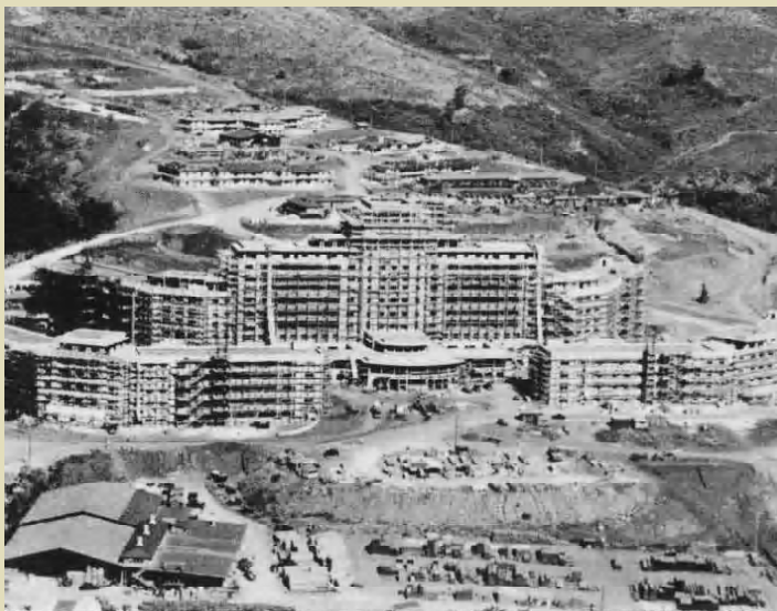
In 1948 HED completed one of Oahu's most famous landmarks, Tripler Army Medical Center (TAMC), at a cost of $40 million. To protect against earthquake damage, the 1,500-bed hospital was constructed as 12 independent buildings. For over 50 years, TAMC has been one of HED's biggest customers. HED has been responsible for numerous additional renovations to TAMC.
