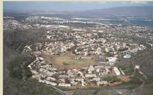
Aliamanu Military Reservation housing, one of HED's biggest family housing projects, was completed in 1978. HED built 2,600 units for $113 million, overcoming unique challenges of the terrain and geology of the crater.
