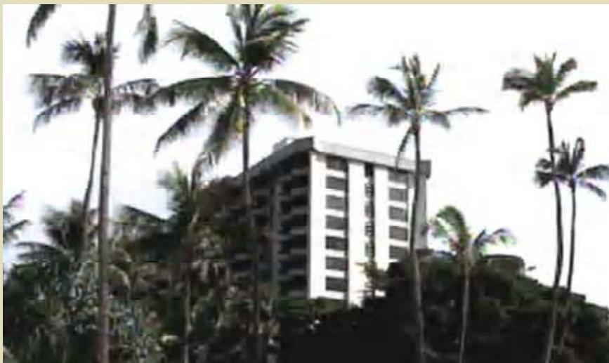
In 1973 HED began construction on the Hale Koa Hotel in Waikiki. Since then, many additions including the second tower and parking structure have been added. Thousands of military members and their families enjoy the facility each year.
