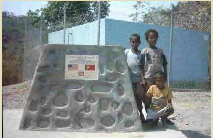
HED partnered with the Australia Agency for International Development to build a community water system in East Timor thus eliminating the water-borne disease problems which had plagued the 650 residents of Lotan Village.
