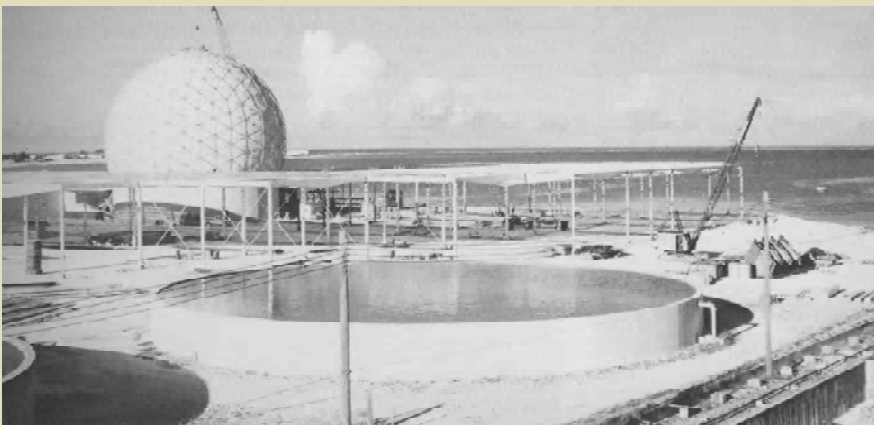
The Zeus acquisition radar receiver antenna and the horizontal ground plane complex on Kwajalein Island were completed in 1962 along with a transmitter building. The receiver building contains 22,255 sq. ft. of floor space.
