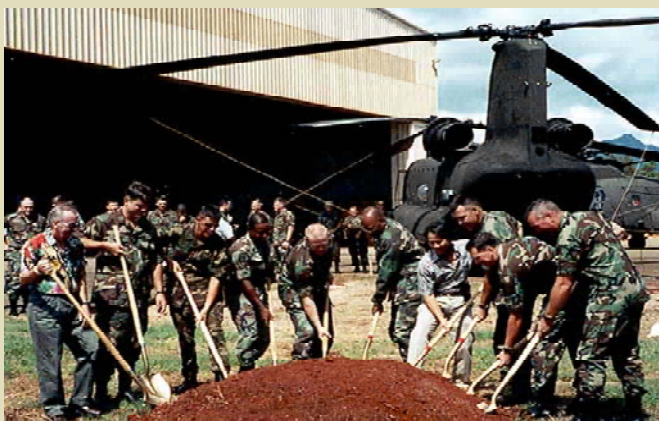
In August 1999 ground was broken on the facilities for the CH-47D Chinook helicopters for B Company, 214th Aviation Regiment (B/214th) at Wheeler Army Airfield. The $5.6 million project included a new hangar, renovation of the existing hangar, taxiway and aprons. Wheeler's original World War II-era runway could not support the 25-ton load generated by the helicopters.
