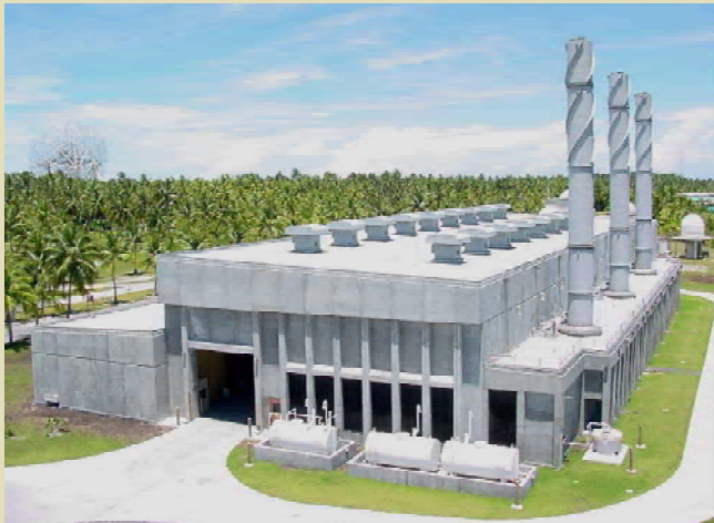
HED's Kwajalein Resident Office oversaw the building of the 13.5 megawatt power plant on the Kwajalein Atoll Island of Roi Namur. The 34,000 sq. ft. facility houses nine 1,500 kilowatt diesel engine-generator sets with state-of-the-art controls. It was completed in 2001, two months ahead of schedule.
