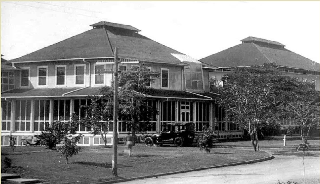
The original Tripler Hospital, Fort Shafter, Palm Circle, circa 1920. The hospital, built in 1907 was redesignated as Tripler General Hospital in 1920, honoring Brig. Gen. Charles Tripler, author of "Manual of the Medical Officer of the United States Army."
