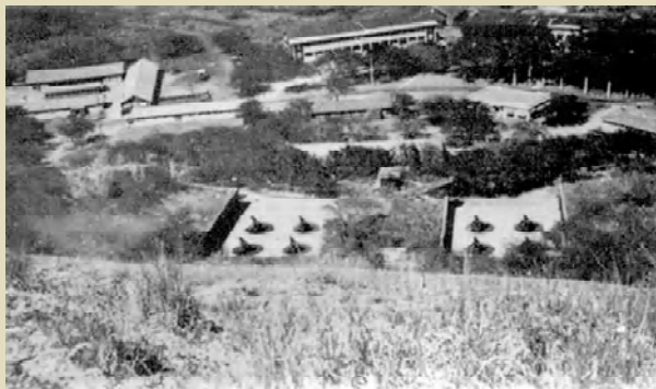
(L & R) Oahu's first coastal fortification, Battery Harlow at Ft. Ruger, circa 1924: HED built Battery Harlow in 1910 at Diamond Head. Its eight 12-inch guns were contained in two concrete pits which were praised for their strength. When the guns were test-fired, only one small crack appeared in the concrete.
