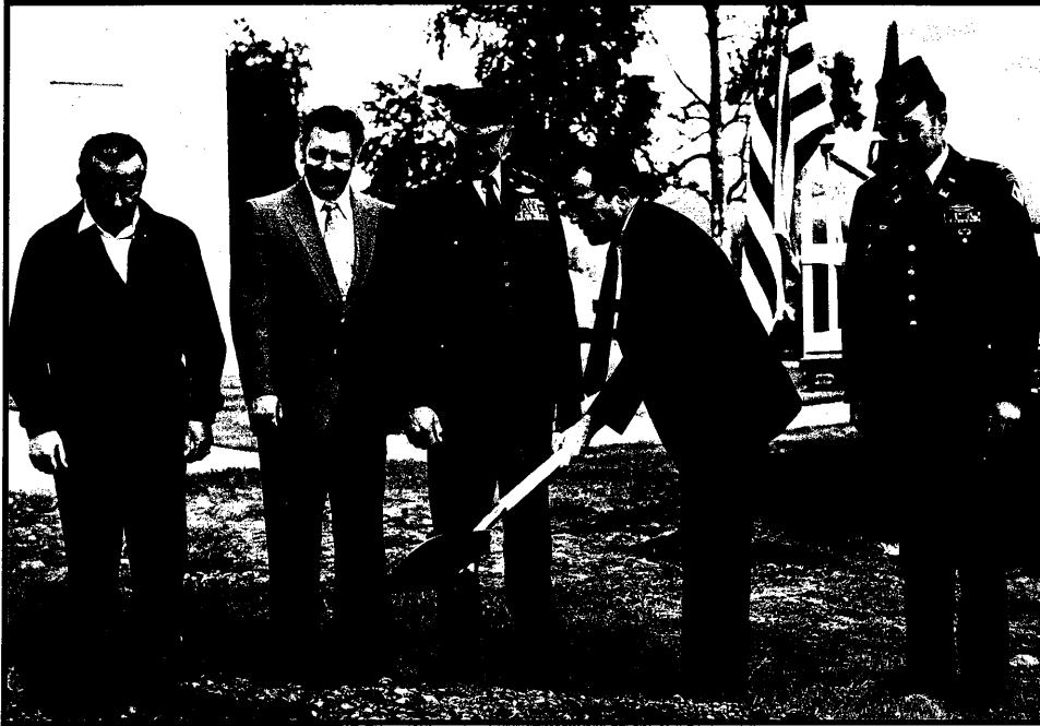
Senator Ted Stevens breaks ground for the Corps' largest construction project in 1980 — the Regional Operations Control Center for the Alaskan Air Command. Observing are (left to right) Joe Russell, manager, and Ed Young, president, of Interstate Co., Inc., the contracting company ; Lt. Gen. Winfield W. Scott, Jr., Commander, Alaskan Air Command; and Col. Lee R. Nunn, District Engineer.
