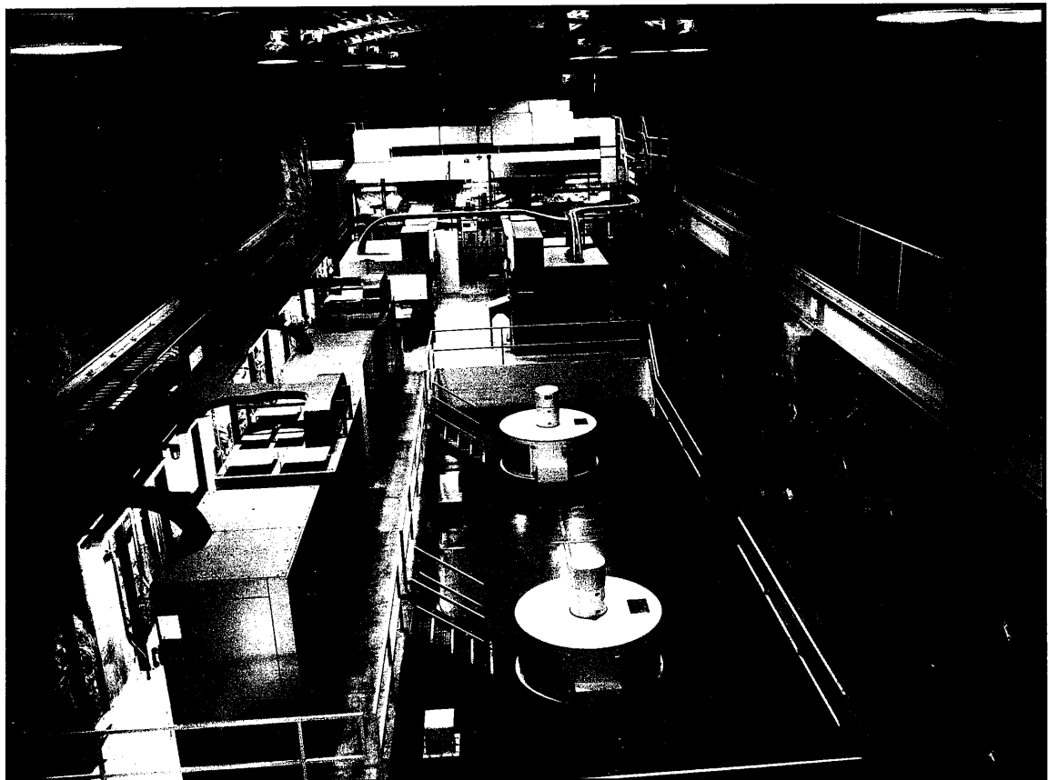
Interior, Powerhouse, Snettisham Hydroelectric Project.
