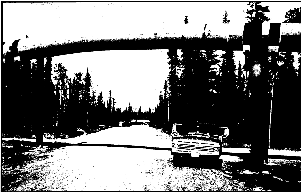
Trans-Alaska Pipeline System.
