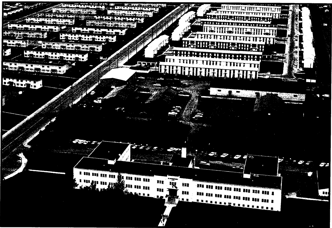
Alaska District headquarters (foreground) and 8-plex housing at Elmendorf, 1965.
