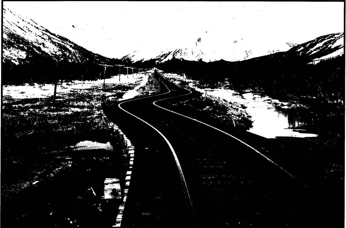
Railroad track warped by earthquake land movement near Portage.
