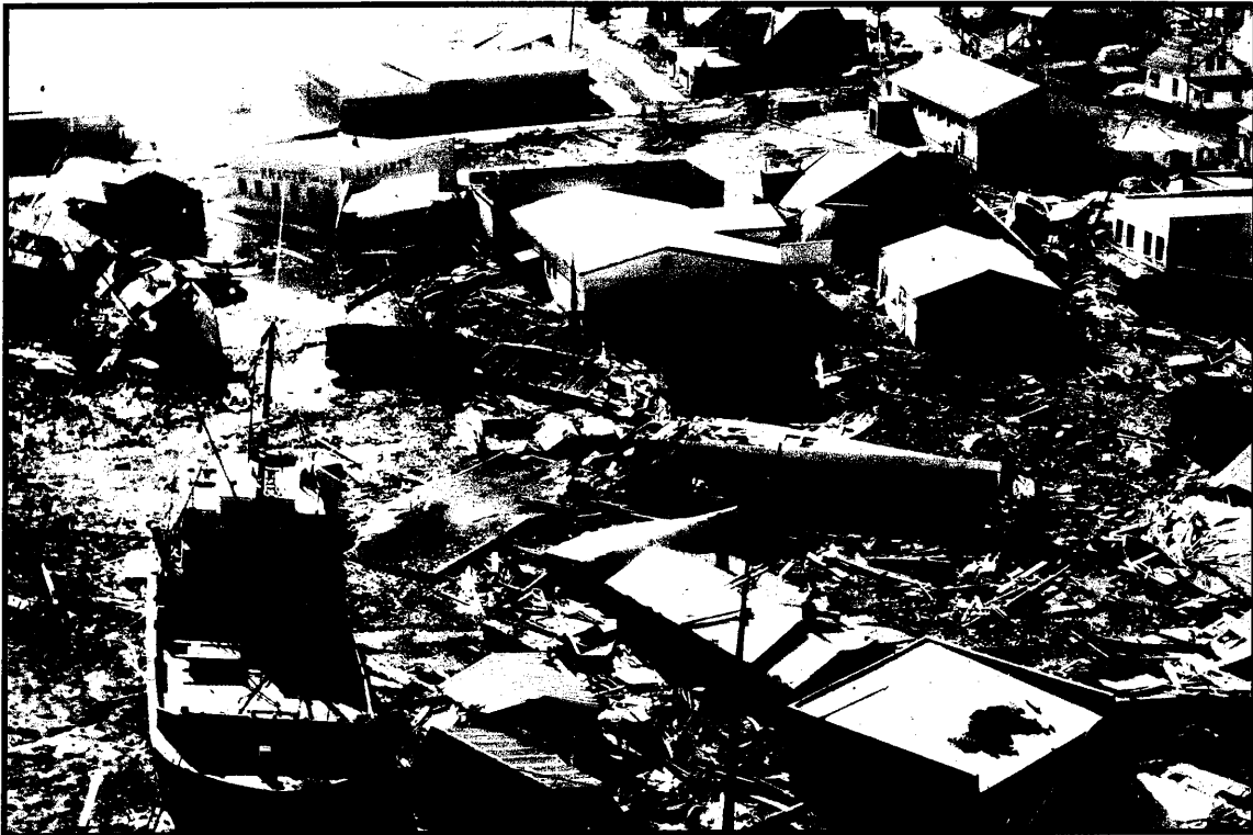
Earthquake damage at Anchorage small-boat harbor. Part of the fishing fleet is shown deposited among the scattered business and warehouse buildings.
