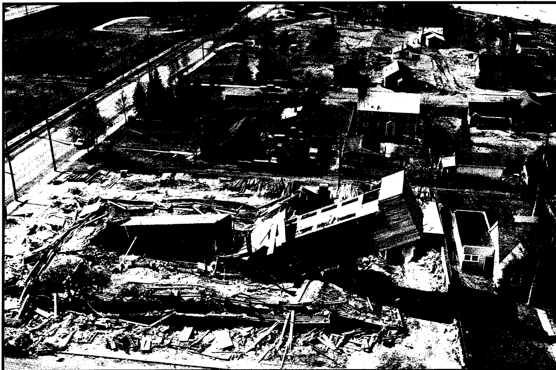
Direct earthquake damage to the Four Seasons Apartment Building, Anchorage.
