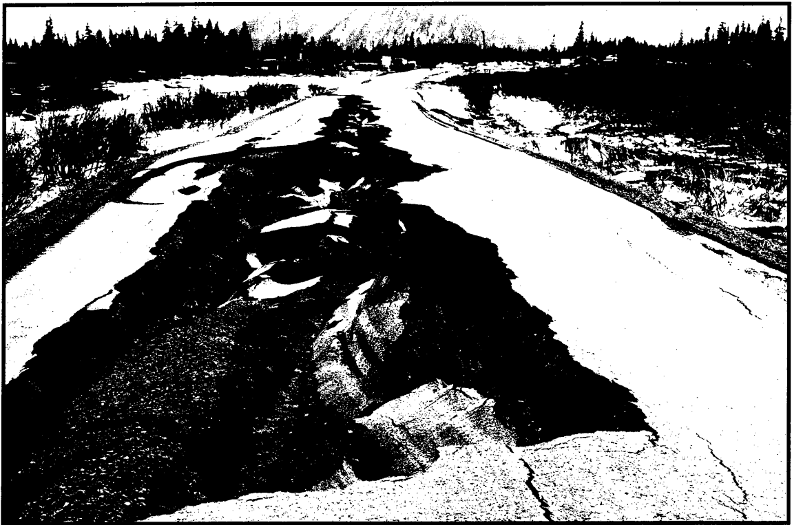
Earthquake damage to highway near Portage.
