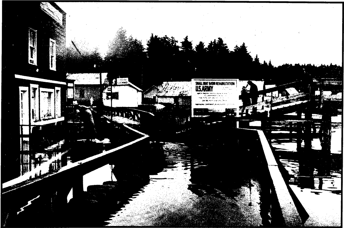
Seldovia, boardwalk at high tide in October 1964.
