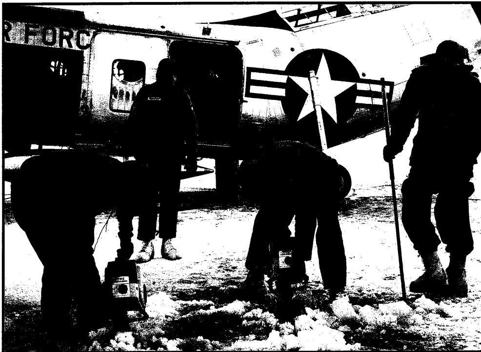
Cutting holes to place ice-blasting charges for flood prevention, 1966.
