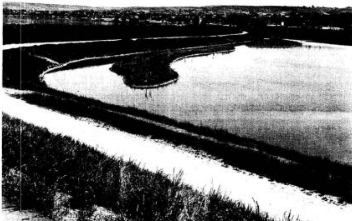
WEST LEWISTON LEVEE
