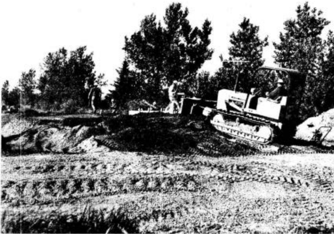
WILLOW CREEK DAM CONSTRUCTION JUNE 1980
