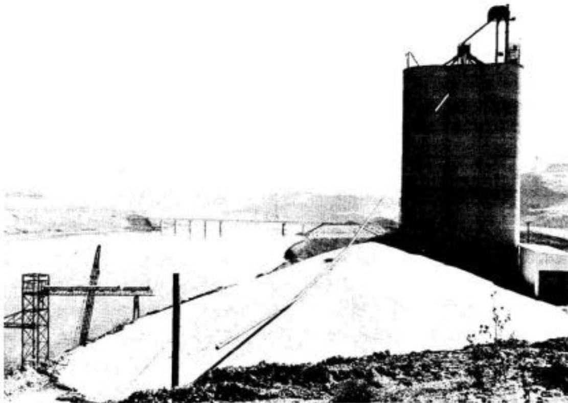
PORT OF COLUMBIA GRAIN ELEVATOR
