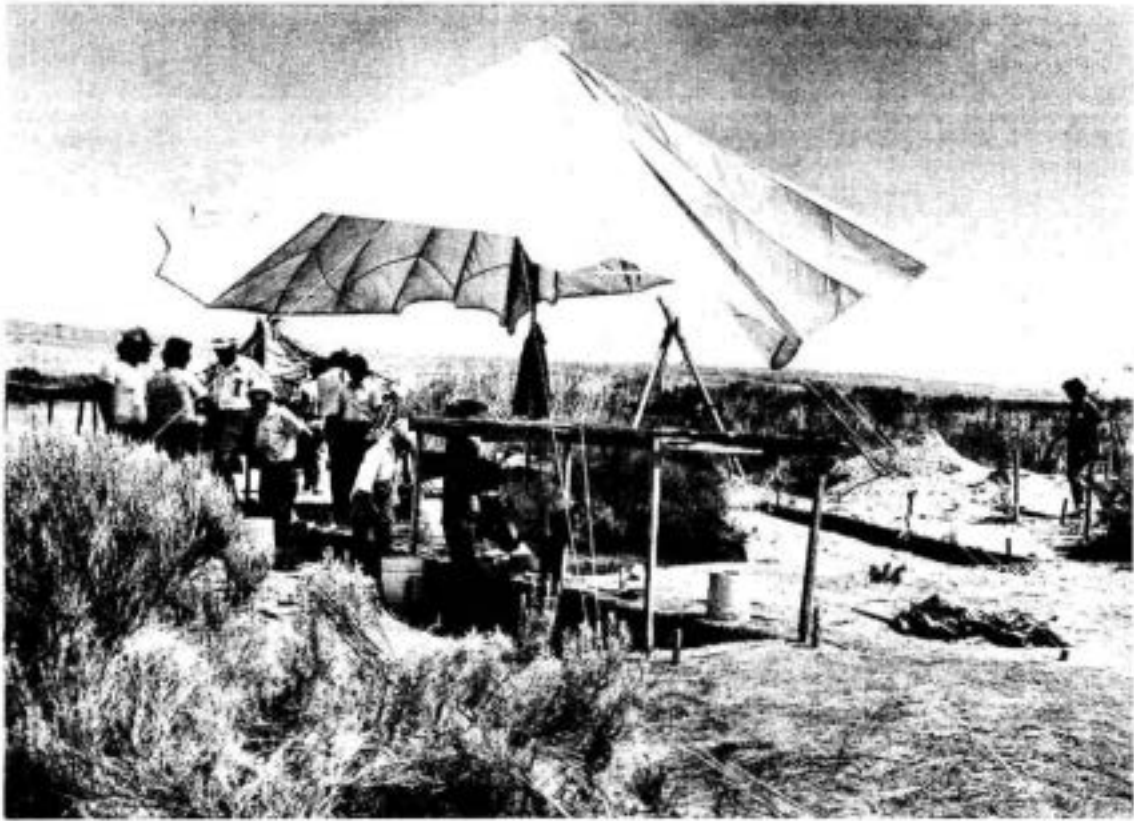
OPEN TRENCH EXCAVATION WORK AREA AT STRAWBERRY ISLAND PROTECTED FROM SUN BY PARACHUTE
