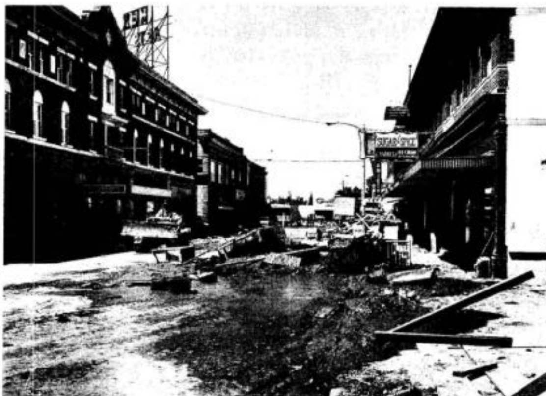
DEBRIS CLEANUP AT REXBURG
