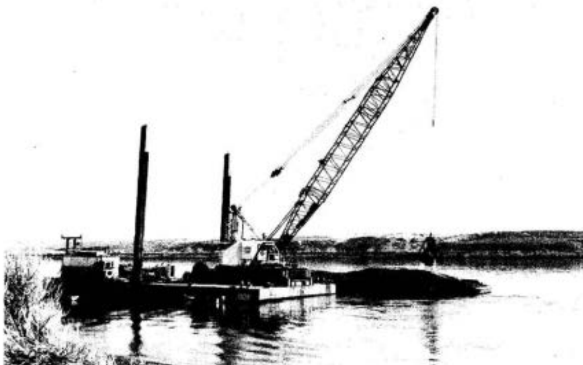
USING DREDGED MATERIAL TO BUILD A GOOSE NESTING AREA NEAR McNARY DAM, 1978
