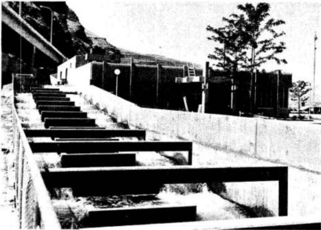
FISH LADDERS AT LOWER GRANITE DAM
