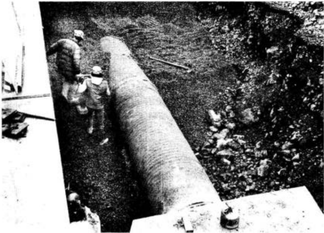
INSTALLING A FINGERLING BYPASS PIPE AT LITTLE GOOSE DAM 1979
