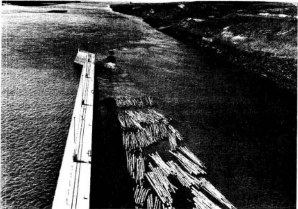
LOGS HEADING DOWNSTREAM ICE HARBOR LOCK
