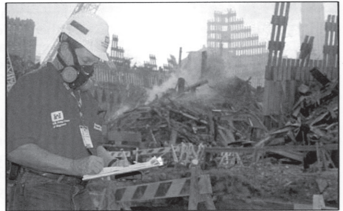
Emergency response personnel in most of lower Manhattan used dust masks, but those working in the rubble needed respirators to protect them from the thicker dust and potential hazards and any contaminants.
