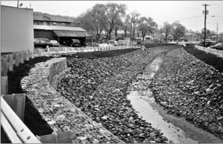
A section of the Molly Ann's Brook Flood Control Project
