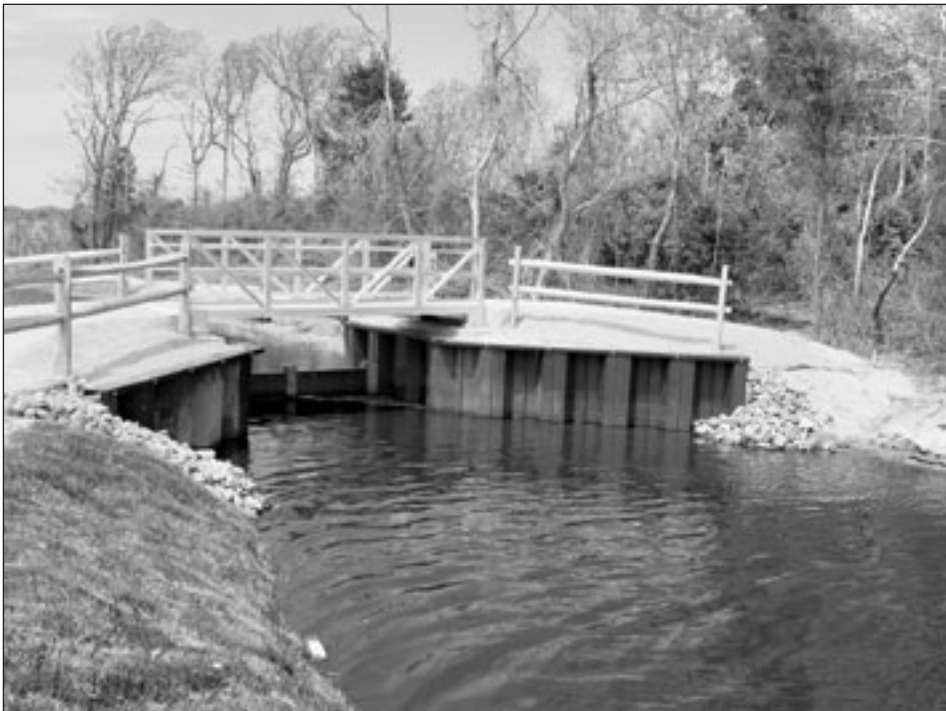
Self-regulating tide gate within the Meadows
