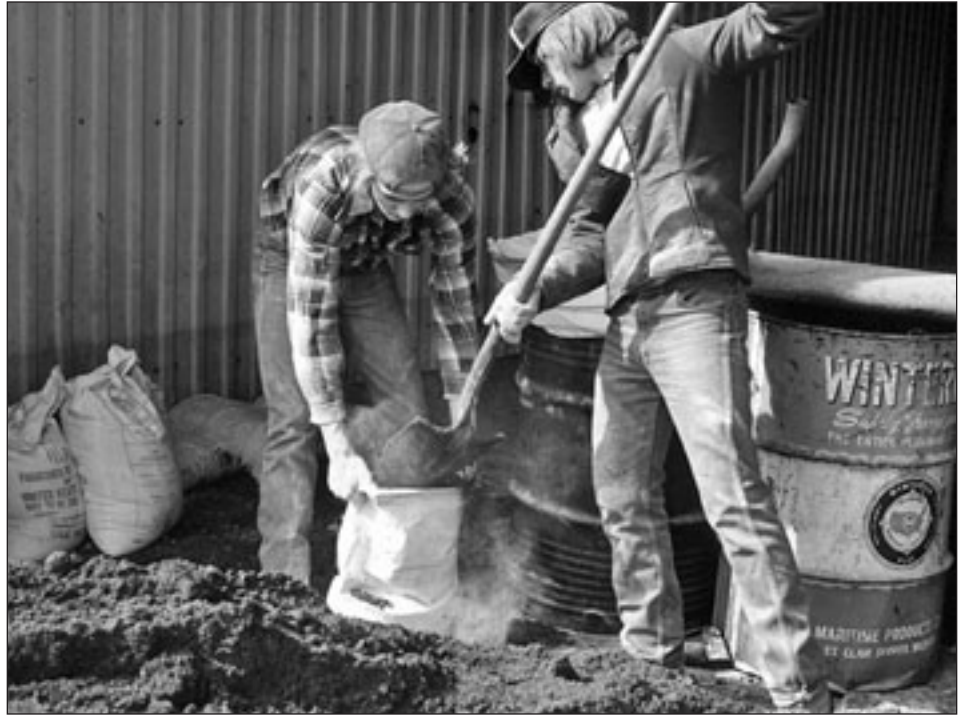
Filling sandbags for flood-fighting
