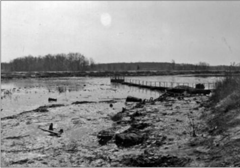
The Bridgeport Rental & Oil Services Superfund site, Bridgeport, N.J., before remediation. It was once rated the most challenging cleanup on EPA's National Priorities List
