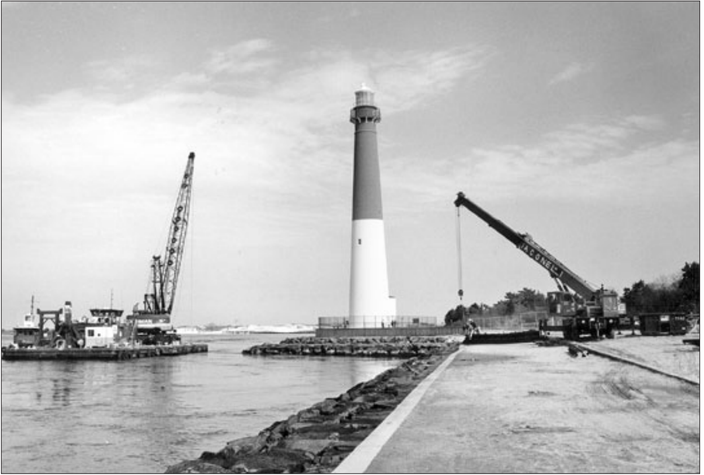
Improving erosion protection around Barnegat Light
