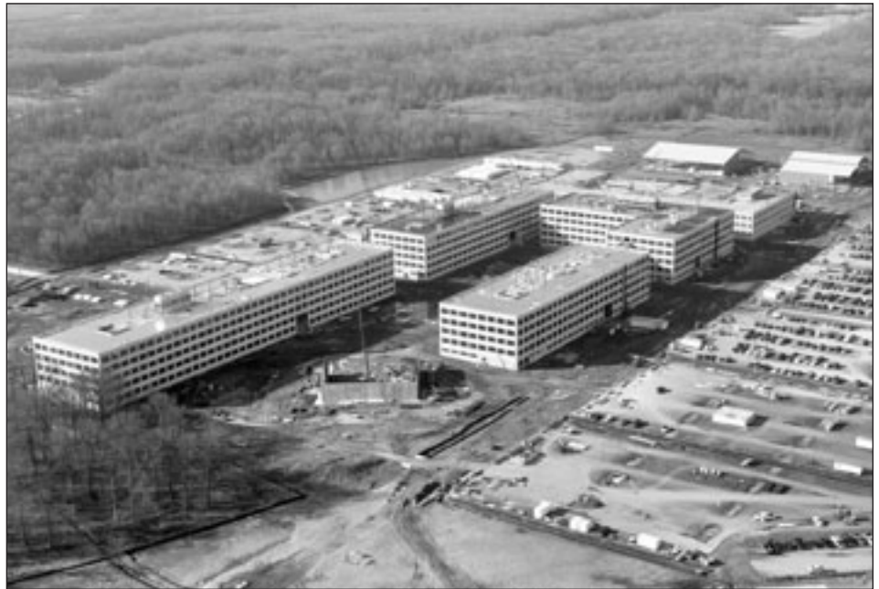
New facilities under construction at Aberdeen Proving Ground, Md., in 2008 for relocation of the Army's Team C4ISR from Fort Monmouth, N.J.
