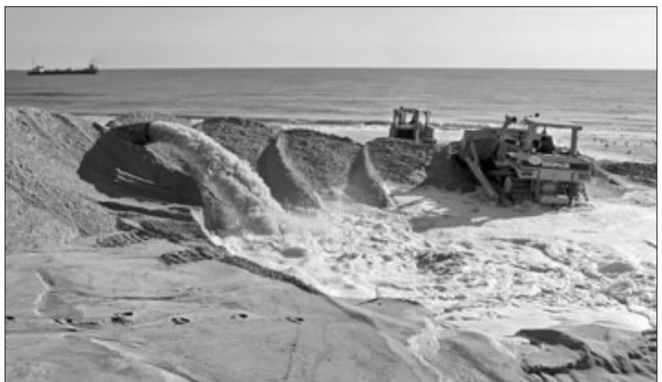
Initial beach nourishment at Surf City along New Jersey’s Long Beach Island
