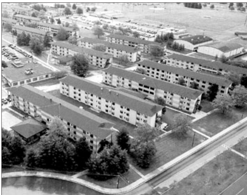
Renovated barracks at Fort Dix
