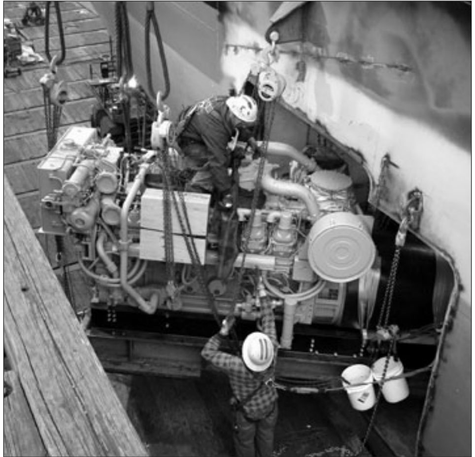
Installing an engine on a hopper dredge
