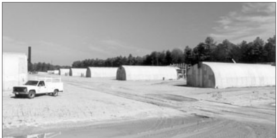
Ammunition Storage Facility, Fort Dix
