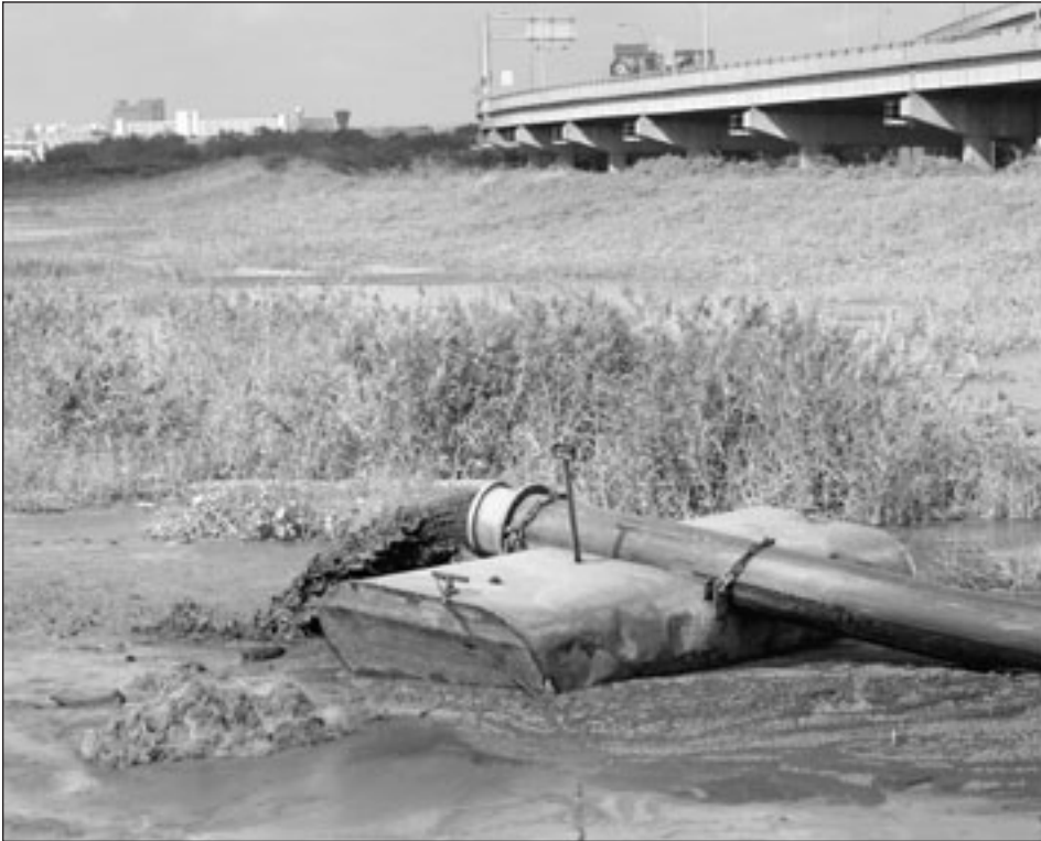
Depositing of dredged material via pipeline at the Fort Mifflin CDF
