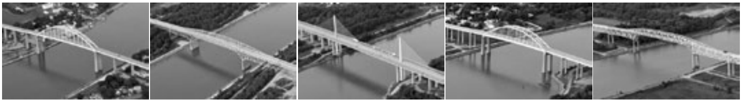
Chesapeake City Bridge
