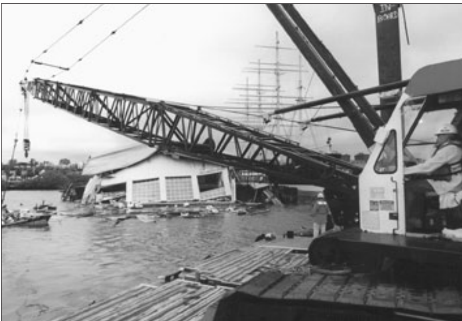
A crane from the Philadelphia District's labor and equipment force removes debris from the Pier 34 site
