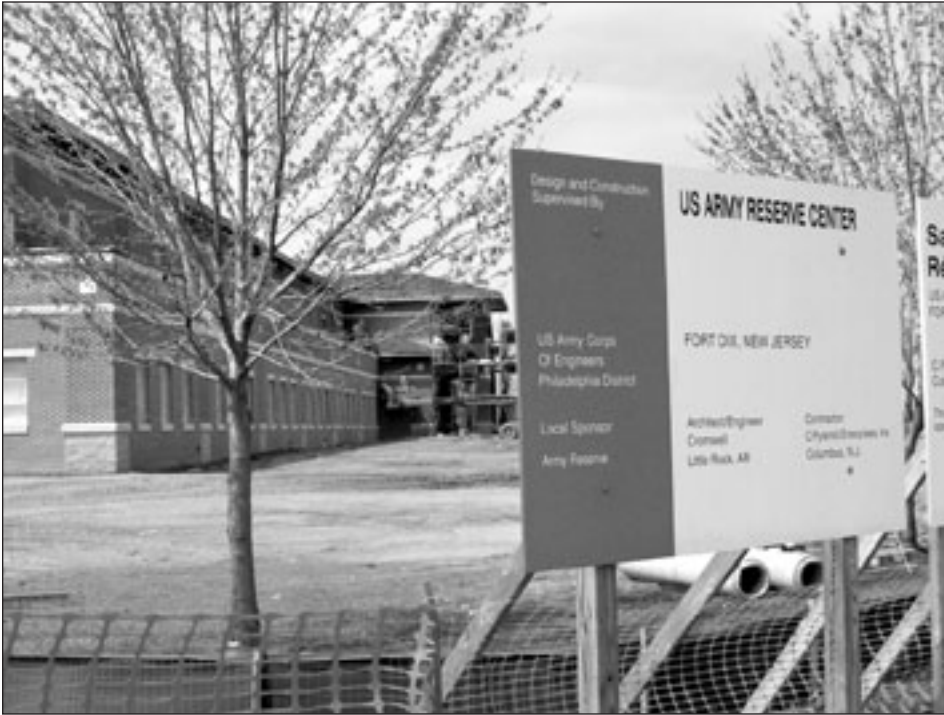
Construction of the US Army Reserve Center at Fort Dix, N.J., built to accommodate units from other installations being closed under BRAC 2005
