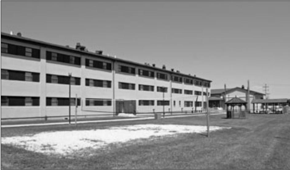
Fort Dix Annual Training Barracks, renovated by the District for the U.S. Army Reserve Command
