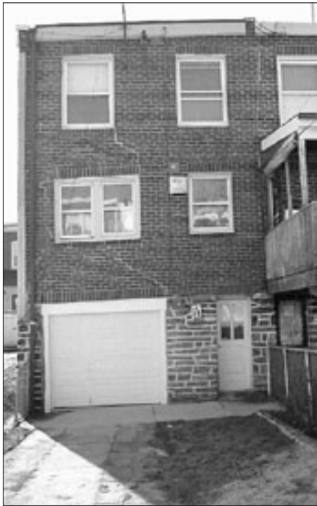
Visible settlement cracks characterized “sinking homes” such as this one in Philadelphia’s Wissinoming section
