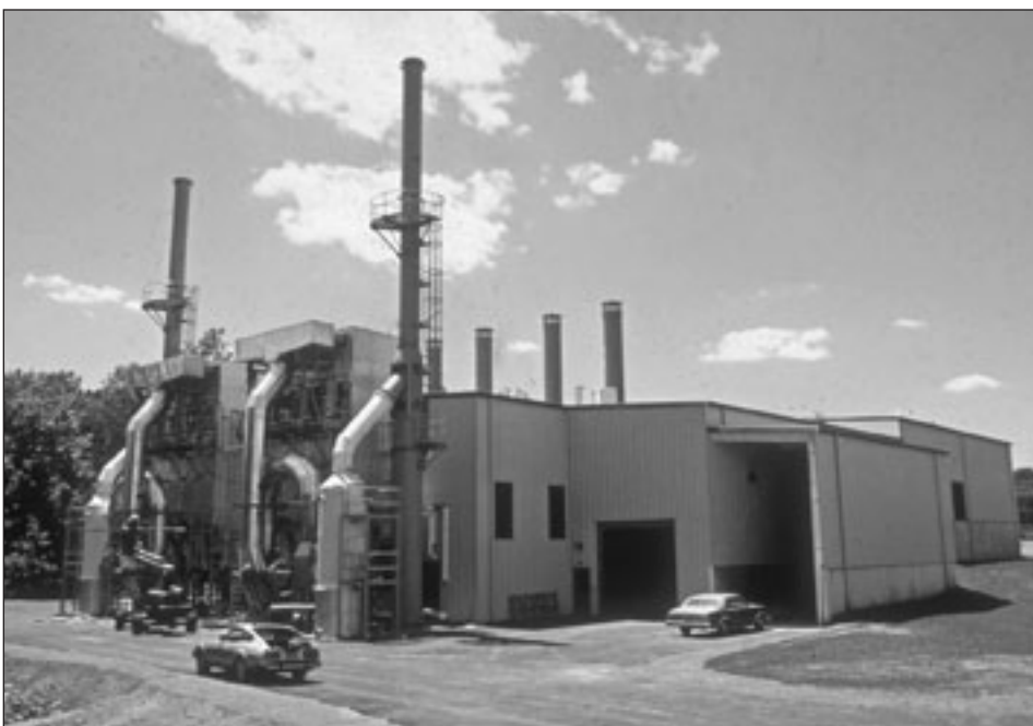
Resource Recovery Facility, Fort Dix
