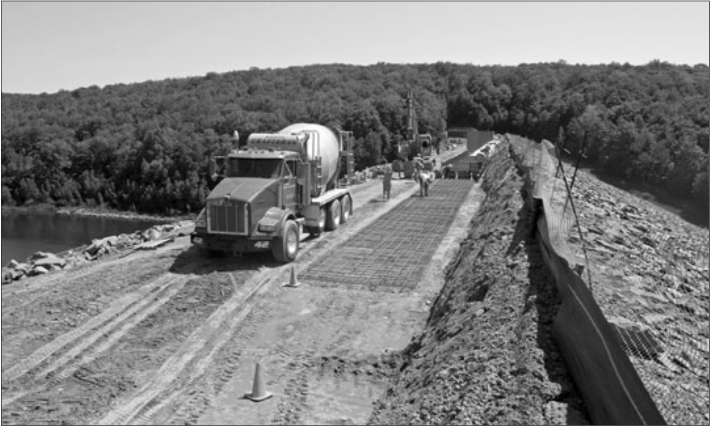
Construction of safety modifications to Prompton Dam in 2007
