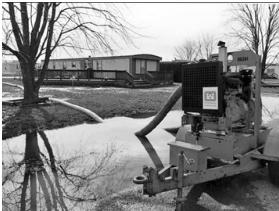
Emergency equipment on loan from the Philadelphia District pumps down flood waters in Sussex County, Del.
