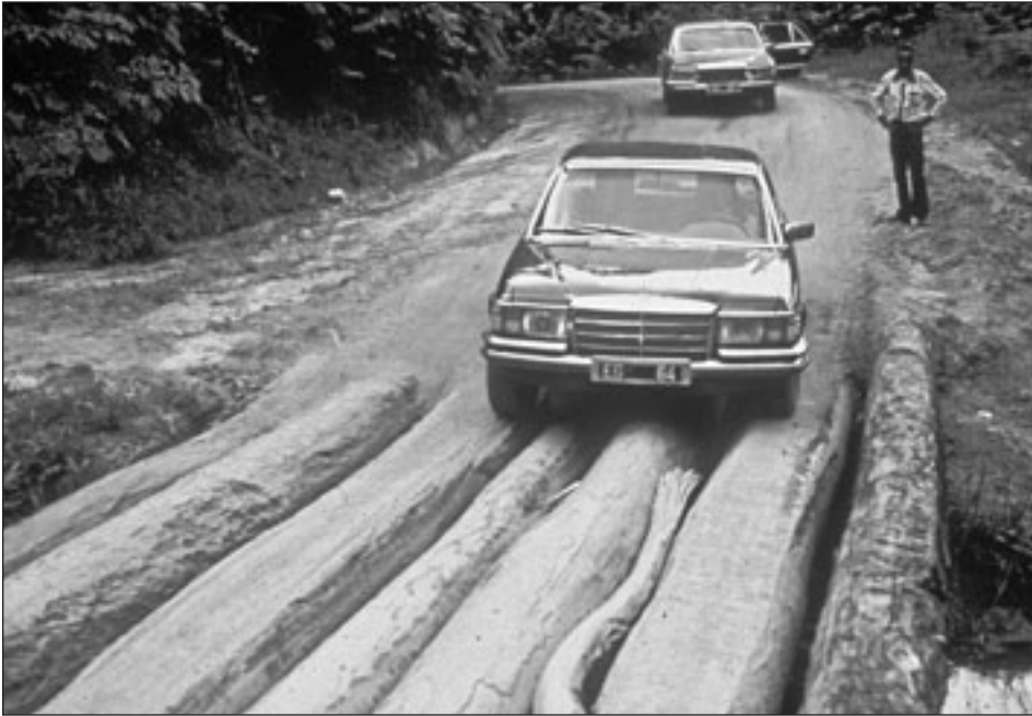
Bridge conditions in Gabon
