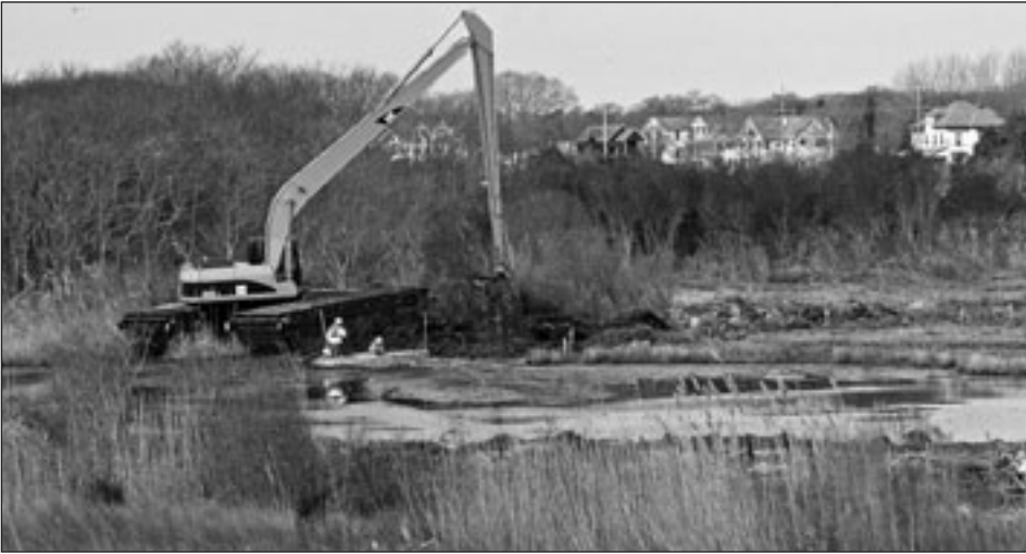
Work at Lower Cape May Meadows included reditching to restore natural stream flows (above) and replanting of native vegetation (below)
