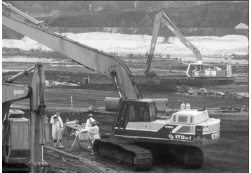
Remediation at the Bridgeport Rental & Oil Services Superfund Site, Bridgeport, N.J.
