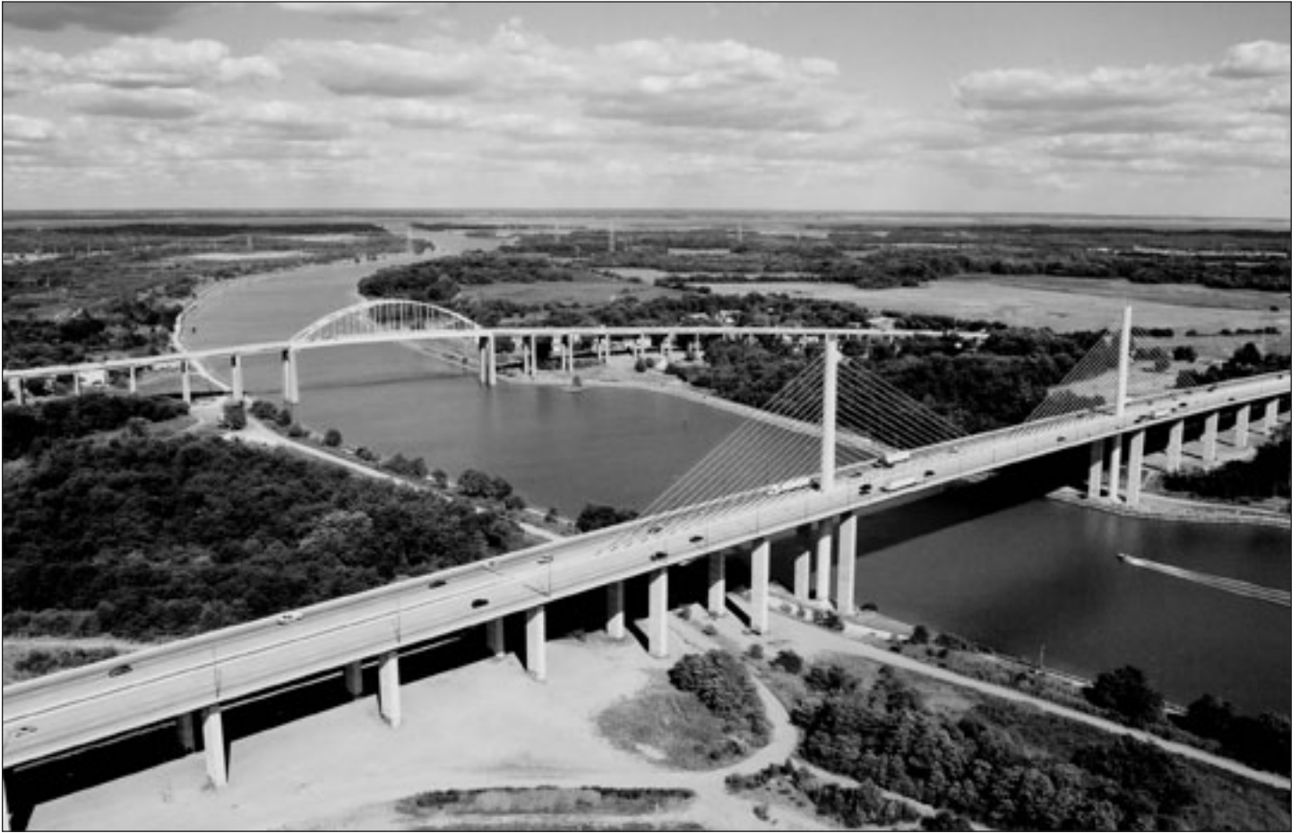
In 1995, a new state-owned bridge (foreground), later named after Senator William V. Roth, Jr., came alongside the Corps' St. Georges Bridge (background) as the primary span across the C&D Canal. Congress transferred it to the Corps in 2007
