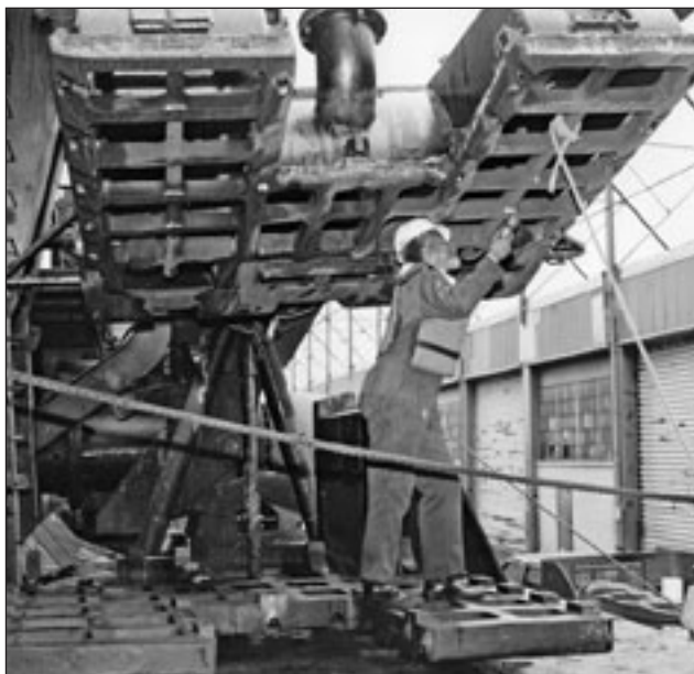
Routine dragarm inspection
