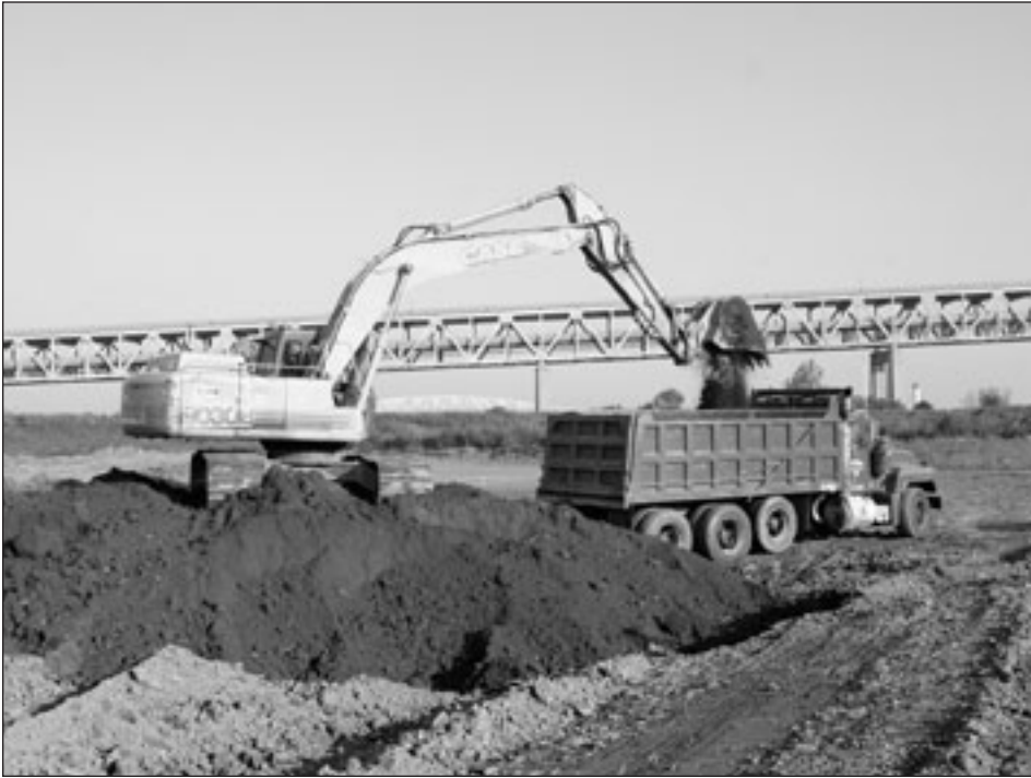
Loading of dried-out dredged material to be transported offsite by third parties for beneficial re-use
