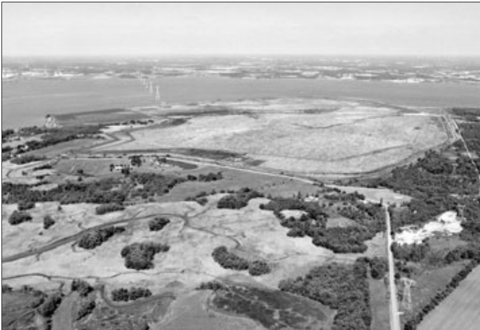
Kilcohook Confined Disposal Facility, one of eight Corps-owned and operated sites for dredged material from the Delaware River, Philadelphia to Sea federal navigation channel
