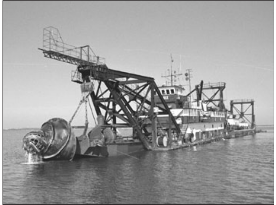
Dredging in the Delaware River, Philadelphia-to-Sea federal navigation channel
