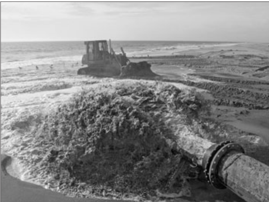
Sand being pumped ashore for beach nourishment at Cape May, N.J.
