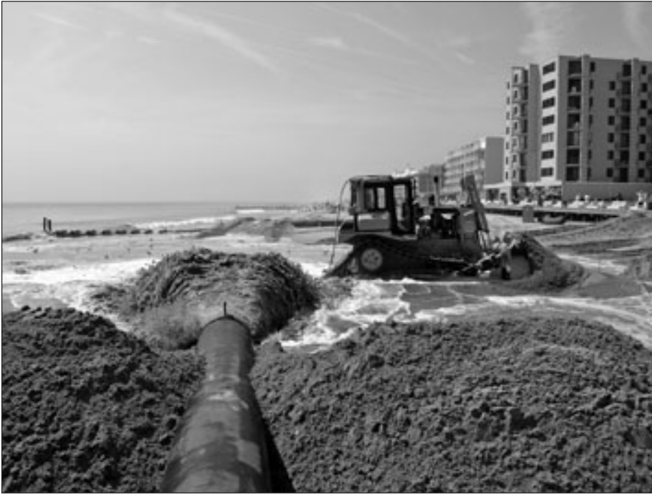
Beachfill operations at Rehoboth Beach, Del.
