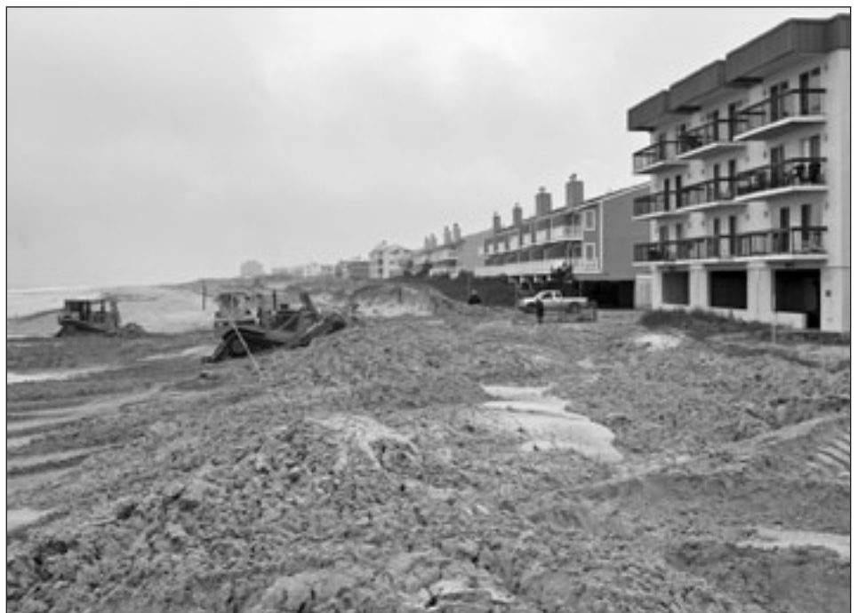
Initial beach nourishment at Brigantine, N.J.
