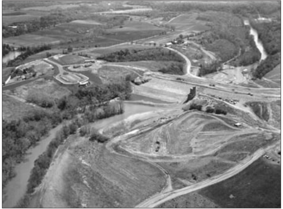
Aerial view of the Blue Marsh Dam under construction
