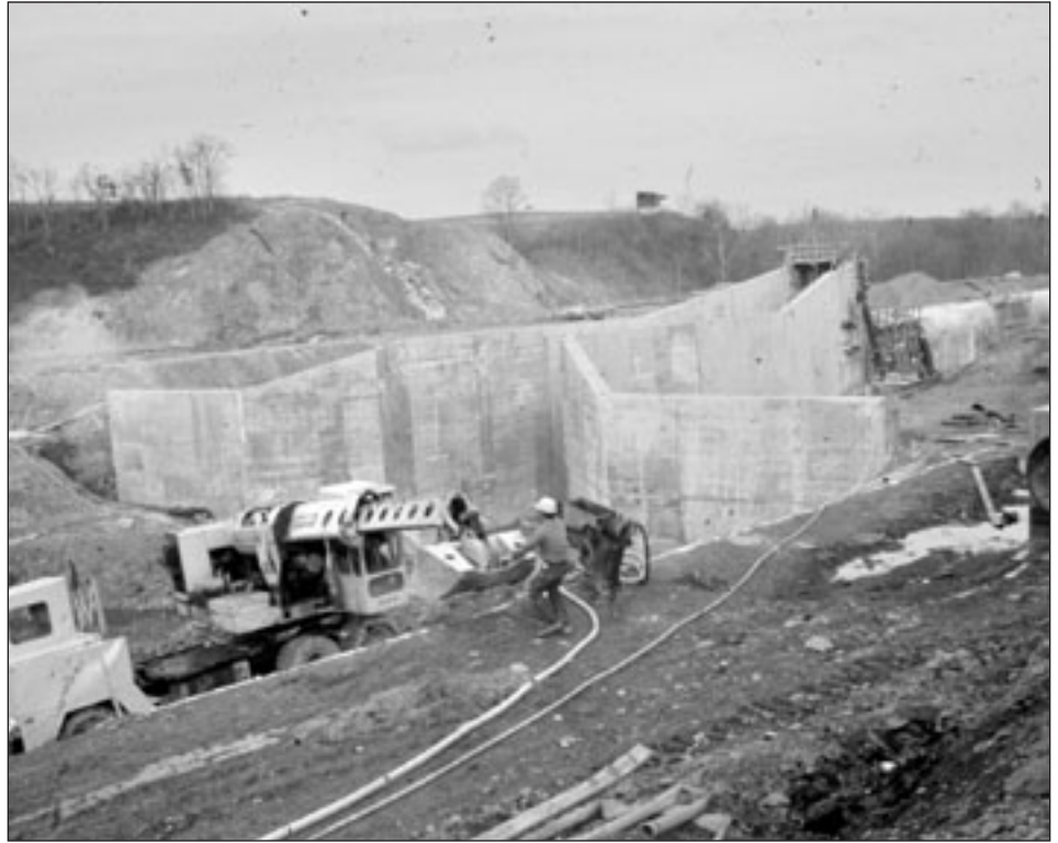
Construction of the Blue Marsh Dam
