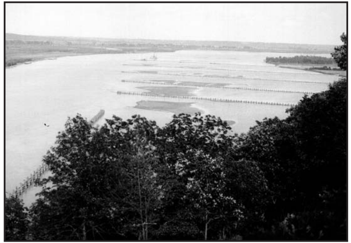
The Missouri River at Indian Cave Bend in Nebraska in 1935. The U.S. Army Corps of Engineers used the Missouri River to create its own navigational channel in many areas. Photo provided
