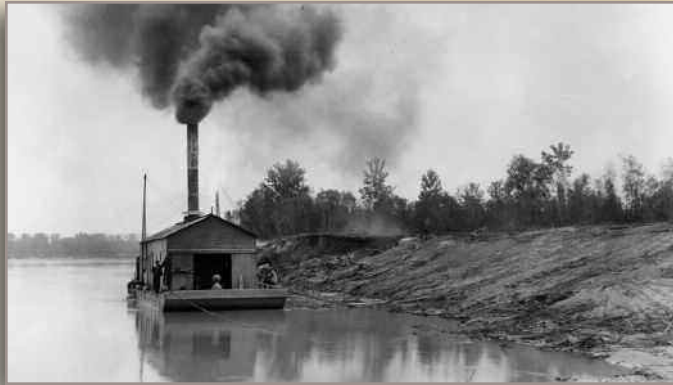
Hydraulic grading on bank
