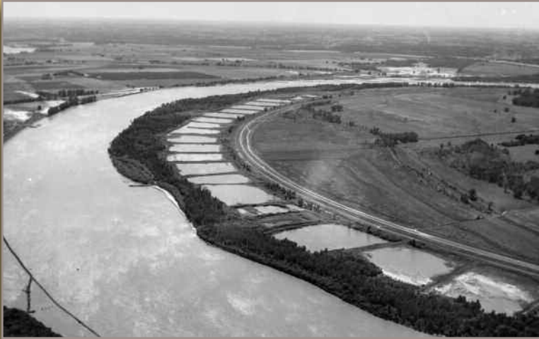
Aerial of Missouri River modifications, 1953
