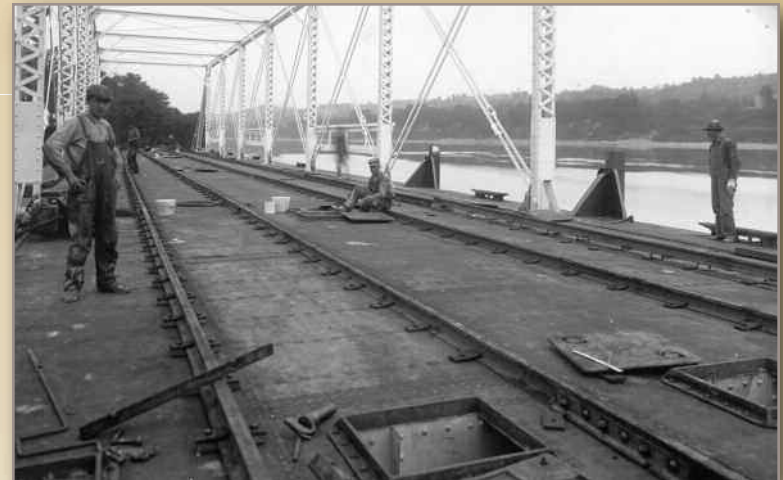
Workers taking a break during railroad bridge construction
