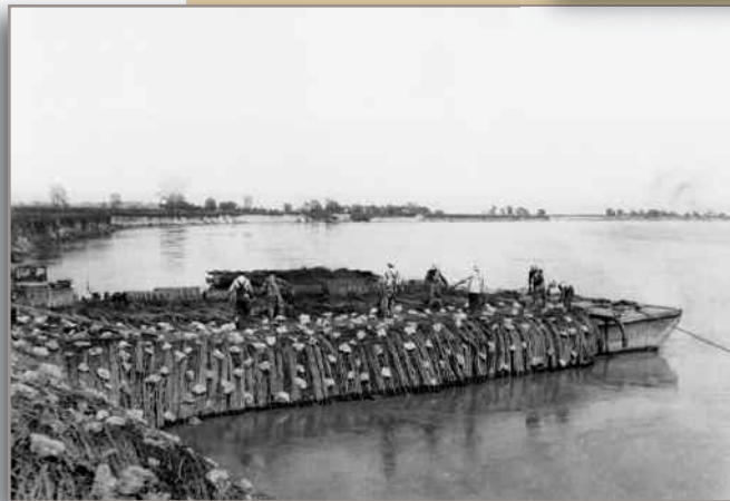
Workers build mattresses on a barge
