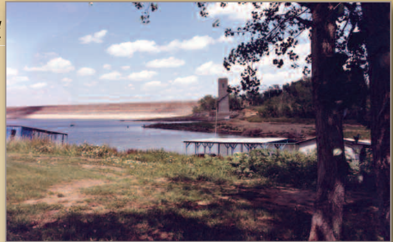
Newly completed Kanopolis Lake
