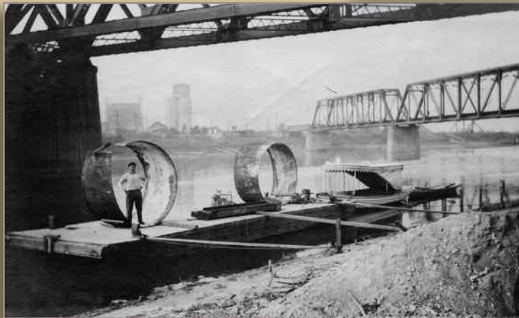
Steel rings and I-beam removed from tubes, August 27, 1913
