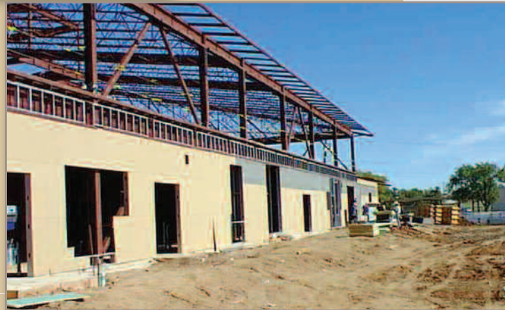
Construction at McConnell Air Force Base
