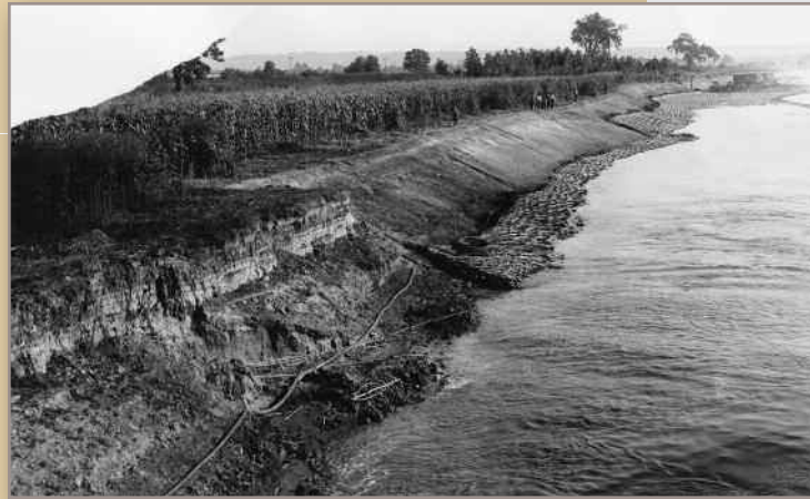
Caving bank partially graded, showing willow mat ready for paving stone
