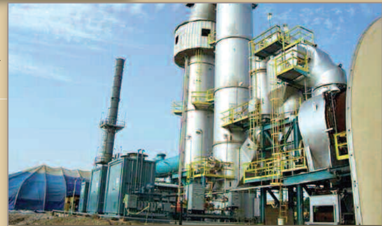
Cleanup and demolition of abandoned buildings at Weldon Springs
