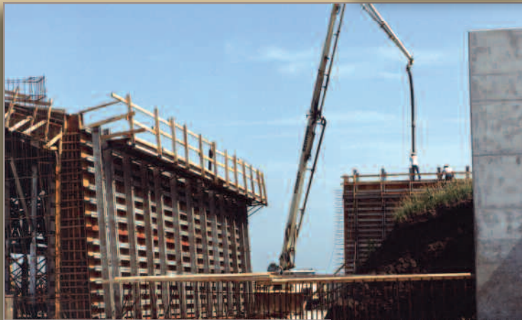
Construction of support facilities at Whiteman Air Force Base, 1993
