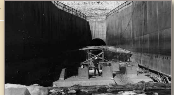
Construction of Pomona Dam, 1963
