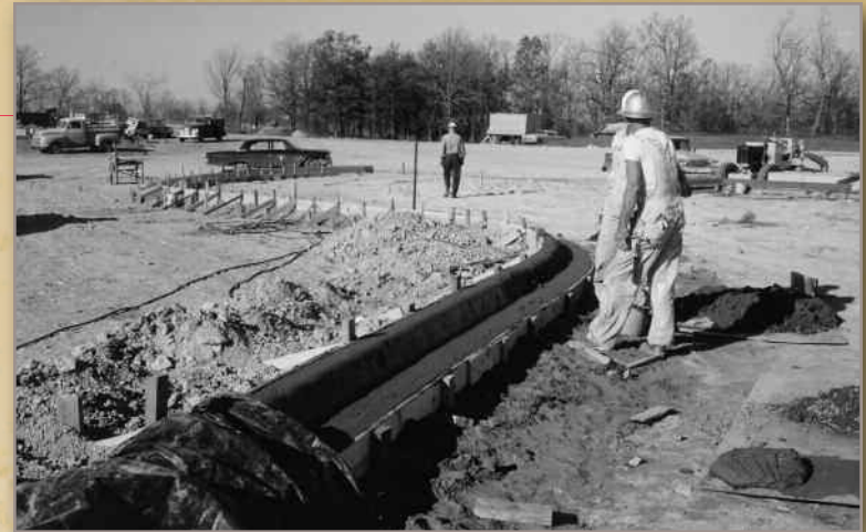
Curb and gutter construction at Stockton Dam, 1964
