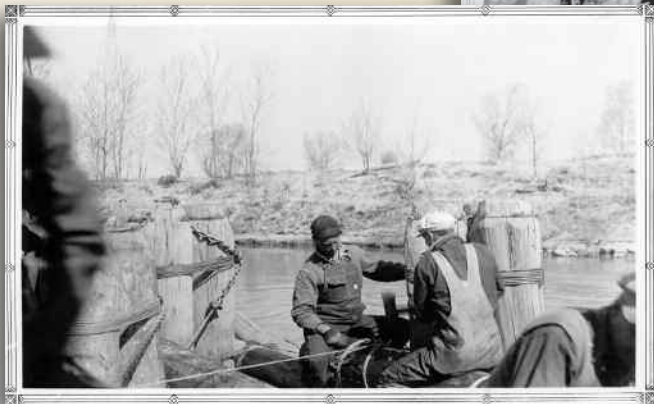
Workers making string dike, Camden Bend, 1936
