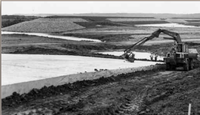
Construction at Clinton Lake, 1978
