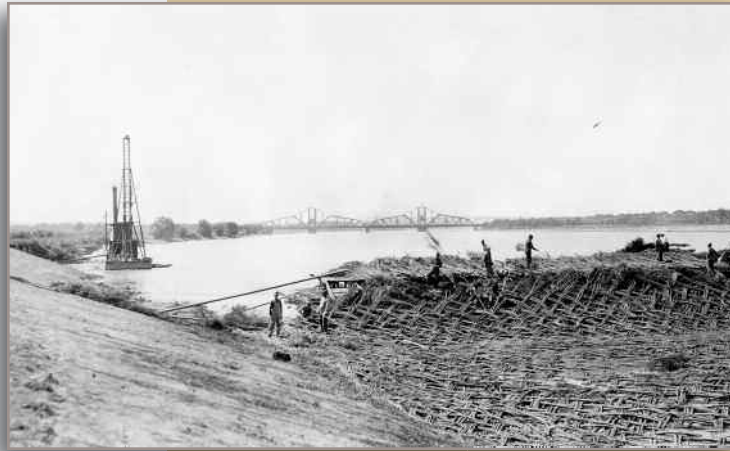
Constructing revetment weaving mattress and grade bank, Council Bluffs, IA
