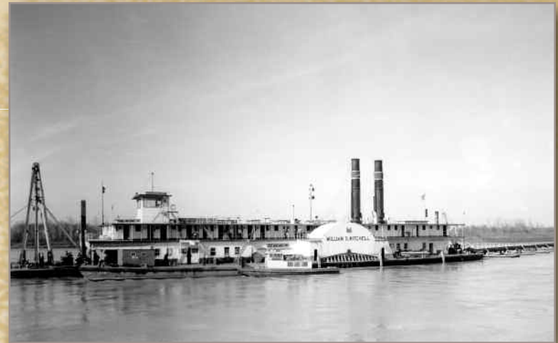
William Mitchell dredge boat. Operational in April of 1938 at Baltimore Bend of the Missouri
