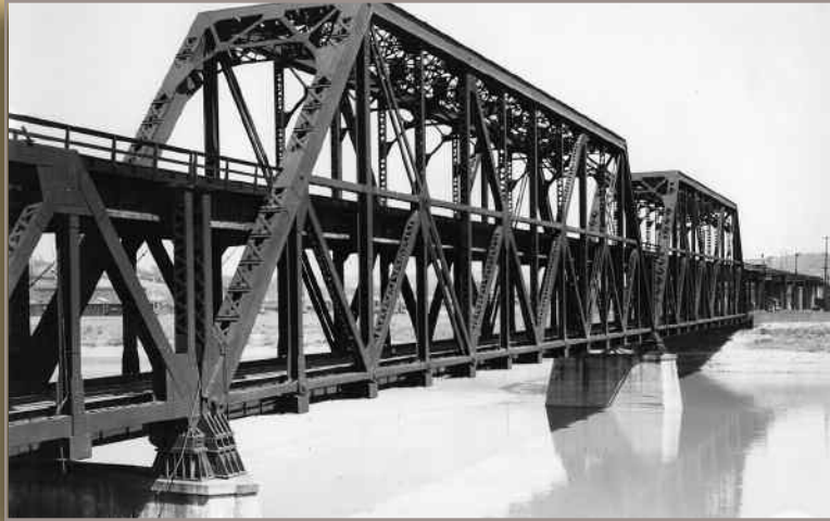
Truss railroad bridge over Kansas River, 1945
