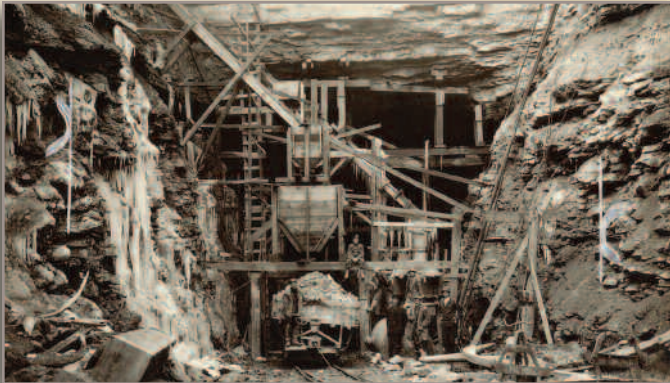
Kansas City constructed the Turkey Creek Tunnel in 1919
