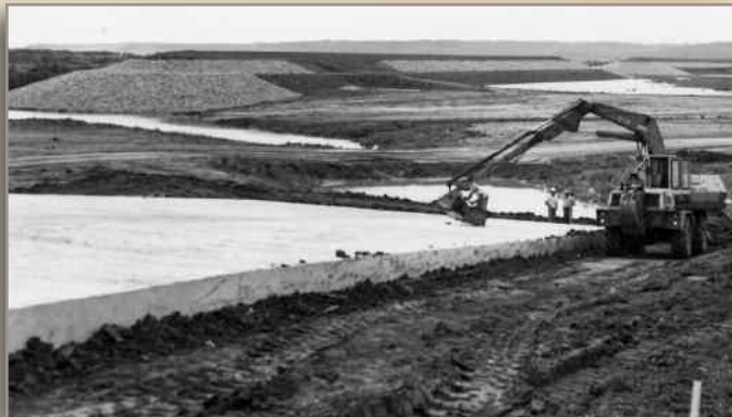
Construction at Clinton Lake, 1978
