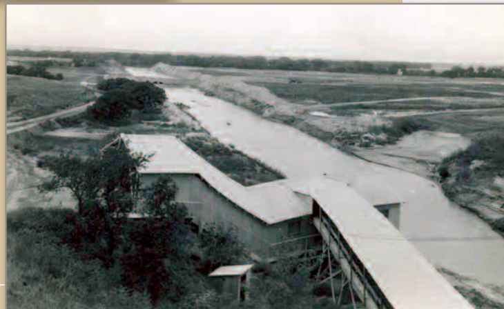
Early construction at Kanopolis Lake
