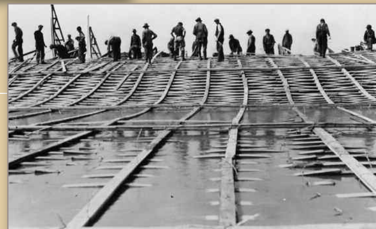
Laying timber for matting, early 1930s
