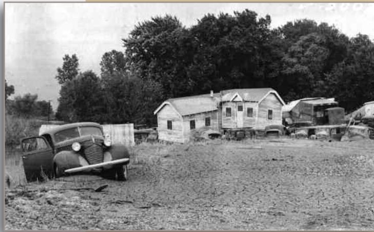
Devastating aftermath of 1951 Flood
