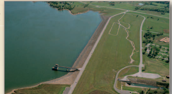
Smithville Dam was authorized in 1965
