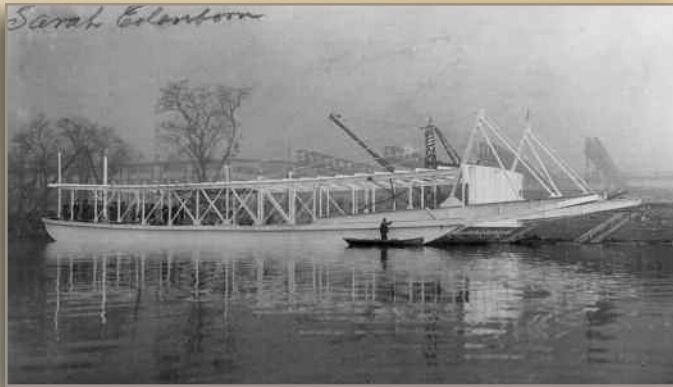
Construction nearly complete on the towboat Sarah Edenboon
