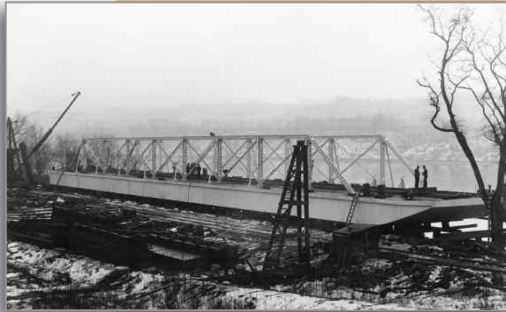
Construction of a Louisiana Railway car barge
