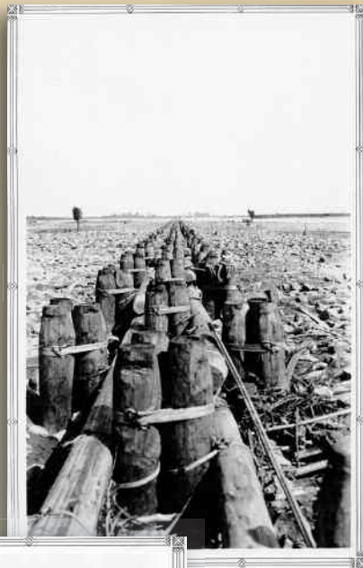
Old wood dike that has fulfilled its purpose, Baltimore Bend
