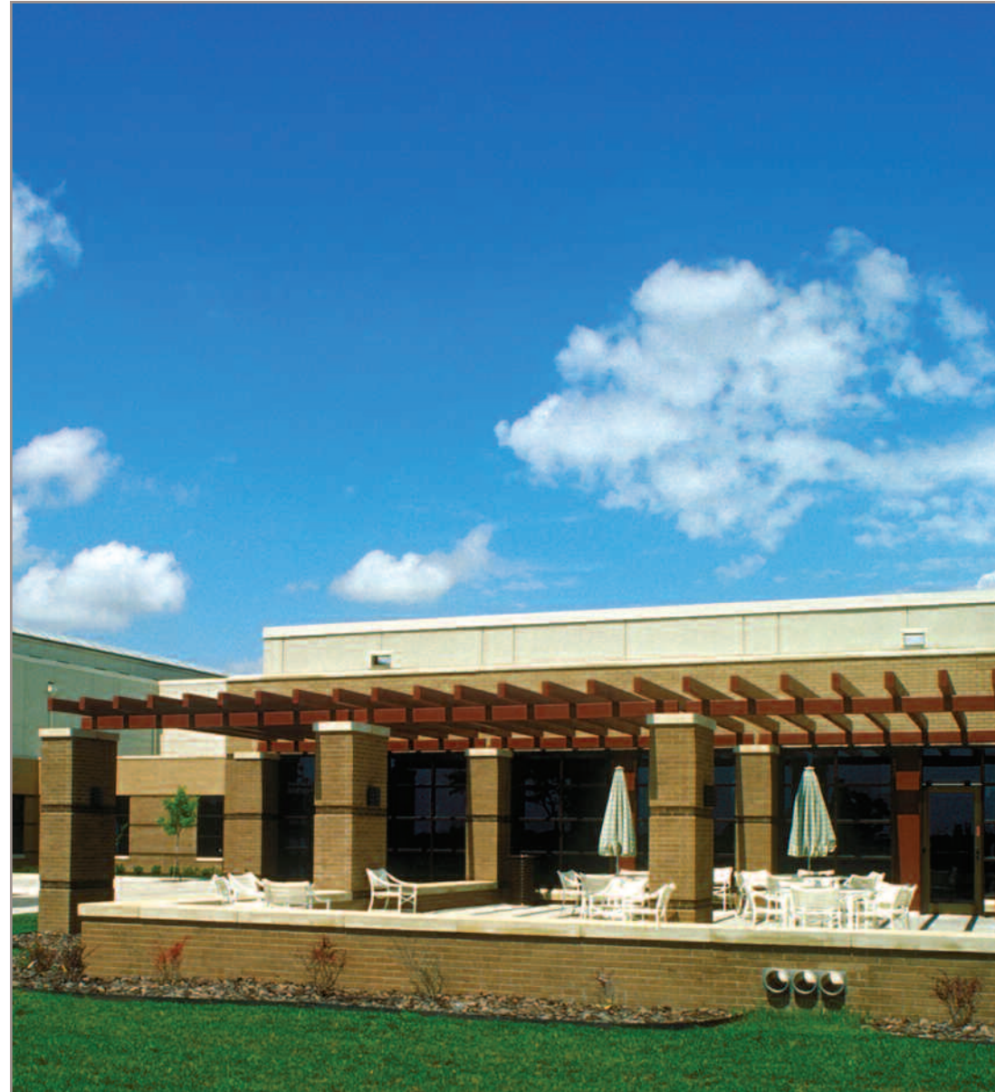
New construction at McConnell Air Force Base
