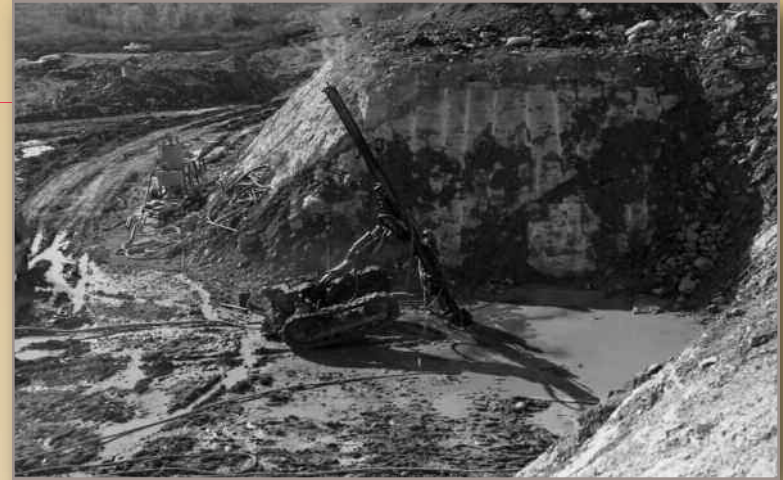
Longview Lake construction began in 1979
