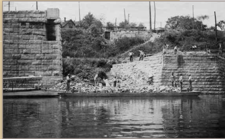
Removing left abutment at Flowline bridge. Barge loaded with 25 yards of stone and ready for timing to Missouri River, August 27, 1913
