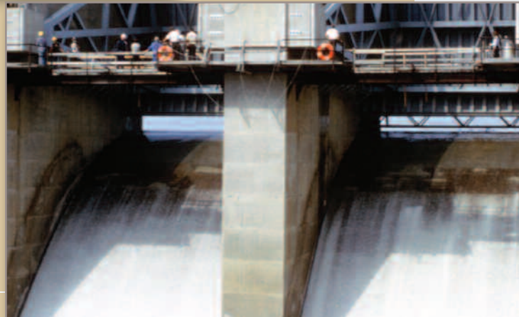
Truman Dam spillway
