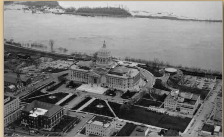
Floodwaters surround Jefferson City, 1973
