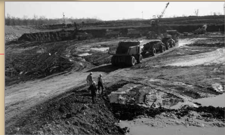
Construction on Stockton Dam, 1964
