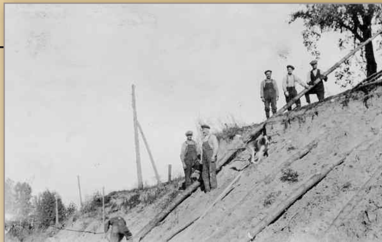
Workers use timbers to help reinforce the bank
