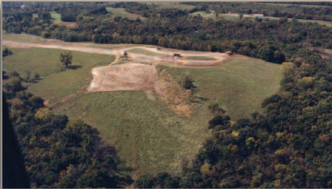
Construction of Blue Springs Lake picnic area, 1985
