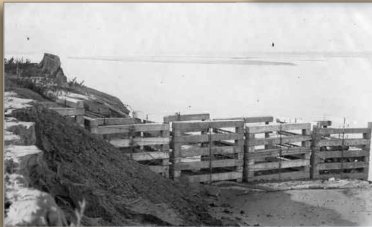
Concrete beam crib dike
