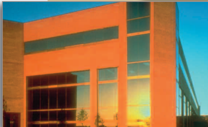
Fort Leonard Wood Engineer School
