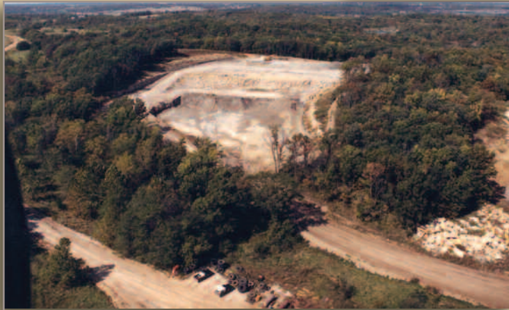
Construction of Blue Springs Lake spillway, 1985
