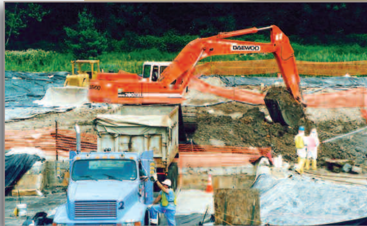
FUSRAP site remediation
