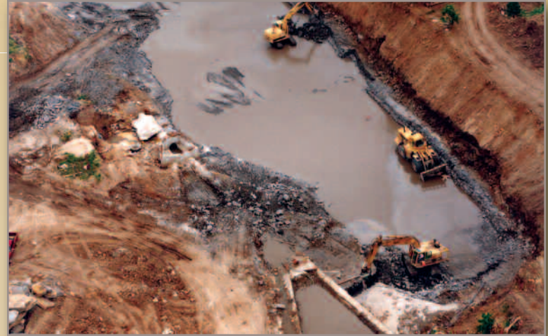
Rebuilding Brush Creek
