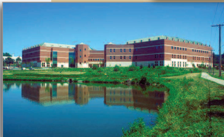
New construction at Fort Leavenworth
