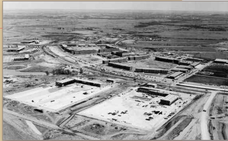
Aerial view of construction activity at Fort Riley, 1969
