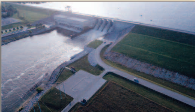
After working through many design challenges, Truman Dam went online with full reliable power December 1, 1999
