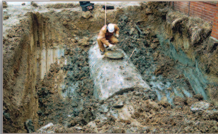
Cleanup of hazardous materials at Weldon Springs Ordnance
