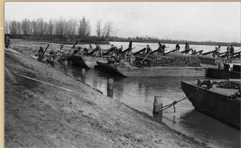
Rock Bluff Bend Revetment, 1933
