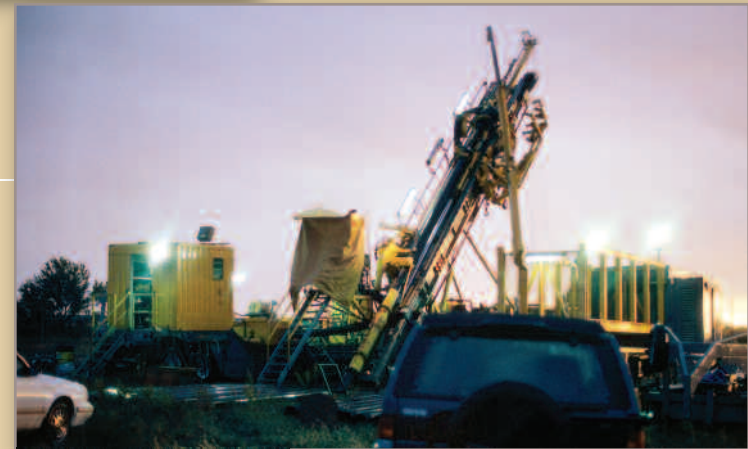
FUDS work at Blaine continues into the night
