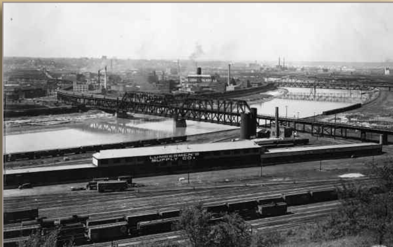
Wide view of truss railroad bridge, Kansas River, 1945
