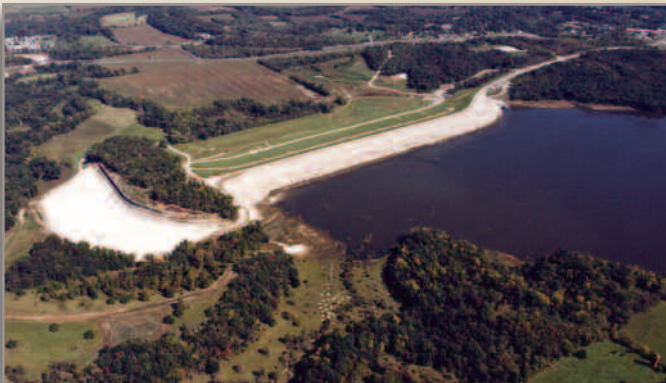
Blue Springs Lake Dam, 1980s
