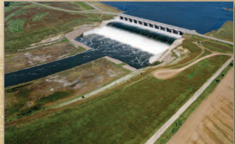
Spillway at Tuttle Creek Dam, completed 1962
