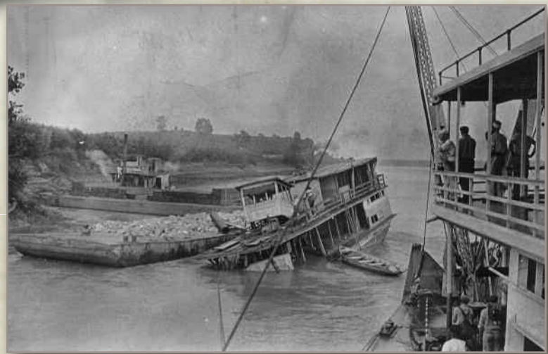
Removing a sunken steamboat
