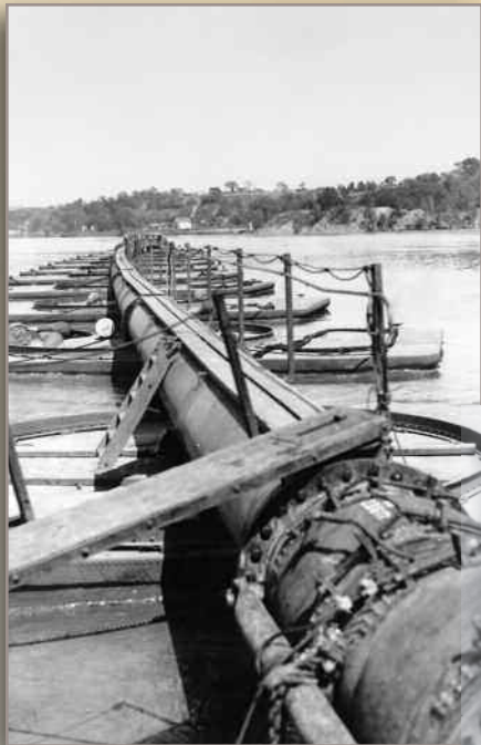
Dredge pipeline floating on water
