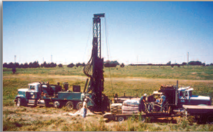
Site cleanup at Blaine Naval Ammunition Depot, Hastings, NE
