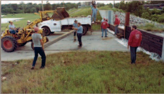
Shoring up the levee on the Marais des Cygnes River during the 1983 flood, Osawatomie, KS
