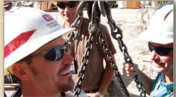
District construction along the Missouri River
