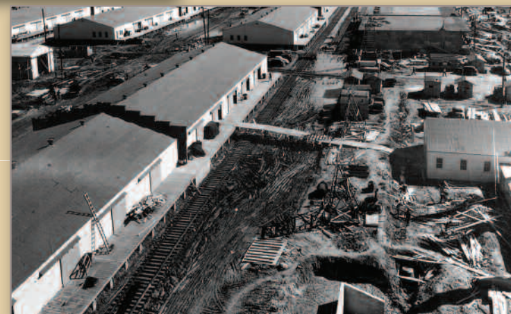
Construction at Fort Leonard Wood, MO, 1941
