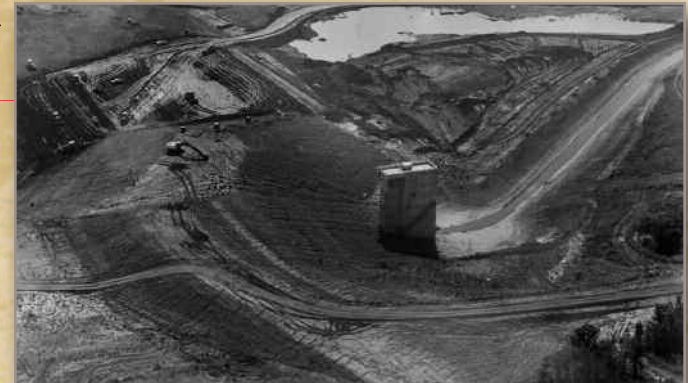
Aerial view of construction at Longview Lake
