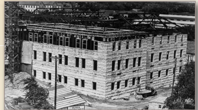
Construction of Patton Hall, Fort Riley, KS (Photo Courtesy: U.S. Cavalry Museum, Fort Riley, KS)
