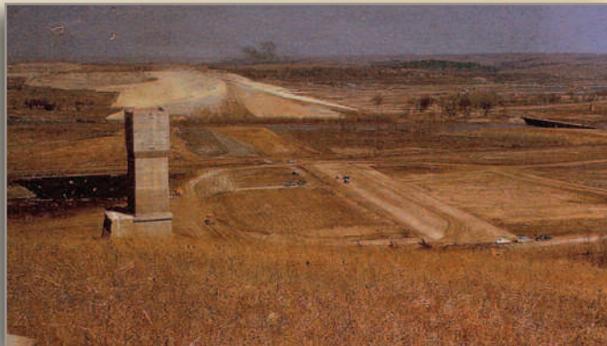
Tuttle Creek Dam under construction
