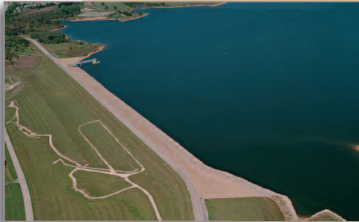
Construction of Smithville Dam was completed in 1977
