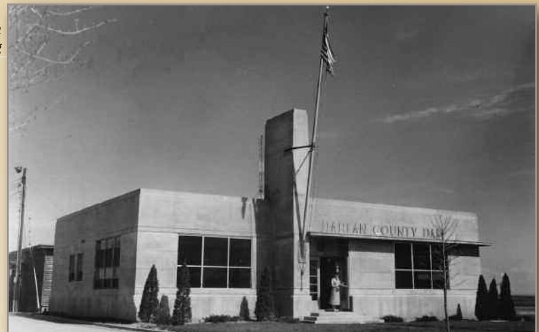
Harlan County Dam administrative building
