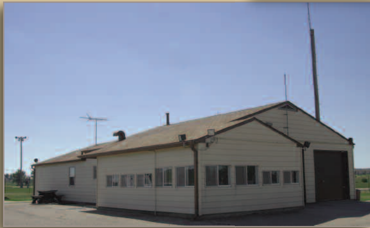
An example of a Minuteman II launch control facility located at Whiteman Air Force Base (U.S. Air Force photo/ Tech Sgt. Samuel A. Park)
