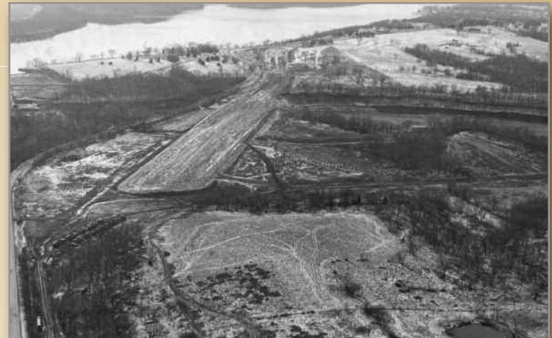
Aerial of road relocation, Blue Springs Lake construction, 1982
