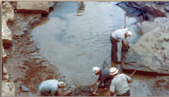
Construction at Melvern Dam, 1973
