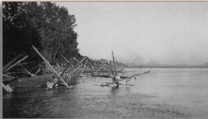
First "Kellner Jetties" built near the foot of Dorman Street. Patented by Mr. Kellner of Atchison, Kansas - October 1925
