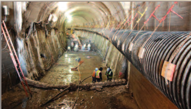
The District is currently rehabilitating the Turkey Creek Tunnel
