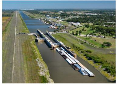
Locks and Dam 27 has twin locks, a main chamber and an auxiliary chamber. The main lock chamber is 1,200 feet long by 110 feet wide. The auxiliary chamber measures 600 feet long by 110 feet wide. Both locks were excavated to bedrock, which serves as the lock chamber floors.
