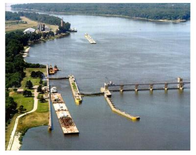
Lock dimensions are 110 feet wide by 600 feet long with additional provisions for an auxiliary lock. Maximum lift is 9.8 feet with an average lift of 6.9 feet. It takes approximately 10 minutes to fill or empty the lock.
