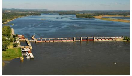
and the upper gate bay of an auxiliary lock. The main lock has the standard 110-foot-wide by 600-foot-long chamber. The average lift is 15 feet. Both the lock and the movable dam are pile-founded structures.
