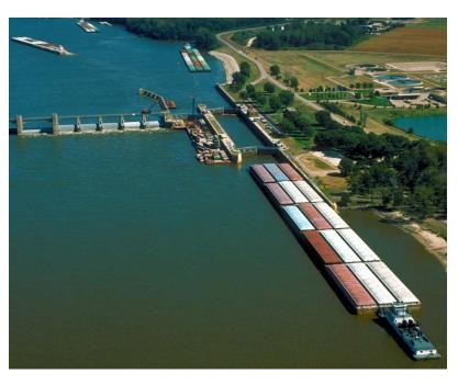
The movable dam has 10 submersible, elliptical Tainter gates (20 feet high by 64 feet long) and three submersible roller gates (20 feet high by 100 feet long). The dam system also includes two earth and sand-filled transitional dikes, and a submersible earth dike. It takes five hours for water to travel from Lock and Dam 20, in Canton, Missouri, to Lock and Dam 21.
