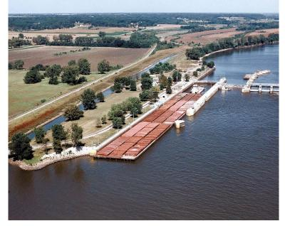
5.3 feet. It takes approximately seven minutes to fill or empty the lock chamber.
