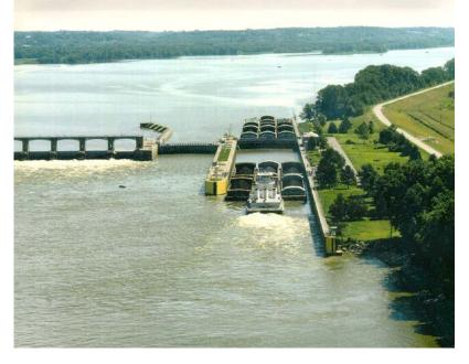
The movable dam has 12 non-submersible Tainter gates (20 feet high and 40 feet long), three submersible Tainter gates of the same dimensions, and four non-submersible roller gates (20 feet high and 80 feet long). The dam system also includes a linear, concrete capped, ogee spillway; and a submersible earth and sand-filled dike. It takes eight hours for water to travel from Lock and Dam 15, in Davenport, Iowa, to Lock and Dam 16.
