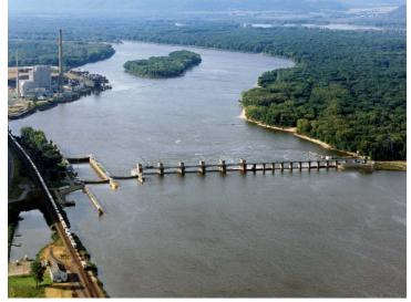
at each end of the lock chamber. There is a partial auxiliary lock consisting of an upstream set of miter gates and short concrete riverwall section. The foundation material consists of piles in sand, gravel and broken clay.
