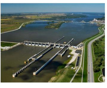
The complex has twin locks. The main lock is 110 by 1,200 feet; the auxiliary lock is 100 feet by 600 feet. The locks are U-shaped and supported on steel H-piles. The maximum lift is 24 feet.
