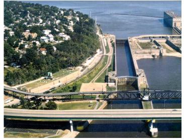
gates, 53-feet 2-inches high. The lower lock gates are conventional miter gates, while the upper service gate is a submergible lift gate. Upstream from the upper service gate is a submergible vertical-lift guard gate which serves as an emergency gate in case of failure of the service gate. This gate also serves as a bridge in the roadway to the old dry dock, old lock, powerhouse and dam.
