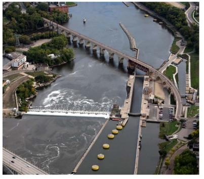
descending bank the Corps has a short non-overflow concrete dam between the Lock and the bank.
