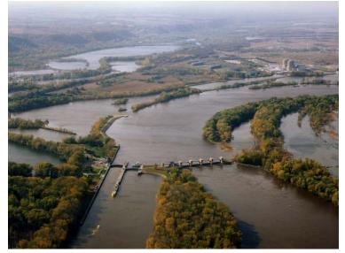
miter gates at each end of the lock chamber. There is a partial auxiliary lock consisting of an upstream set of miter gates and a short concrete riverwall section. The lock foundations are set in sand, silt and clay.
