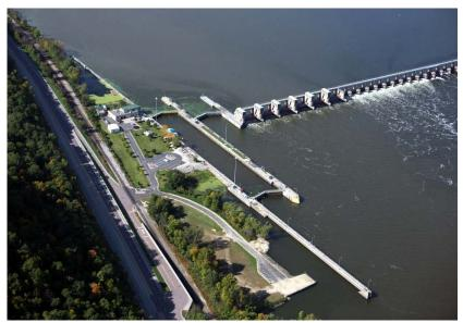
tailwater elevation of 651.0 feet, and a vertical lift of 9.0 feet. There are miter gates at each end of the lock chamber and a partial auxiliary lock consisting of an upstream set of miter gates and short concrete riverwall section. The foundation consists of piles in sand and gravel.
