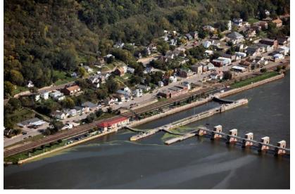
tailwater elevation of 660.0 feet, and a vertical lift of 7.0 feet. There are miter gates at each end of the lock chamber. There is a partial auxiliary lock consisting of an upstream set of miter gates and short concrete riverwall section. The foundation is piles in sand and gravel.
