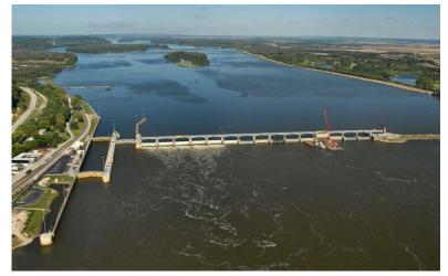
atop sand and gravel, Lock 24 is founded on durable shale. Because of the presence of a firm foundation material, the lock chamber is not floored and no lateral struts were provided to stabilize the intermediate and river walls.
