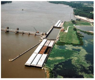
water depth of eight feet at the upper sill and seven feet at the lower sill. The main lock's maximum lift is 11 feet with an average lift of 9.8 feet. It takes approximately eight minutes to fill or empty the main lock.
