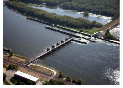
the lock chamber. A partial auxiliary lock consists of an upstream set of miter gates and a short concrete riverwall.
