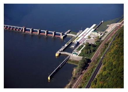
partial auxiliary lock consisting of an upstream set of miter gates and short concrete riverwall section.
