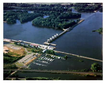
The movable dam consists of an 893-foot-long concrete structure with five roller gates (20 feet high by 80 feet long) and 10 non-submersible Tainter gates (15 feet high by 35 feet long), and is located adjacent to the auxiliary lock. Completing the dam system is an earthen embankment approximately 1,600 feet long, located between the movable dam and high ground on the Minnesota side of the river, with a 1,000-foot-long concrete overflow spillway.
