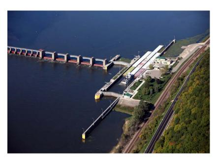
partial auxiliary lock consisting of an upstream set of miter gates and short concrete riverwall section.
