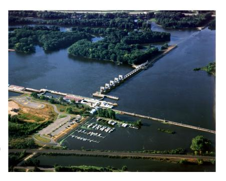
The movable dam consists of an 893-foot-long concrete structure with five roller gates (20 feet high by 80 feet long) and 10 non-submersible Tainter gates (15 feet high by 35 feet long), and is located adjacent to the auxiliary lock. Completing the dam system is an earthen embankment approximately 1,600 feet long, located between the movable dam and high ground on the Minnesota side of the river, with a 1,000-foot-long concrete overflow spillway.
