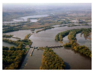
miter gates at each end of the lock chamber. There is a partial auxiliary lock consisting of an upstream set of miter gates and a short concrete riverwall section. The lock foundations are set in sand, silt and clay.
