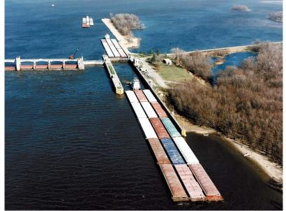
Lock dimensions are 110 by 600 feet with additional provisions for an auxiliary lock. The maximum lift is 11 feet with an average lift of 8.6 feet. It takes approximately 10 minutes to fill or empty the lock chamber.
