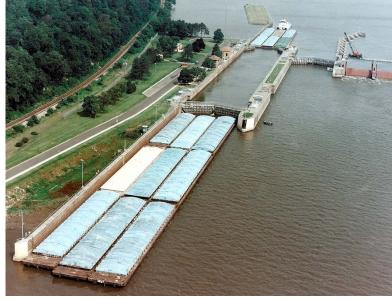
Lock dimensions are 110 feet wide by 600 feet long with additional provisions for an auxiliary lock. The maximum lift is 11 feet with an average lift of 9.4 feet. It takes approximately seven minutes to fill or empty the lock chamber.
