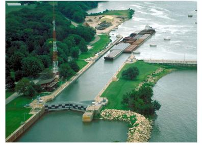
concrete in 1982. The 52-foot-long ice chute section of the dam includes a 52-foot-long inoperable Tainter gate. The lock is the standard 600 feet long by 110 feet wide. The maximum lift is 18.5 feet with an average lift of 17 feet. It takes approximately 12 minutes to fill the lock chamber; nine minutes to empty.
