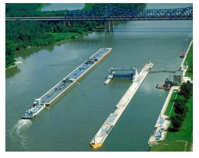
From 1987-1990, a major rehabilitation changed the physical components of the dam and operating procedures by replacing 26 of the original 134 wickets with a single 84-foot long submersible Tainter gate adjacent to the lock wall.
