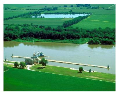
feet wide by 14.92 feet high, with a .25-foot gap between wickets. From 1987-1991, a major rehabilitation changed the physical components of the dam and operating procedures by replacing 26 of the original 135 wickets with a single 84-foot long submersible Tainter gate adjacent to the lock wall.
