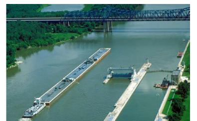
From 1987-1990, a major rehabilitation changed the physical components of the dam and operating procedures by replacing 26 of the original 134 wickets with a single 84-foot long submersible Tainter gate adjacent to the lock wall.
