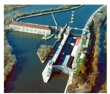
support structures to the Corps in the early 1980s for the roughly forty-five foot high embankment, controlling works, powerhouse substructures, and all pool retention structures. The Corps controls the lock; however, has no ownership of the controlling works.
