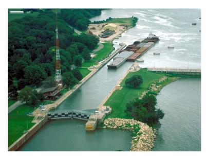
concrete in 1982. The 52-foot-long ice chute section of the dam includes a 52-foot-long inoperable Tainter gate. The lock is the standard 600 feet long by 110 feet wide. The maximum lift is 18.5 feet with an average lift of 17 feet. It takes approximately 12 minutes to fill the lock chamber; nine minutes to empty.
