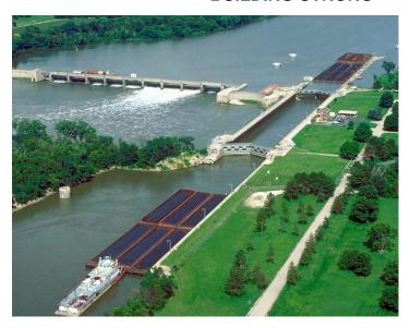
The dam consists of an arch dam section, a fixed spillway section, nine Tainter gates (60 feet wide by 17 feet high), 18 plugged headgates, and a 500-foot-long earthfill section with steel sheet pile cut-off wall connecting the headgate section to the Illinois and Michigan Canal embankment.
