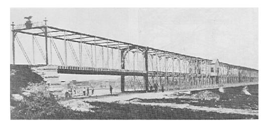
In 1872, another bridge was built to replace the wooden one. However, the location was changed. This bridge was built on the same site as the present day Government Bridge. It consisted of a single rail line above a wagon path. The train track was designed to be on top because the smoke and noise frightened horses when trains ran under them.
