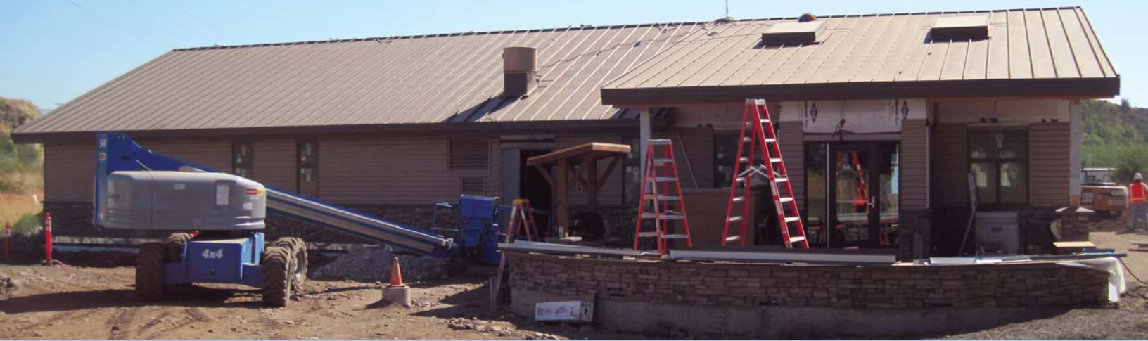
U.S. Army Corps of Engineers photos
