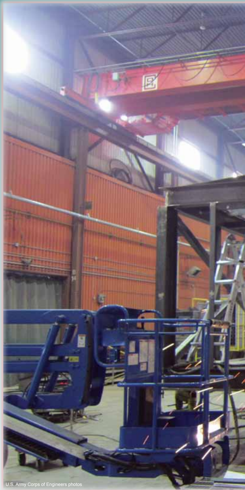
U.S. Army Corps of Engineers photos
