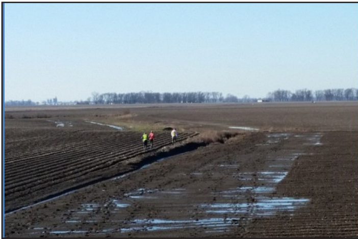
Vidalia Area Office staff working with Louisiana ARNG to check boil.
