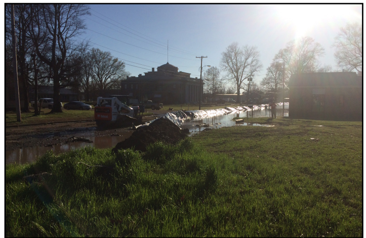
Corps Field Office provided the visqueen supplies used in the Coldwater flood fight. (Photos by Joseph Matthews)
