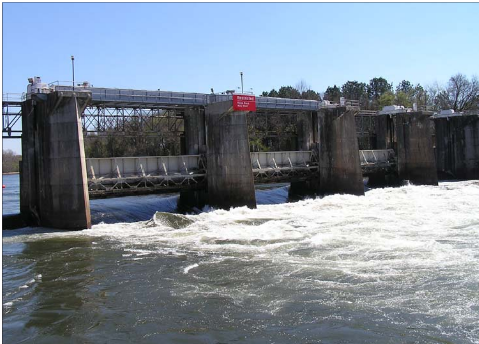
New Savannah Bluff Lock and Dam is shown during the pulse release. When flows in the Savannah exceed 16,000 cubic feet per second, the gates of the structure are raised, which scientists hypothesized would encourage fish passage through the structure.
