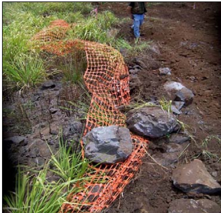
Photo 1: July 25, 2006 – Boulders rolled onto fencing
