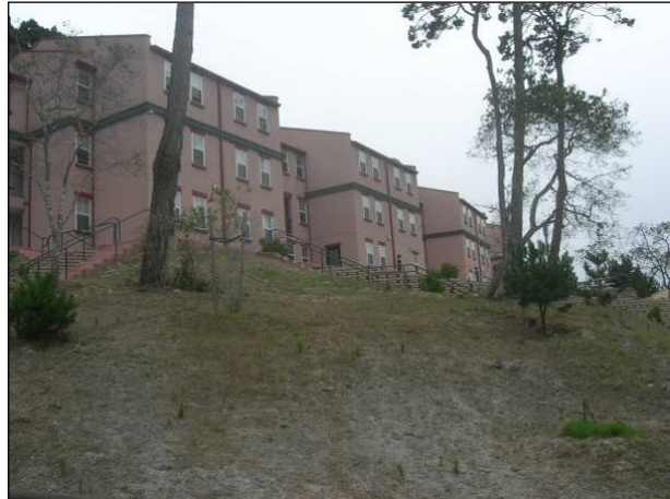
Photo 6. Newer Barracks Buildings at the POM
