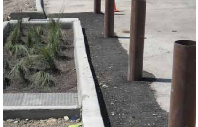
This LID modular wetland stormwater control feature is at Fort Hood, Tex. Photo courtesy of ERDC.
