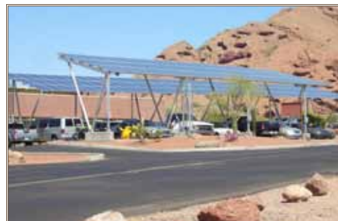
In 2012 the Arizona ARNG opened up a pilot program solar parking lot. The 20-car site provides covered parking for vehicles, and the top of the parking structure is covered in solar panels. The solar array has a capacity of 44.5 kW DC peak, expected to produce 75,000kWh/Year.
