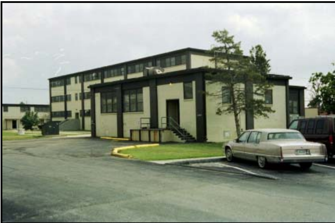
Figure 4.1.23 105-man hammerhead barracks, Bldg. 2381 (1953), Ft. Knox, view SE (RCG&A).
