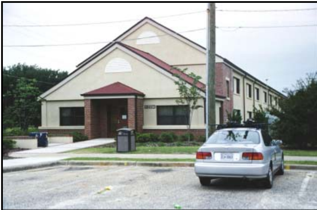
Figure 4.2.15 Renovated two-story, hammerhead BOQ, Bldg. 1-2334 (1953), Ft. Bragg, view NW (RCG&A).
