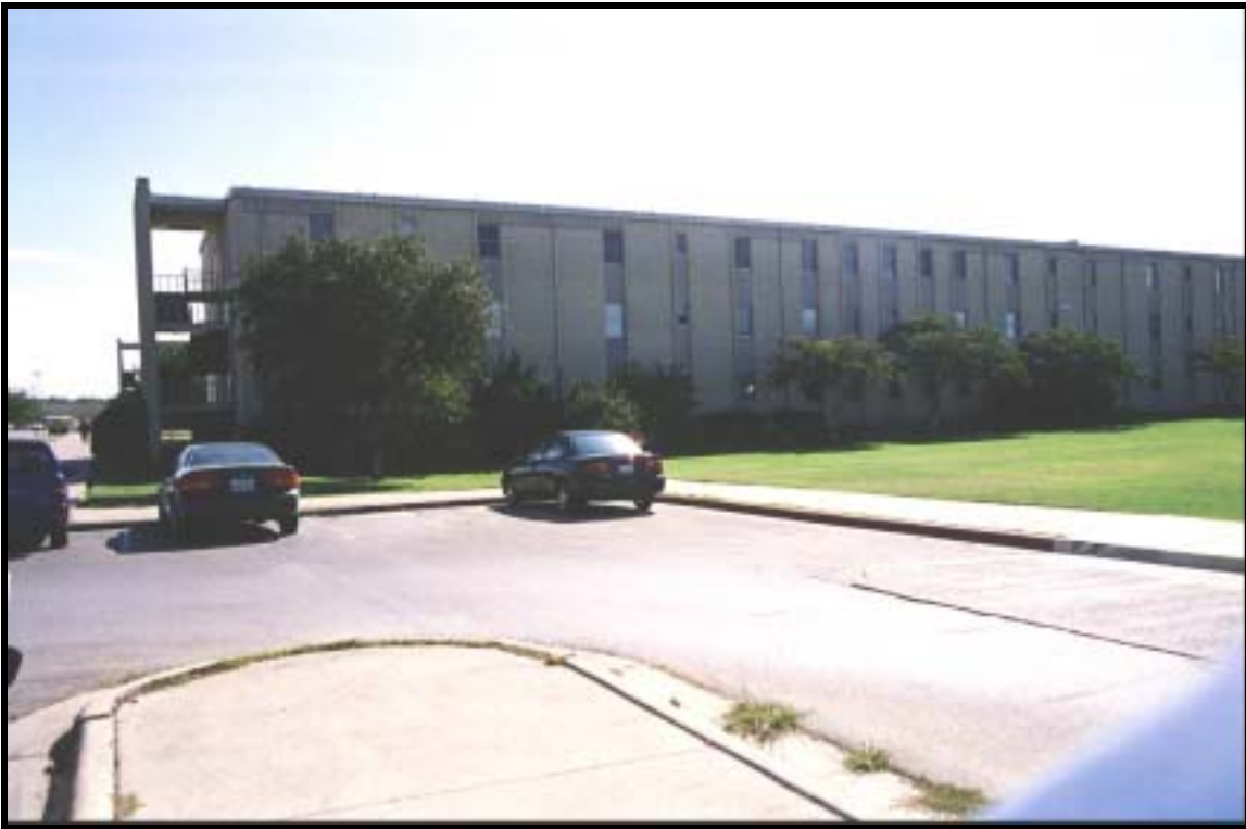
Figure 4.1.93 A-style barracks, Bldg. 41002 (1972), Ft. Hood, view SW (RCG&A).
