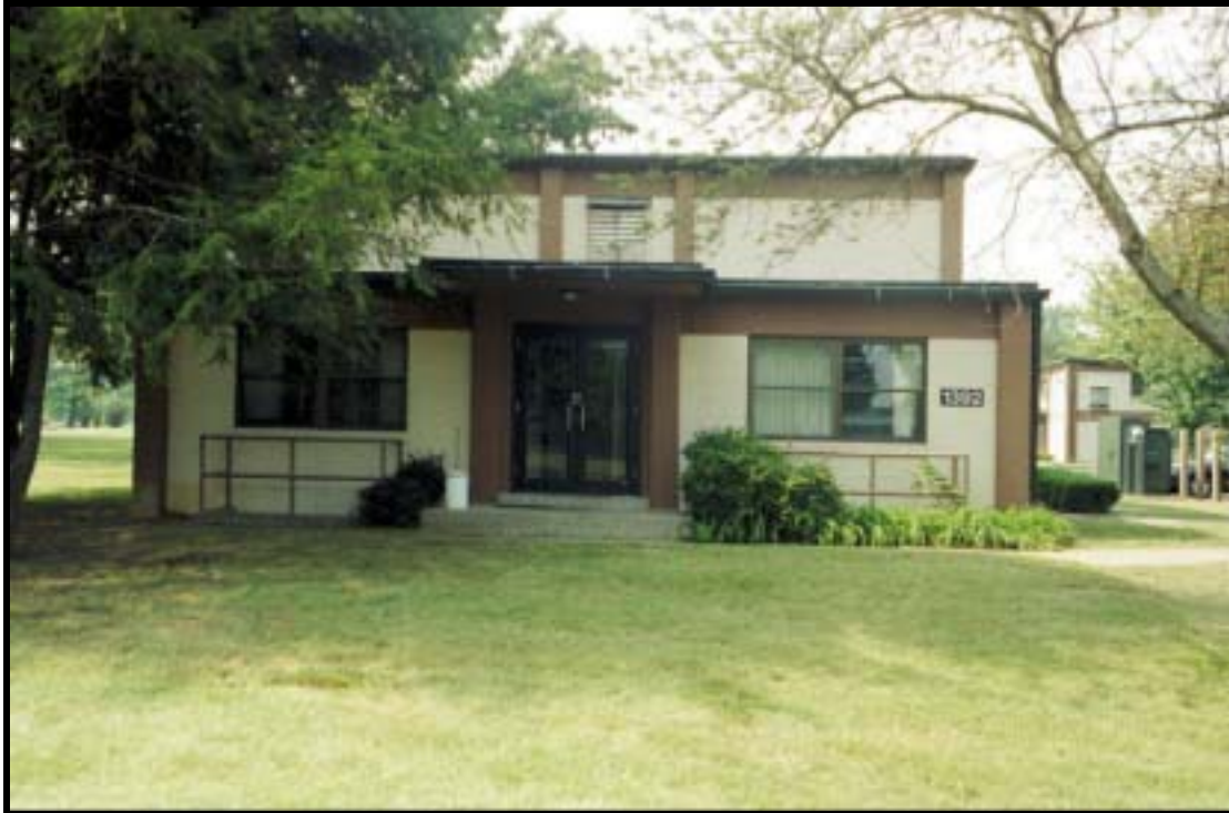
Figure 4.2.12 Two-story, hammerhead BOQ, Bldg. 1392 (1954), Ft. Knox, view W (RCG&A).
