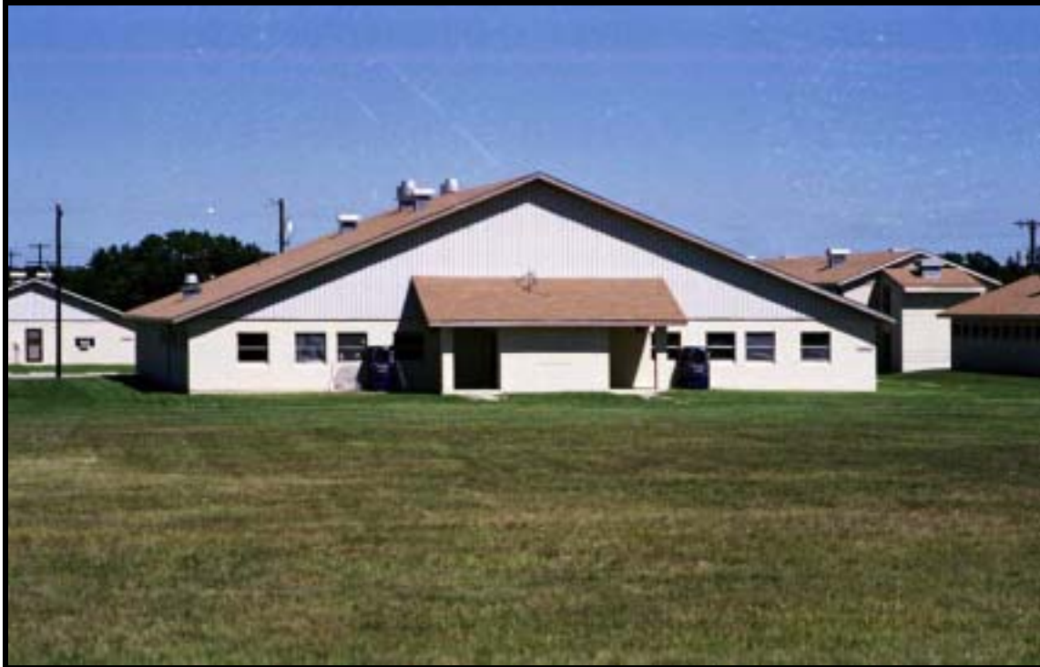
Figure 4.1.125 Army Reserve Annual Training dining facility, Bldg. 56447 (1979), North Ft. Hood, view NE (RCG&A).
