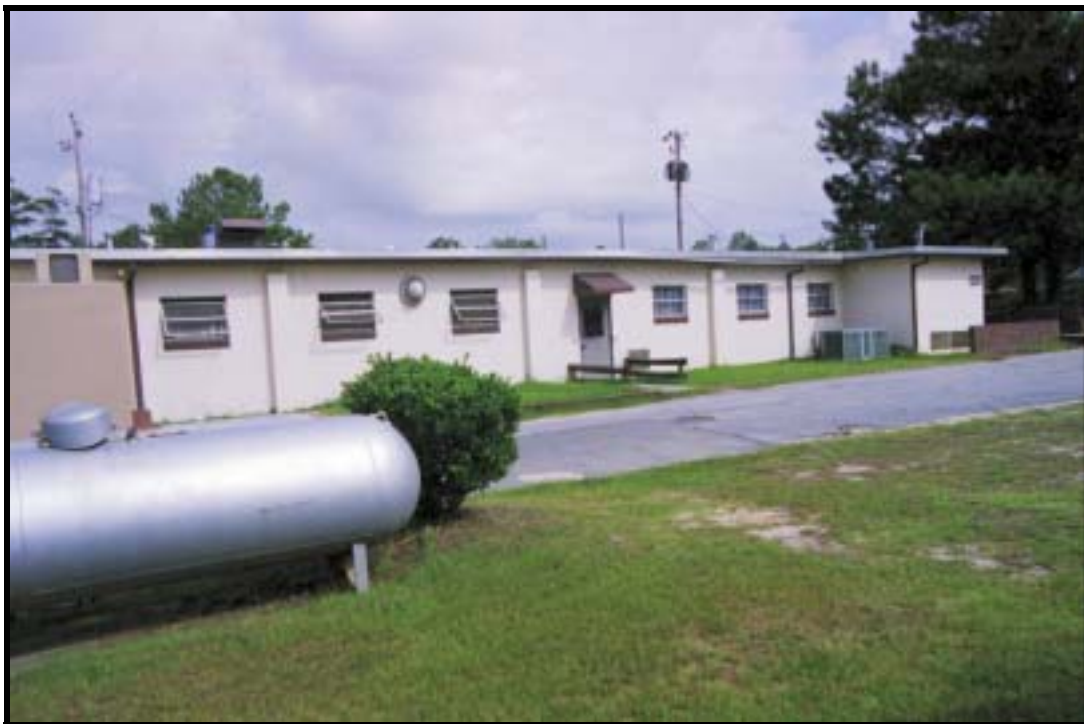
Figure 4.1.177 Semi-permanent dining facility, Bldg. 4702 (1967), Ft. Benning, view W (RCG&A).
