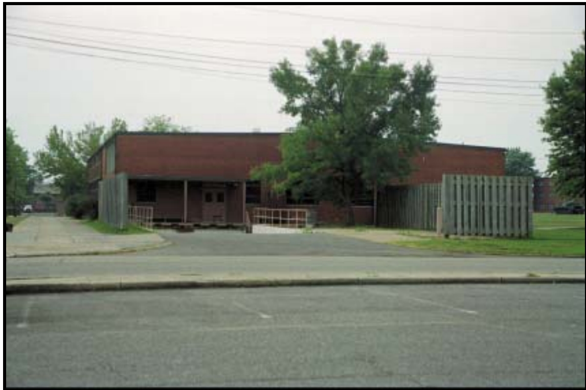
Figure 4.1.81 Rolling Pin dining facility, Bldg. 5917 (1969), Ft. Knox, view S (RCG&A).
