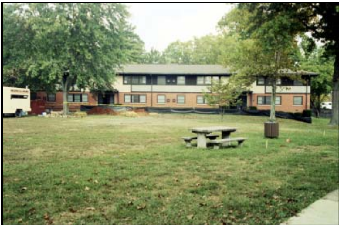
Figure 4.2.27 Two-story, apartment type women's BOQ, Bldg. 857 (1959), Ft. Knox, view N (RCG&A).
