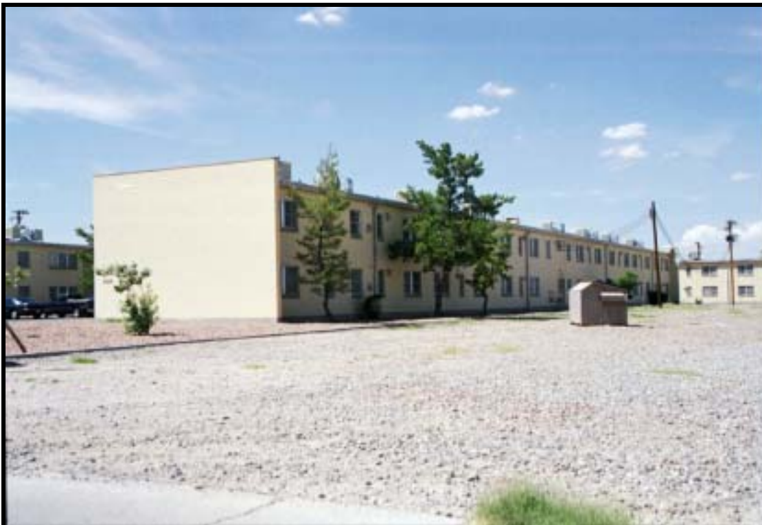
Figure 4.2.33 Two-story, apartment type BOQ, Bldg. 5045 (1962), Ft. Bliss, view NW (RCG&A).
