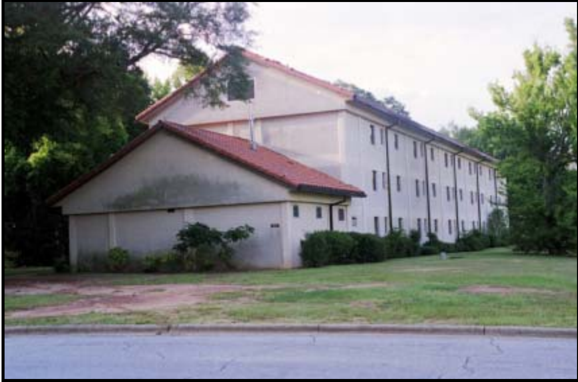
Figure 4.2.22 Renovated three-story, hammerhead UOQ, Bldg. 975 (1956), Ft. Benning, view SE (RCG&A).
