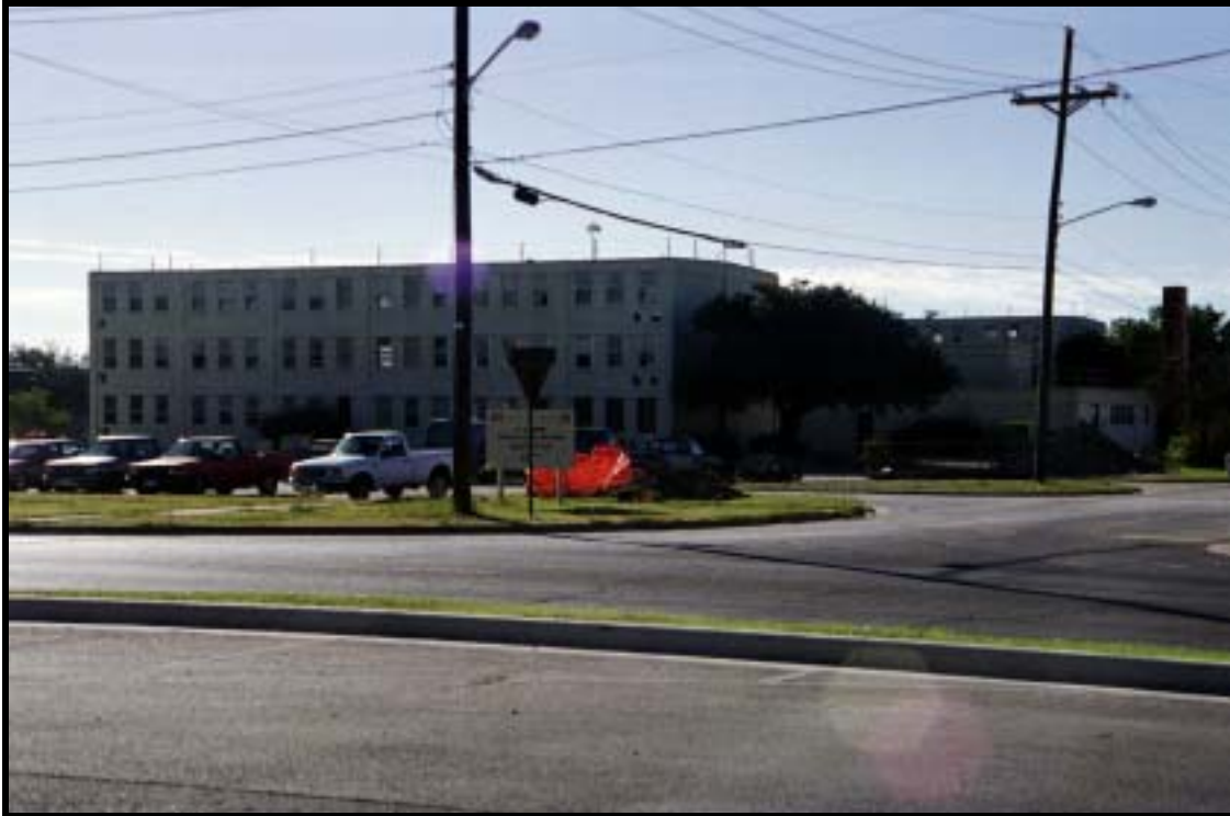
Figure 4.1.61 Renovating H-style, two-company barracks, Bldg. 9211 (1958), Ft. Hood, view SE (RCG&A).
