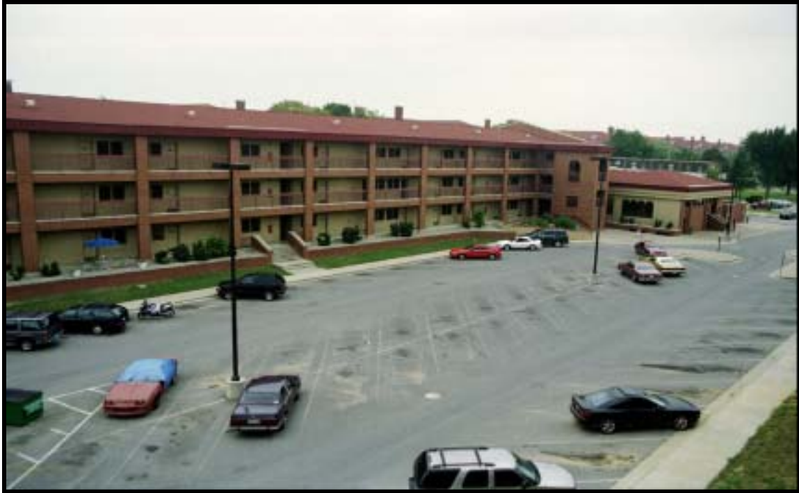
Figure 3.1.39 Totally renovated hammerhead barracks, Bldg. 1482 (1953), Ft. Knox, view SW (RCG&A).
