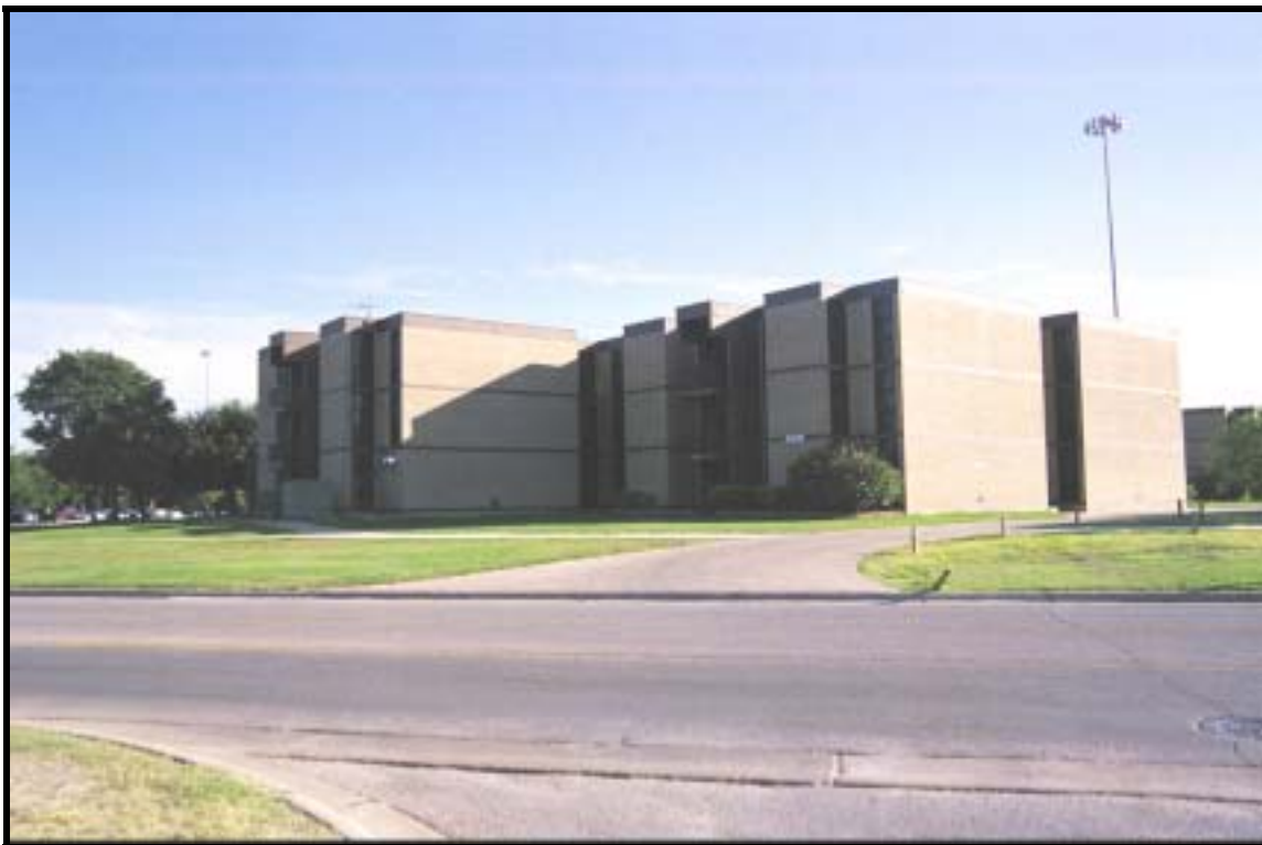
Figure 4.1.104 LBC&W barracks, Bldg. 39039 (1978), Ft. Hood, view S (RCG&A).
