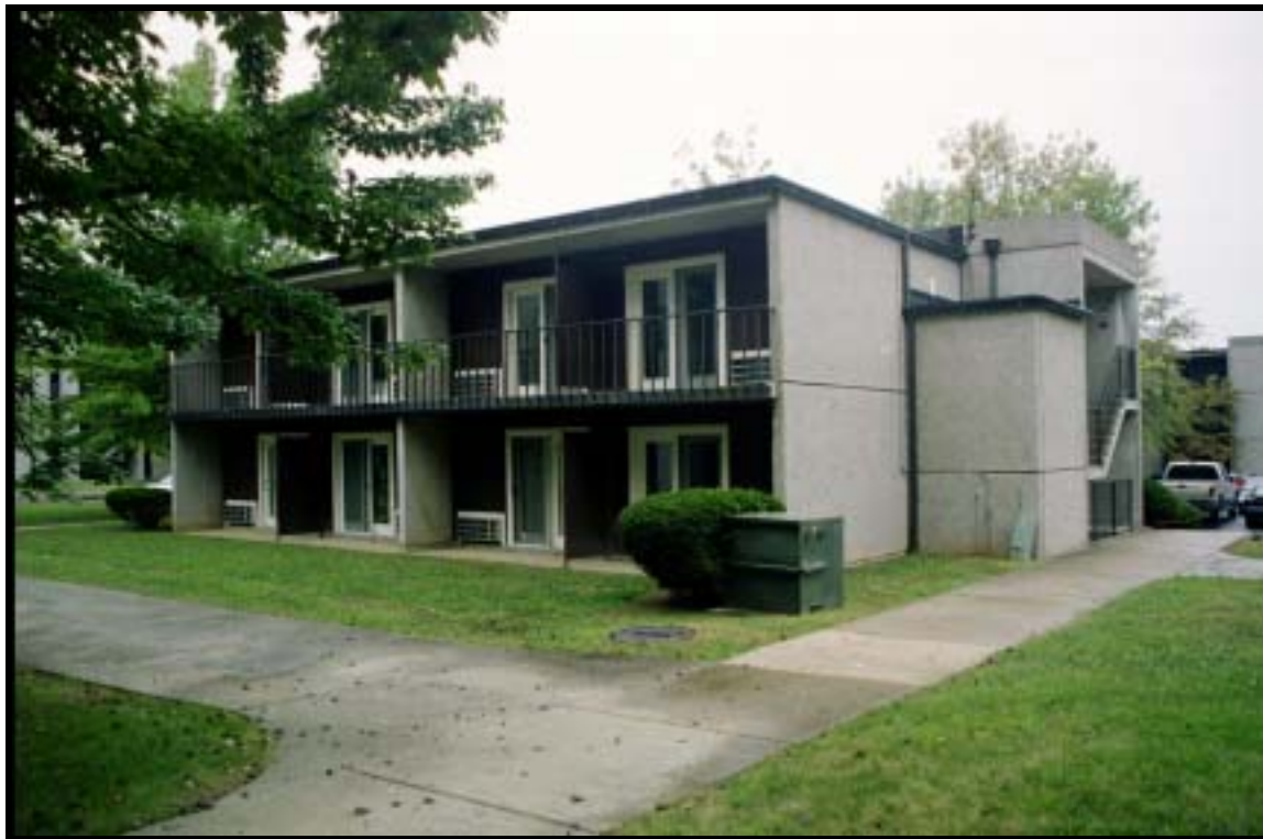
Figure 3.24 Apartment-type BOQ, Bldg. 2604 (1974), Ft. Knox, view NW (RCG&A).
