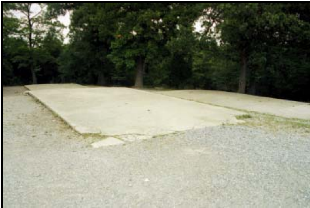
Figure 4.1.228 Tent Pad, Ft. Knox, view NE (RCG&A).
