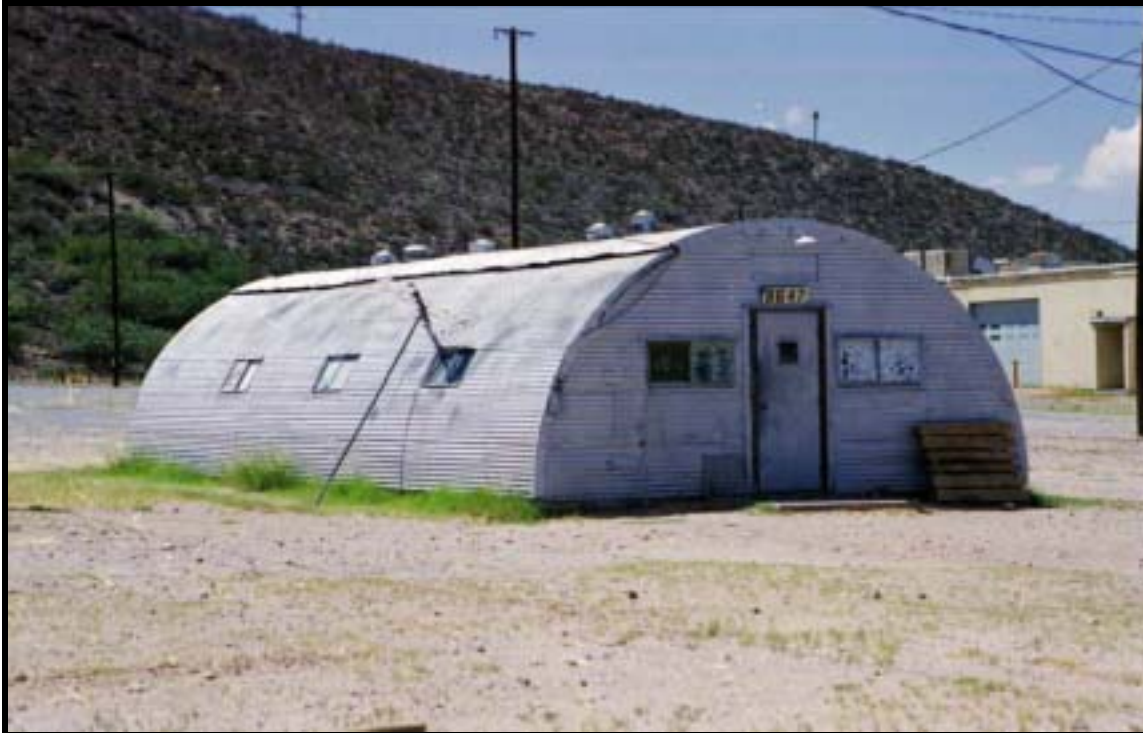
Figure 4.1.199 Quonset hut, Bldg. 8647 (1958), Oro Grande Range, Ft. Bliss, view W (RCG&A).
