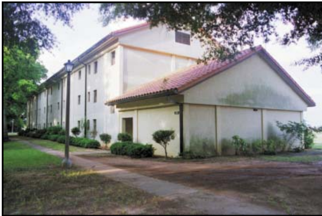
Figure 4.2.21 Renovated three-story, hammerhead UOQ, Bldg. 975 (1956), Ft. Benning, view S (RCG&A).
