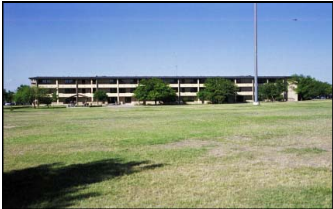
Figure 4.1.83 Renovated Rolling Pin, two-company barracks, Bldg. 37006 (1968), Ft. Hood, view N (RCG&A).
