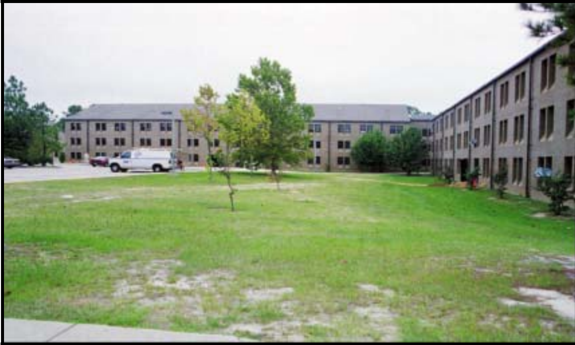
Figure 4.1.151 Double Quadrangle barracks, Bldg. E-4824 (1988), Ft. Bragg, view N (RCG&A).
