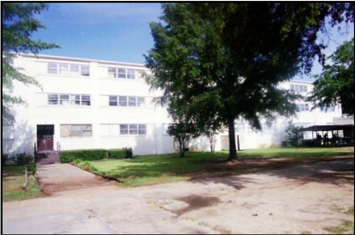
Figure 4.1.13 225-man hammerhead barracks, Bldg. 2839 (1954), Ft. Benning, view W (RCG&A).
