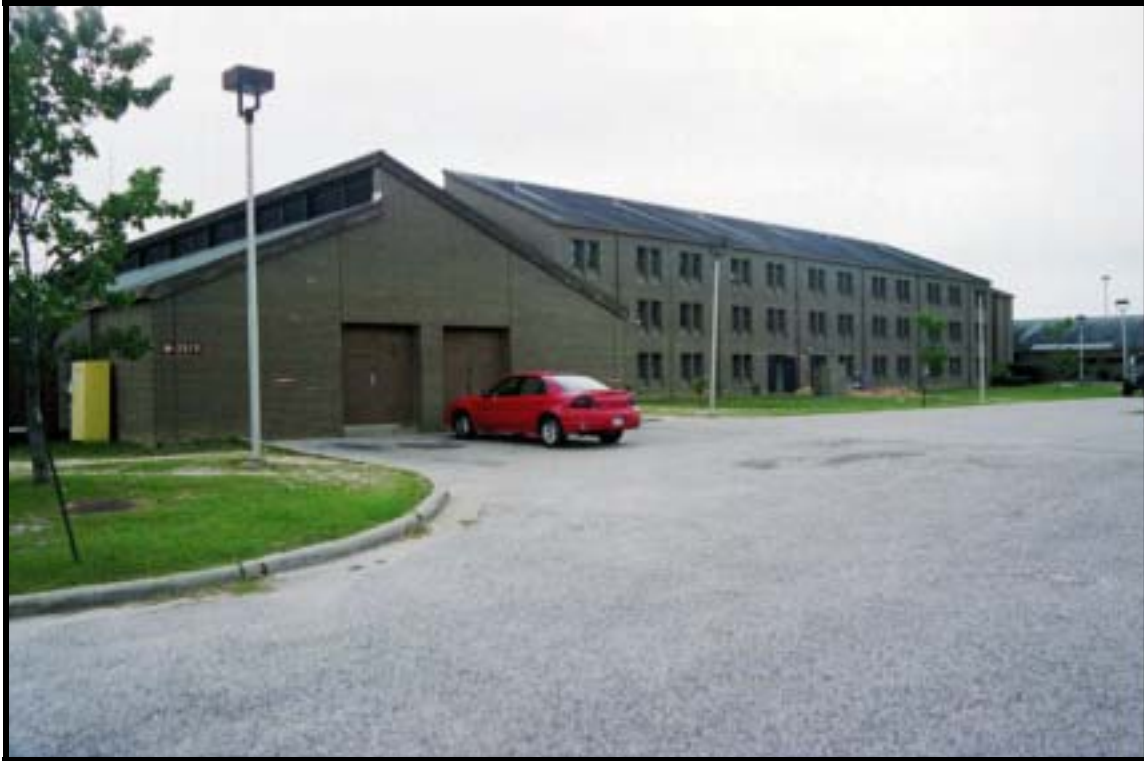
Figure 4.1.59 Quadrangle barracks, Bldg. M-3519 (1987), Ft. Bragg, view NE (RCG&A).
