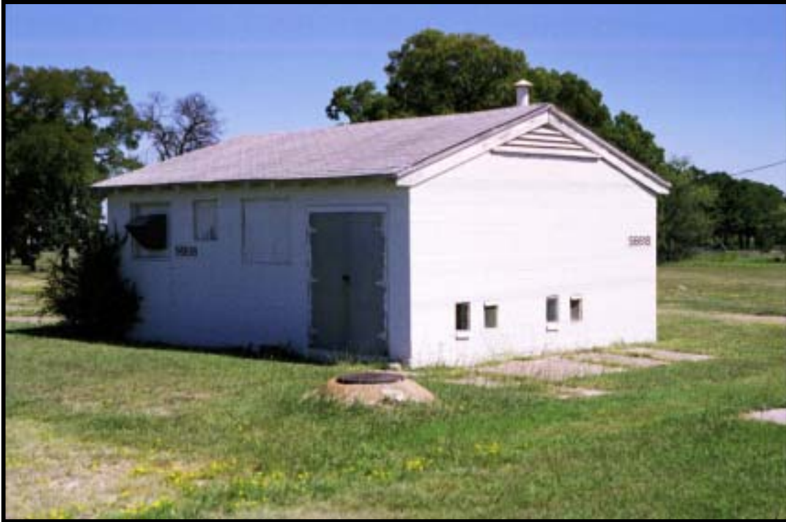
Figure 4.1.214 C-hut dining facility, Bldg. 56618 (1951), North Ft. Hood, view E (RCG&A).
