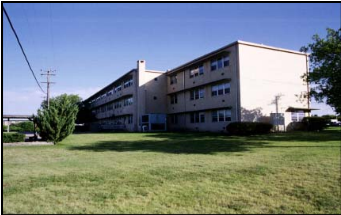
Figure 4.1.75 Rolling Pin, two-company barracks, Bldg. 36001 (1968), Ft. Hood, view SE (RCG&A).
