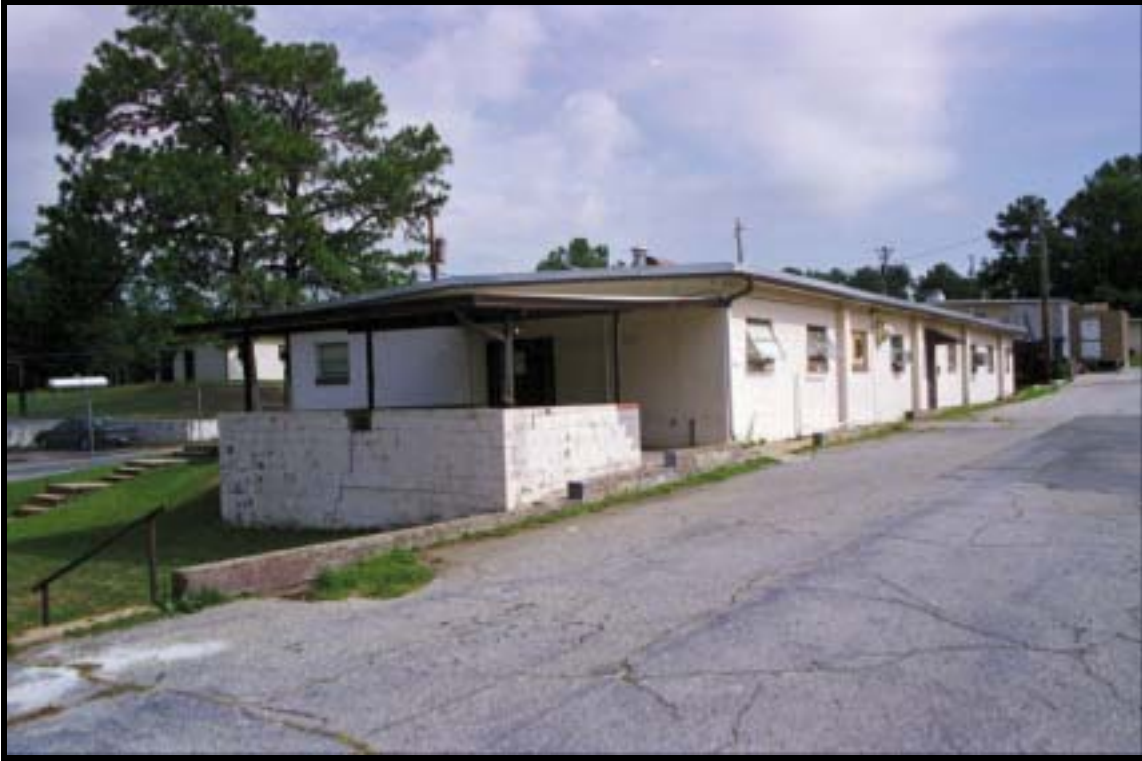
Figure 4.1.178 Semi-permanent dayroom, Bldg. 4703 (1967), Ft. Benning, view W (RCG&A).
