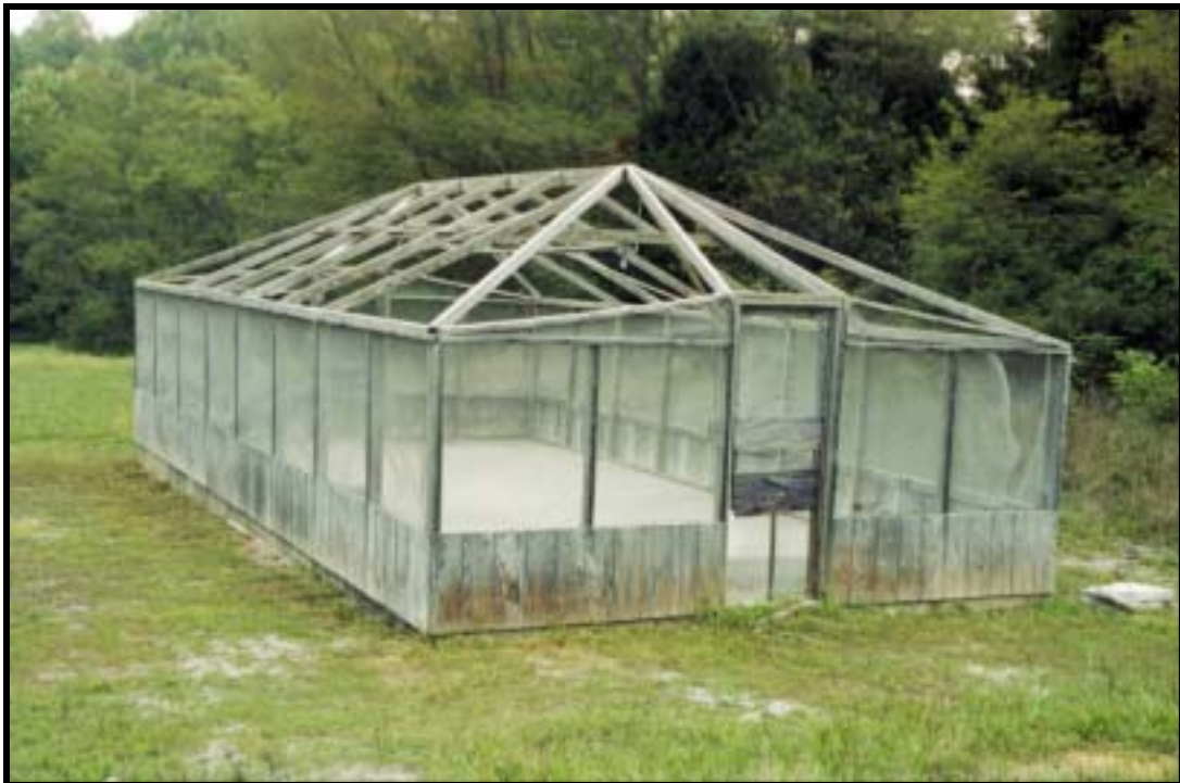
Figure 4.1.230 Tent Pad with wood tent frame, Ft. Knox, view NE (RCG&A).
