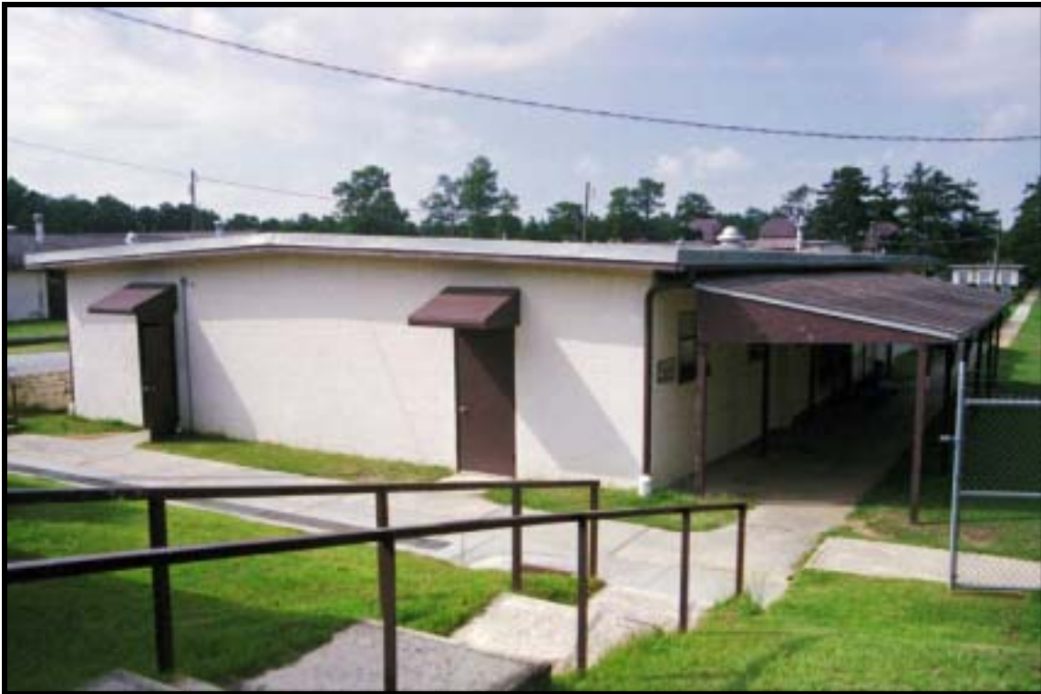
Figure 4.1.179 Semi-permanent dayroom, Bldg. 4703 (1967), Ft. Benning, view E (RCG&A).
