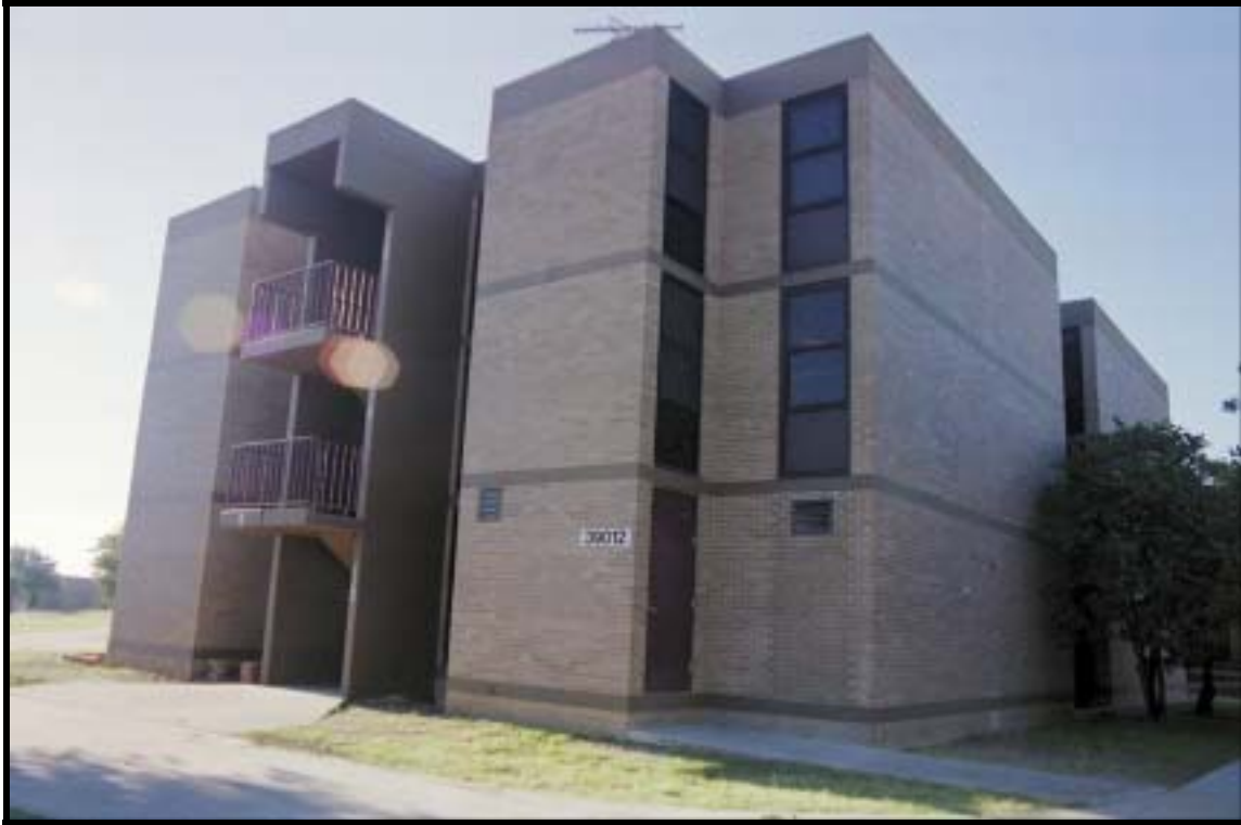
Figure 4.1.103 LBC&W barracks, Bldg. 39012 (1977), Ft. Hood, view SE (RCG&A).
