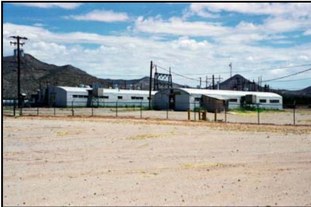
Figure 4.1.208 Mobilization dining facilities, Bldg. 8615, 8614, Oro Grande Range, Ft. Bliss, view E (RCG&A).
