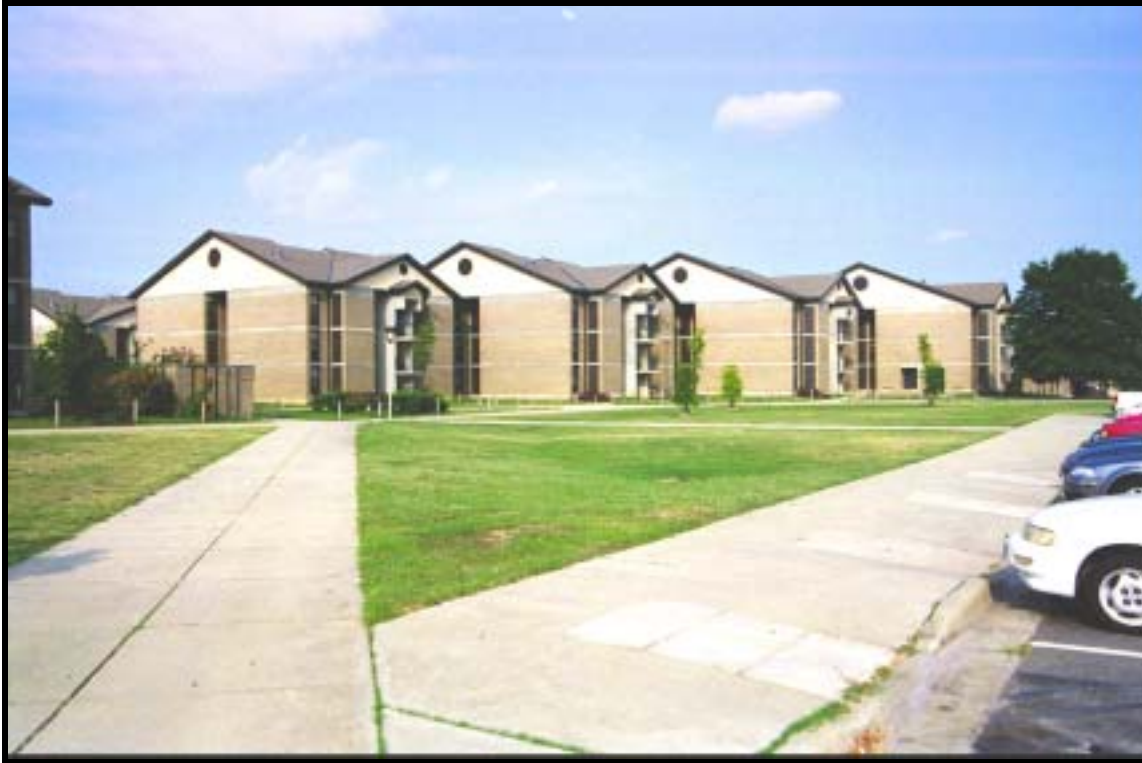
Figure 4.1.105 LBC&W barracks, Bldg. H-4817 (1980), Ft. Bragg, view NE (RCG&A).
