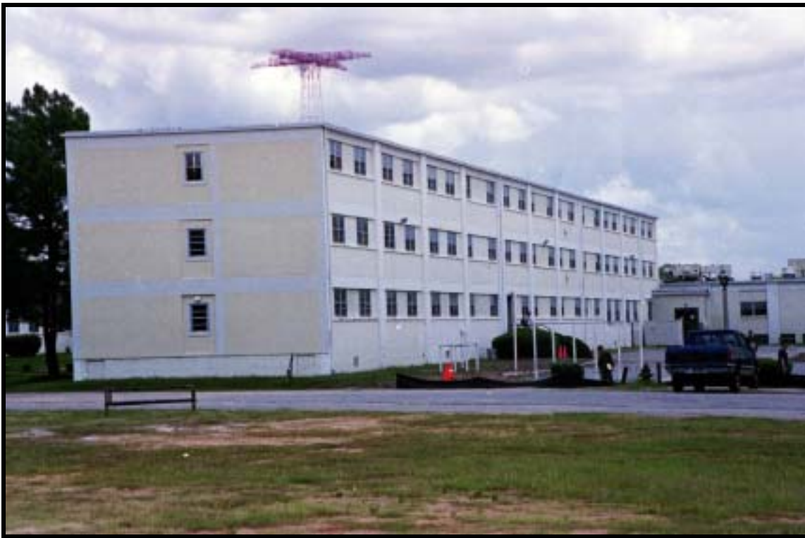
Figure 4.1.28 Double hammerhead barracks, Bldg. 2753 A (1954), Ft. Benning, view NE (RCG&A).
