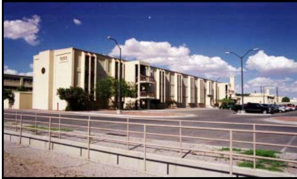
Figure 4.1.33 Extensive renovations to hammerhead barracks include new windows, window treatments, exterior materials, and exterior stairs, Bldg. 1003 (1956), Ft. Bliss, view NE (RCG&A).
