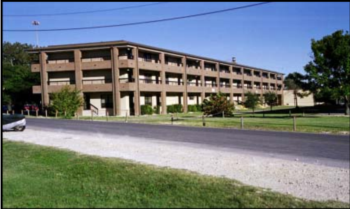
Figure 4.1.37 Rebuilt hammerhead barracks includes balconies and new exterior materials, Bldg. 10020 (1953), Ft. Hood, view NW (RCG&A).
