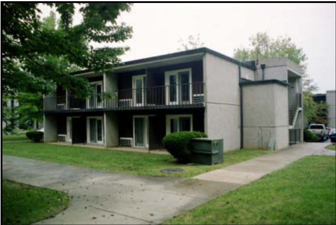
Figure 4.2.47 Apartment-type BOQ, Bldg. 2604 (1974), Ft. Knox, view NW (RCG&A).
