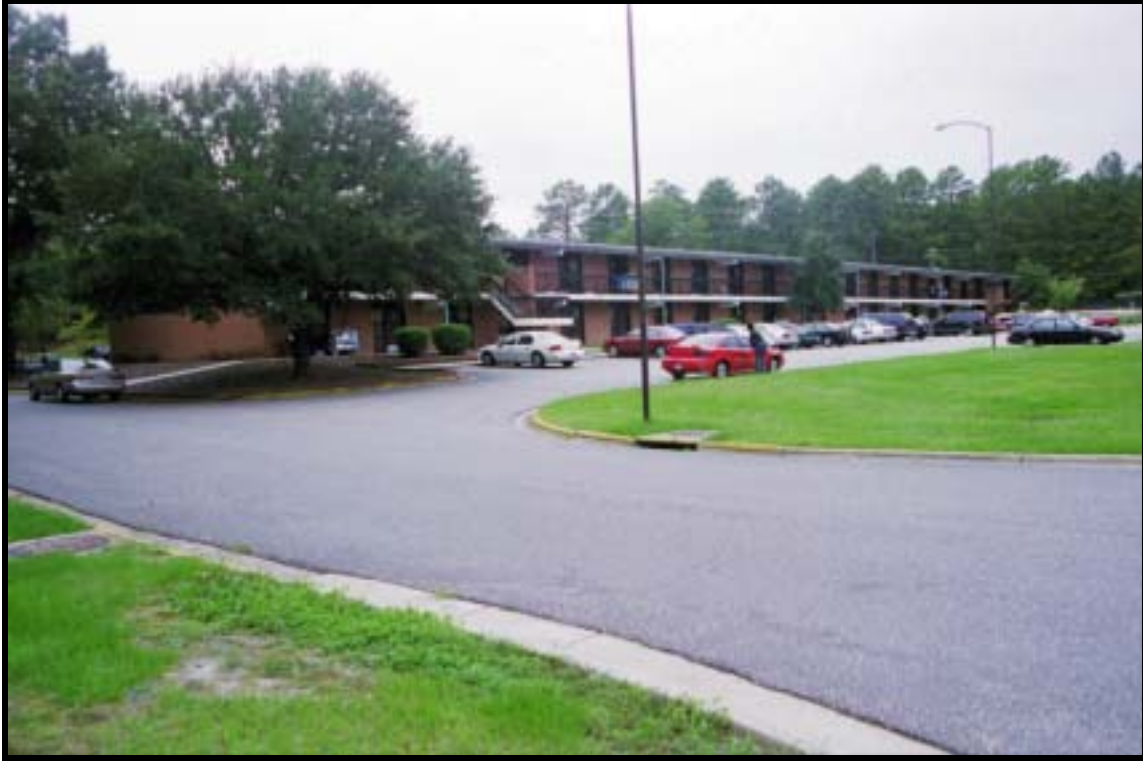
Figure 4.3.11 Transient quarter, Bldg. D-4218 (1971), Ft. Bragg, view SW (RCG&A).
