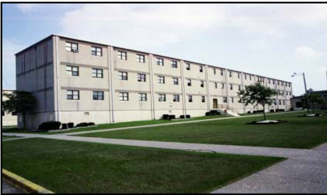
Figure 4.1.32 Alterations to hammerhead barracks include window replacements and new exterior materials, Bldg. C5322 (1955), Ft. Bragg, view SE (RCG&A).
