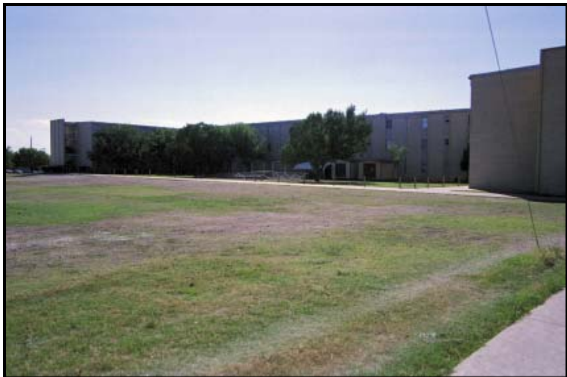
Figure 4.1.92 A-style barracks, Bldg. 41002 (1972), Ft. Hood, view SW (RCG&A).
