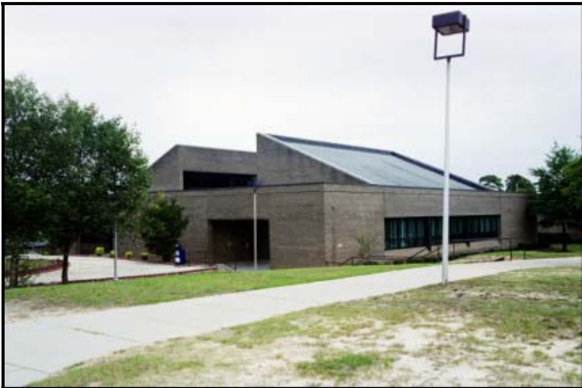
Figure 4.1.162 Quadrangle dining facility, Bldg. M-3234, Ft. Bragg, view SE (RCG&A).
