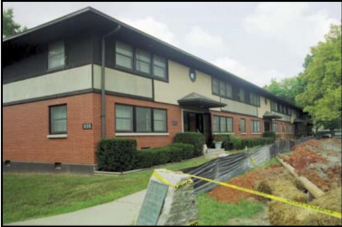
Figure 4.2.26 Two-story, apartment type women's BOQ, Bldg. 855 (1959), Ft. Knox, view W (RCG&A).
