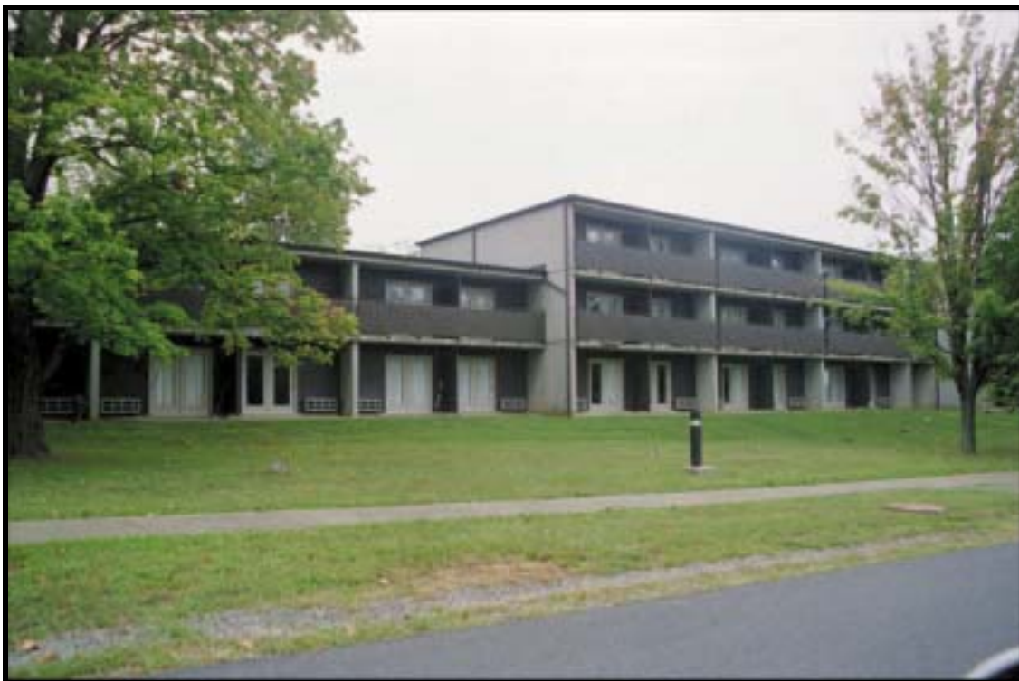
Figure 4.2.45 Apartment-type BOQ, Bldg. 2601 (1974), Ft. Knox, view SE (RCG&A).
