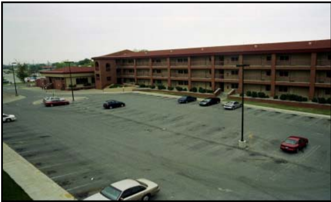
Figure 4.1.42 Totally renovated hammerhead barracks, Bldg. 1484 (1953), Ft. Knox, view NW (RCG&A).
