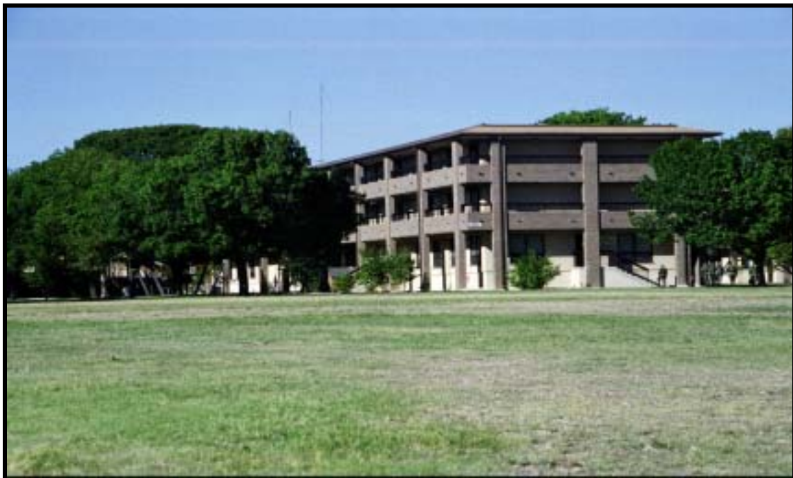
Figure 4.1.38 Rebuilt hammerhead barracks includes balconies and new exterior materials, Bldg. 9421 (1956), Ft. Hood, view N (RCG&A).
