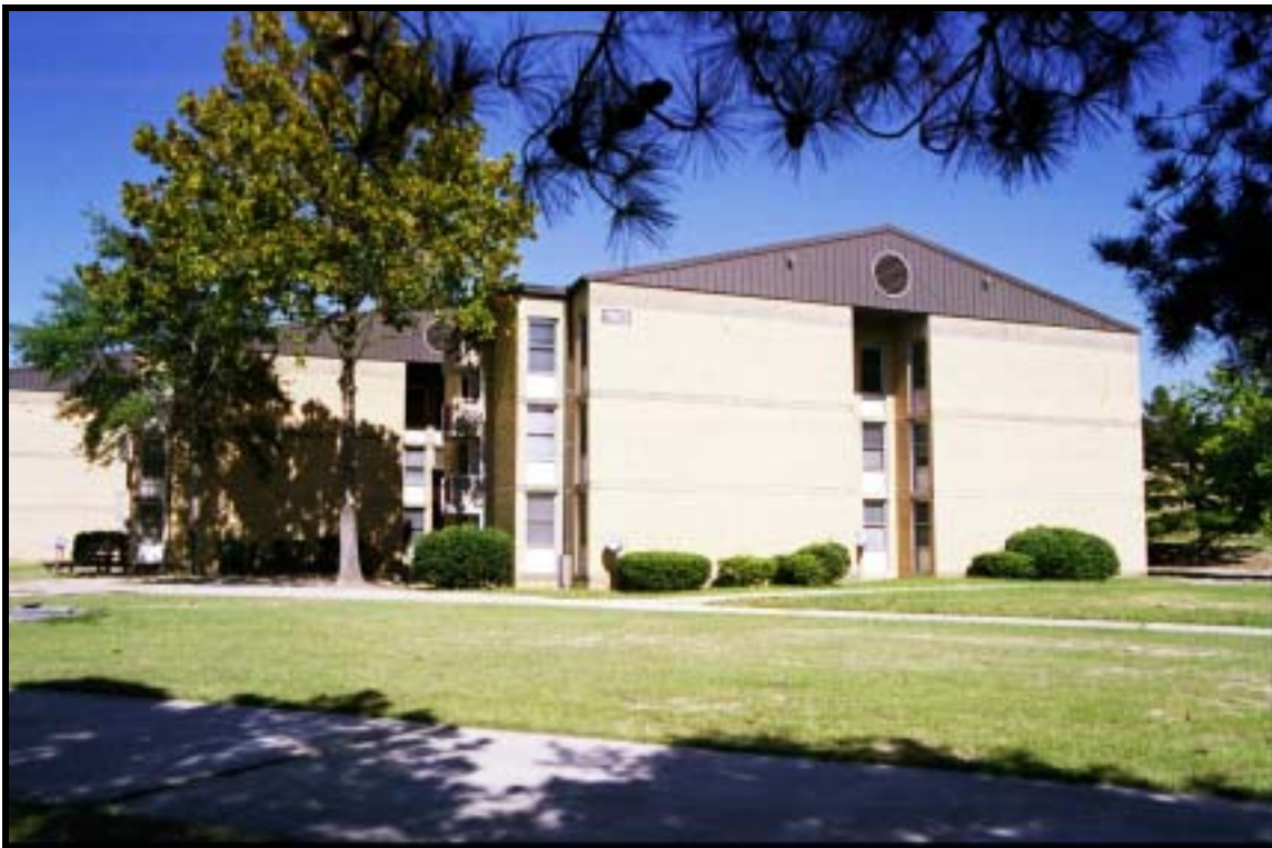
Figure 4.1.108 LBC&W barracks, Bldg. 1150 (1979), Ft. Polk, view NE (RCG&A).
