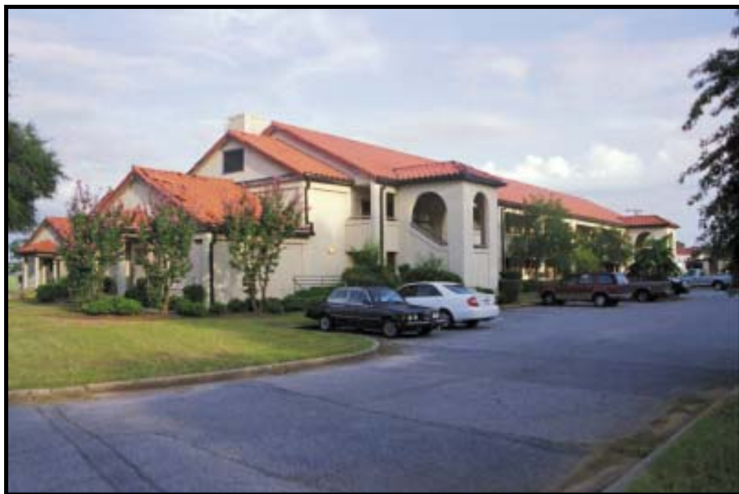
Figure 4.2.19 Renovated two-story, hammerhead UOQ, Bldg. 973 (1953), Ft. Benning, view NW (RCG&A).
