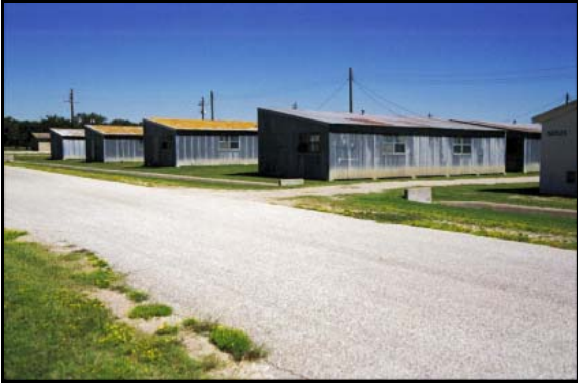
Figure 4.1.210 Overview of C-huts, North Ft. Hood, view E (RCG&A).
