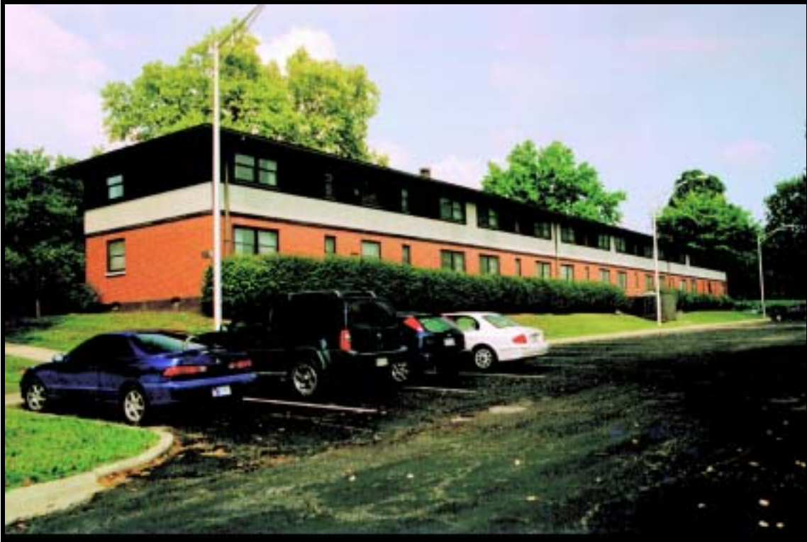
Figure 4.2.28 Two-story, apartment type women's BOQ, Bldg. 856 (1959), Ft. Knox, view N (RCG&A).
