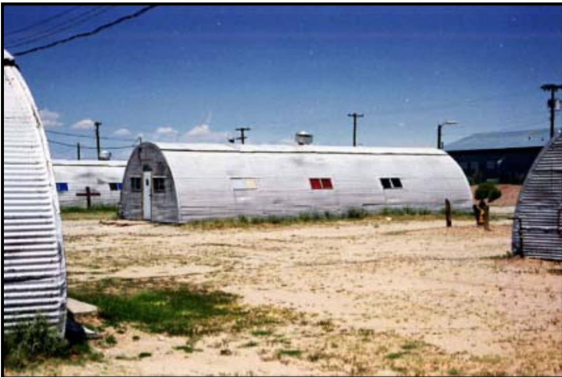
Figure 4.1.200 Quonset hut, Bldg. 8650 (1958), Oro Grande Range, Ft. Bliss, view NW (RCG&A).
