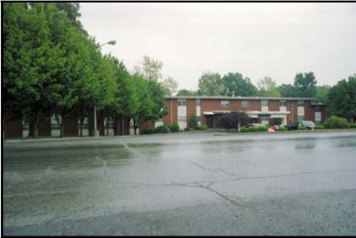
Figure 4.3.5 Transient quarter, Guest House, Bldg. 6597 (1970), Ft. Knox, view E (RCG&A).
