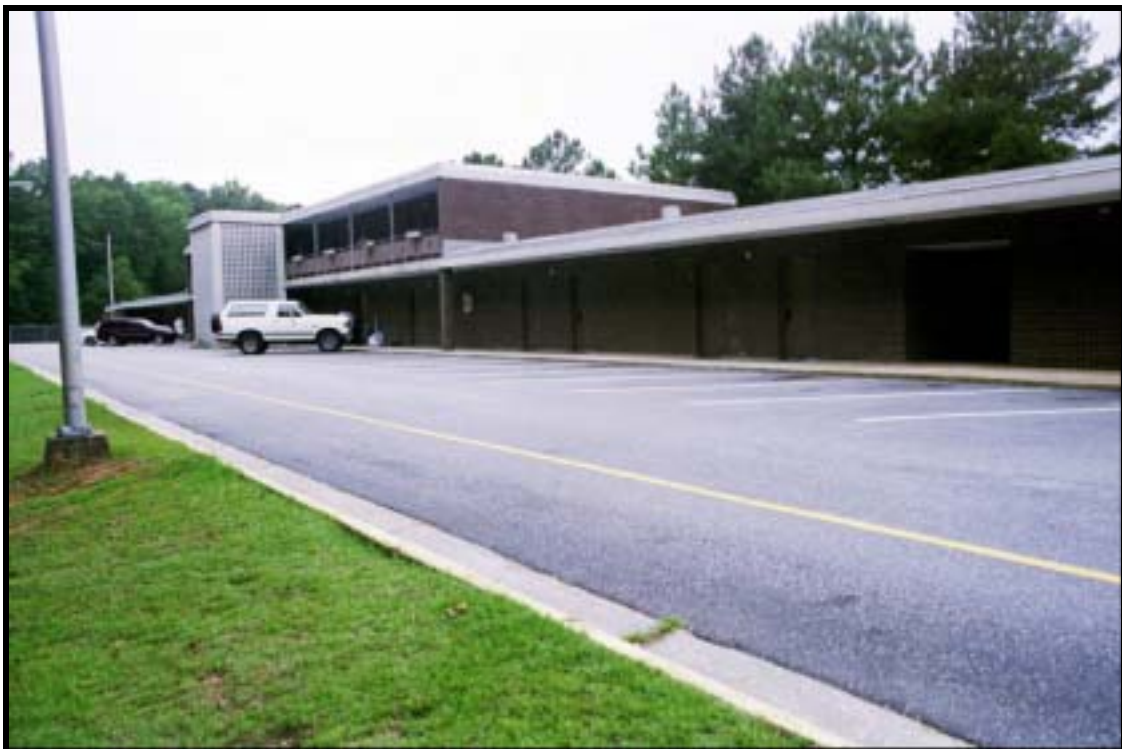
Figure 4.3.4 Transient quarter, Leal House, Bldg. 5-5047 (1969), Ft. Bragg, view SW (RCG&A).
