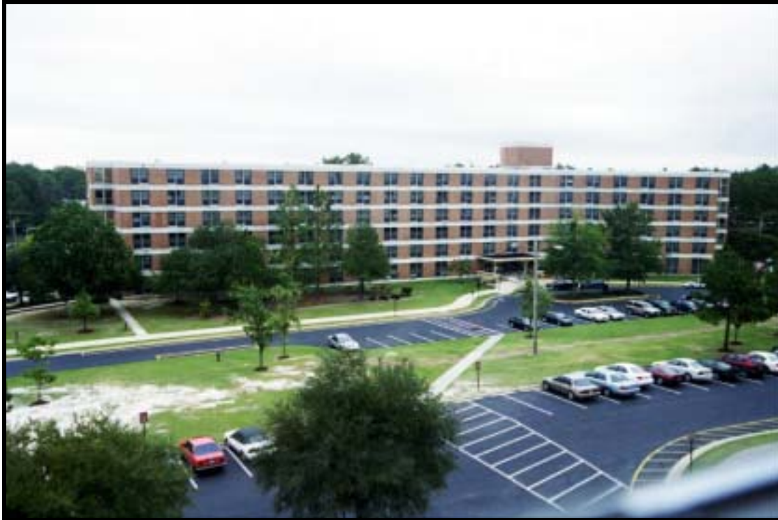
Figure 4.2.70 High Rise BOQ, Moon Hall, Bldg. C-3601 (1966), Ft. Bragg, view SE (RCG&A).
