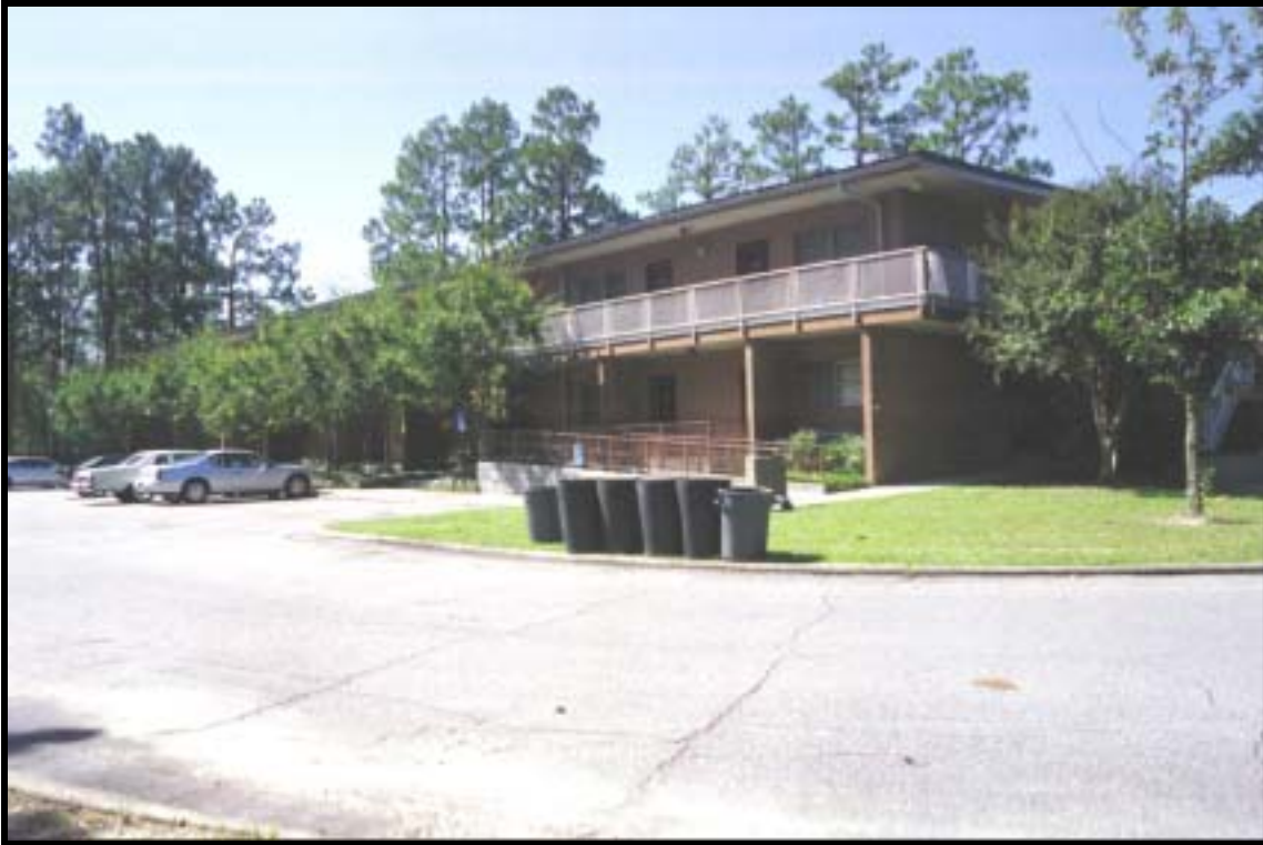
Figure 4.2.39 Motel-type BOQ, Bldg. 332 (1973), Ft. Polk, view W (RCG&A).
