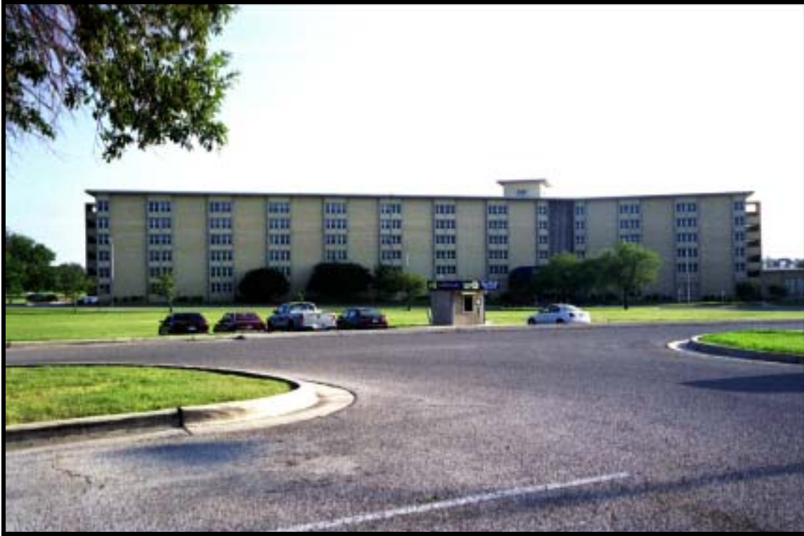
Figure 3.23 High-rise BOQ, Keith Ware Hall, Bldg. 36006 (1969), Ft. Hood, view N (RCG&A).
