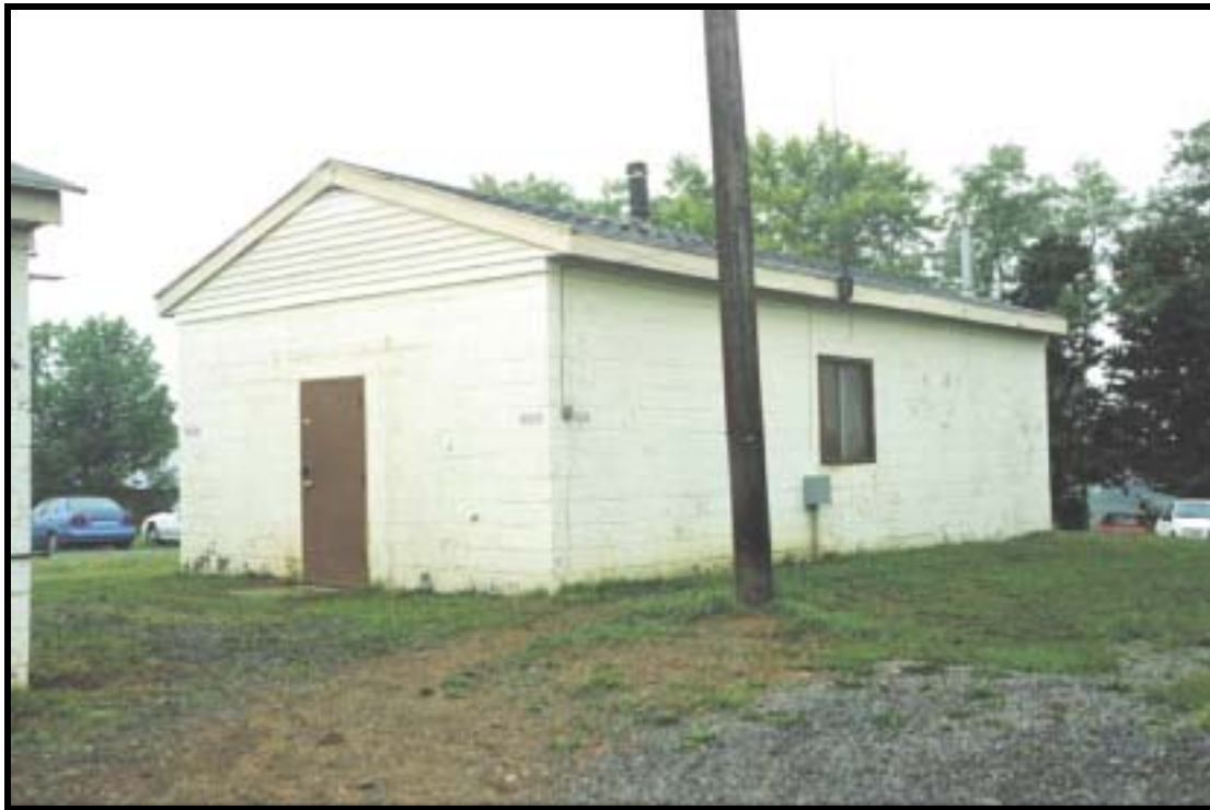
Figure 4.1.197 Hutment, Bldg. 9169 (1987), Ft. Knox, view SW (RCG&A).
