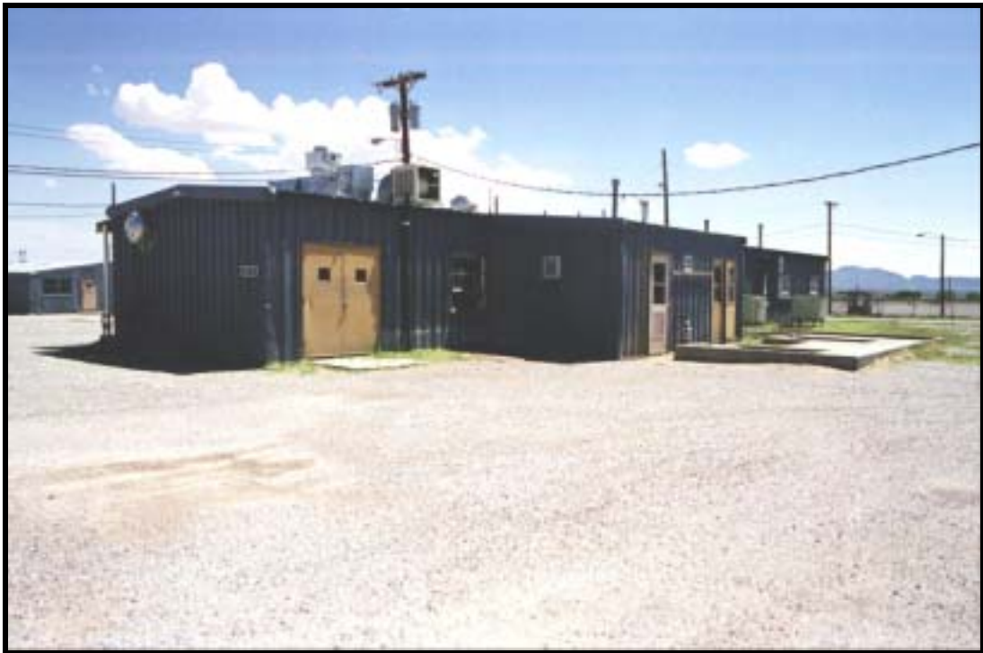
Figure 4.1.224 Mobilization dining facility, Bldg. 8160 (1966), Dona Ana Range, Ft. Bliss, view SW (RCG&A).
