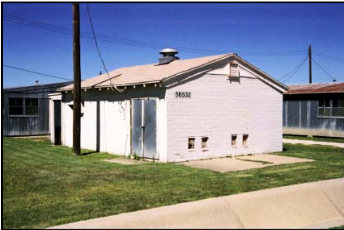
Figure 4.1.213 C-hut dining facility, Bldg. 56532 (1951), North Ft. Hood, view N (RCG&A).
