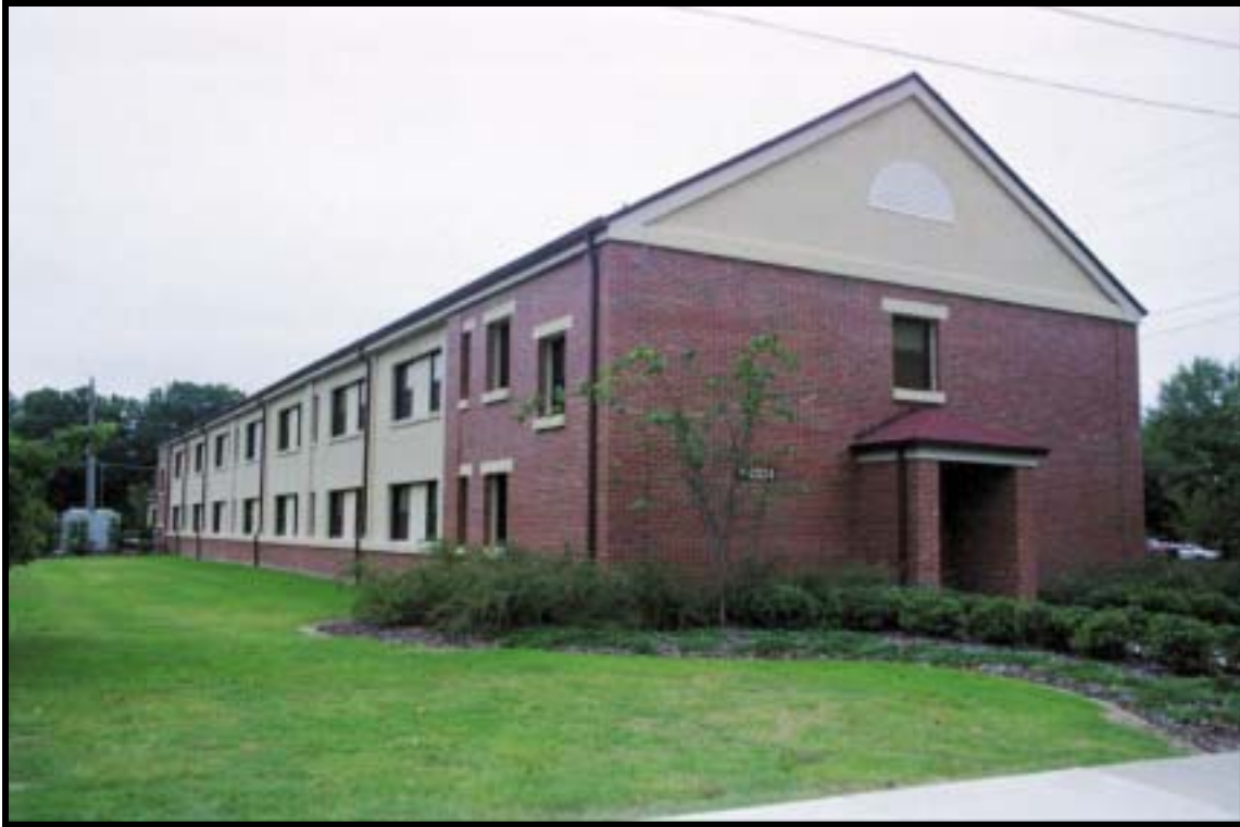
Figure 4.2.16 Renovated two-story, hammerhead BOQ, Bldg. 1-2334 (1953), Ft. Bragg, view S (RCG&A).
