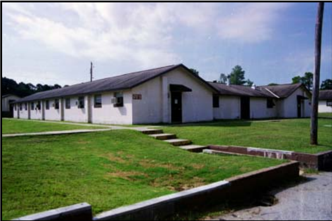
Figure 4.1.175 Semi-permanent 72-man “U” barracks, Bldg. 4707 (1967), Ft. Benning, view E (RCG&A).
