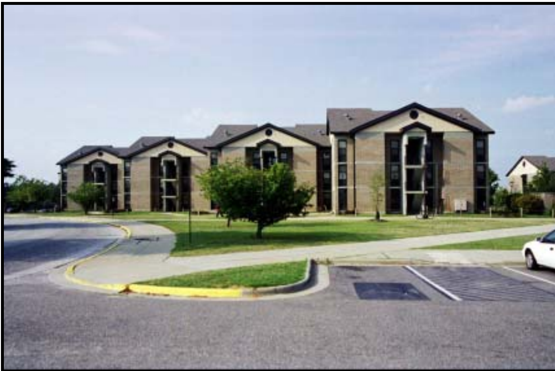
Figure 4.1.106 LBC&W barracks, Bldg. H-4812 (1980), Ft. Bragg, view N (RCG&A).
