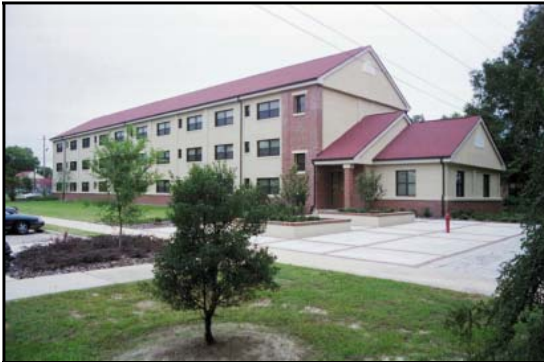
Figure 4.2.17 Renovated three-story, hammerhead BOQ, Bldg. 1-1938 (1955), Ft. Bragg, view NE (RCG&A).
