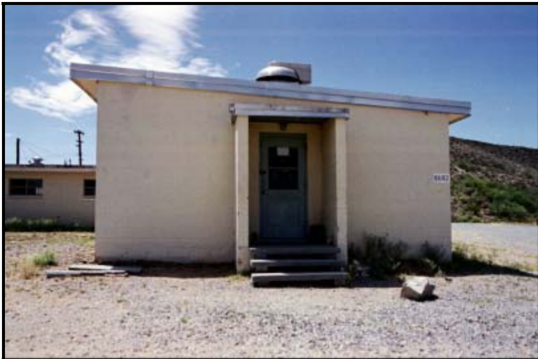
Figure 4.1.187 Door detail, Semi-permanent 80-man “H” barracks, Bldg. 8682 (1961), Oro Grande Range, Ft. Bliss, view SW (RCG&A).
