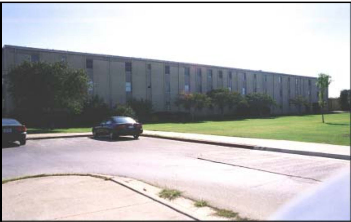
Figure 4.1.94 A-style barracks, Bldg. 41002 (1972), Ft. Hood, view SW (RCG&A).
