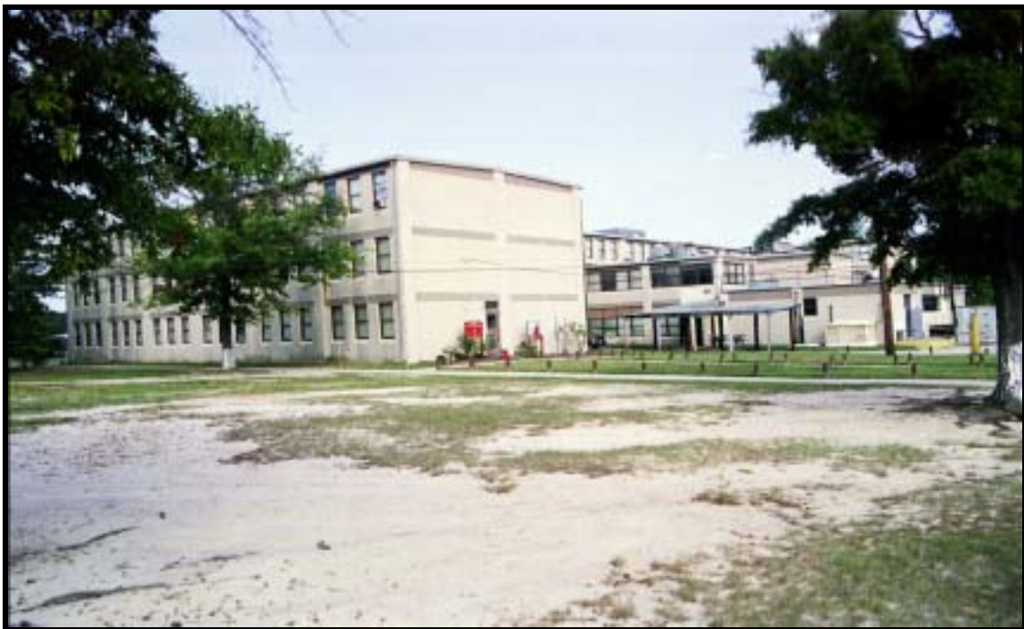
Figure 4.1.60 Alterations to H-style, two-company barracks include new windows and exterior materials, Bldg. C-9349 (1958), Ft. Bragg, view NW (RCG&A).
