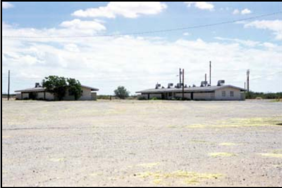
Figure 4.2.84 Semi-permanent 16-man BOQ, Bldg. S-8609, S-8610 (1961), Oro Grande Range, Ft. Bliss, view SE (RCG&A).
