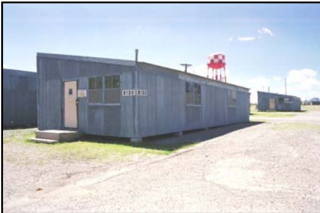
Figure 4.1.221 C-hut, Bldg. 8130 (1966), Dona Ana Range, Ft. Bliss, view W (RCG&A).
