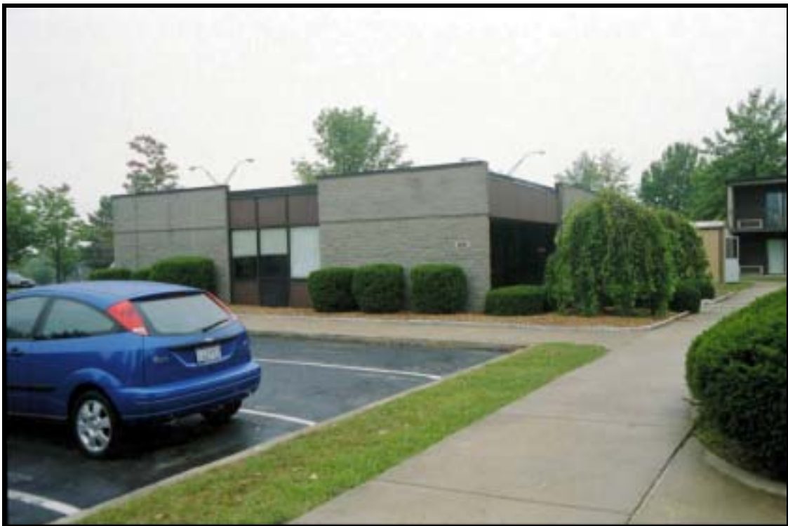
Figure 4.2.51 Community center converted to administration and supply, Bldg. 2608 (1974), Ft. Knox, view SW (RCG&A).
