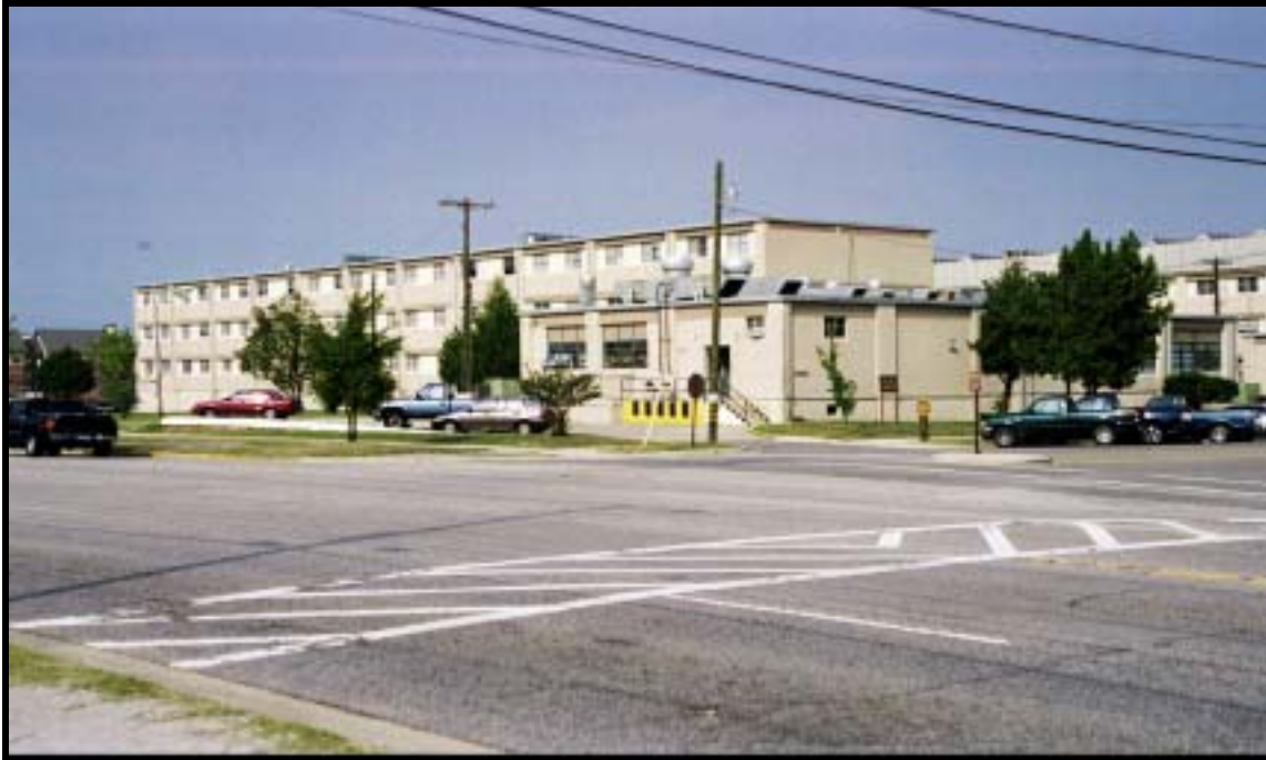
Figure 4.1.31 Small alterations to hammerhead barracks include infill of window openings, Bldg. C4120 (1955), Ft. Bragg, view N (RCG&A).
