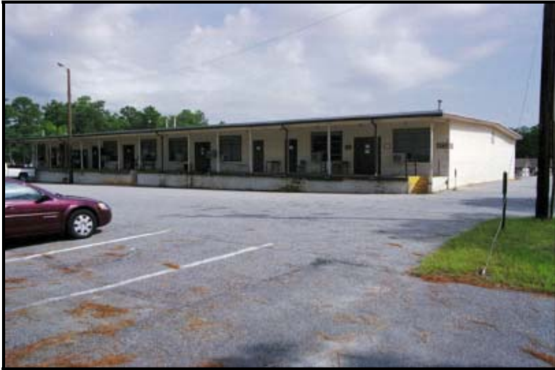
Figure 4.1.180 Semi-permanent administration and supply office, Bldg. 4713 (1967) Ft. Benning, view W (RCG&A).
