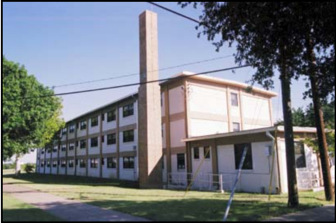
Figure 4.2.14 Three-story, hammerhead BOQ, Bldg. 5786 (1956), Ft. Hood, view SE (RCG&A).
