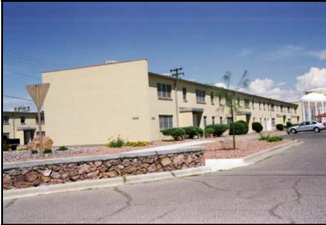
Figure 4.2.32 Two-story, apartment type BOQ, Bldg. 5042 (1962), Ft. Bliss, view SW (RCG&A).
