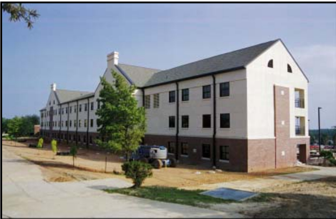
Figure 4.1.85 Renovated Rolling Pin, two-company barracks, Bldg. D-3142 (1971), Ft. Bragg, view SE (RCG&A).
