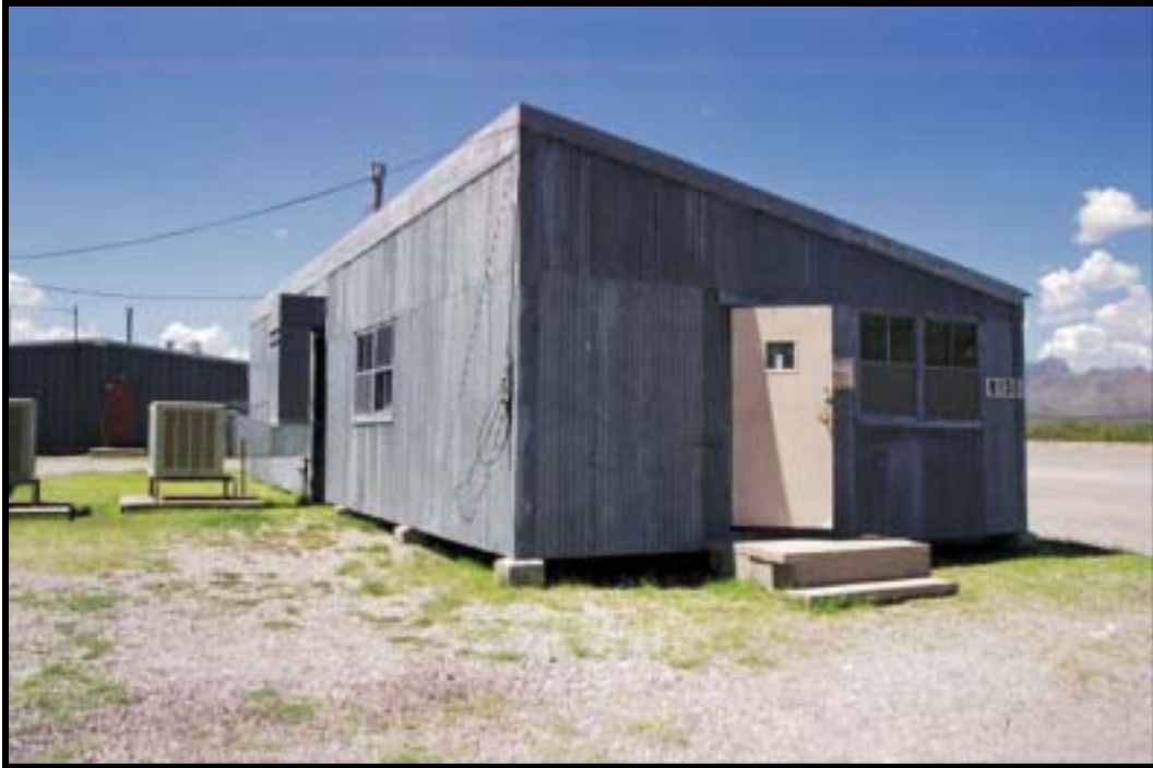
Figure 4.1.220 C-hut, Bldg. 8130 (1966), Dona Ana Range, Ft. Bliss, view NW (RCG&A).
