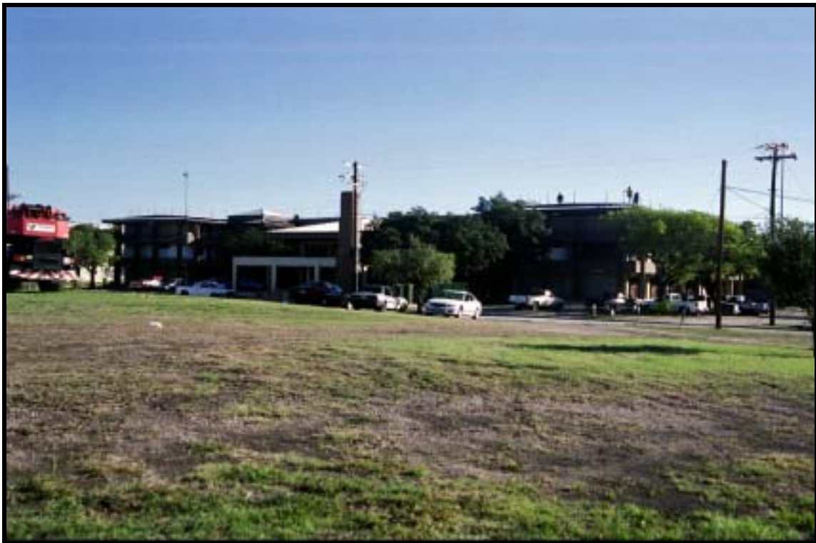
Figure 4.1.64 Renovated H-style, two-company barracks, Bldg. 9210 (1958), Ft. Hood, view NE (RCG&A).
