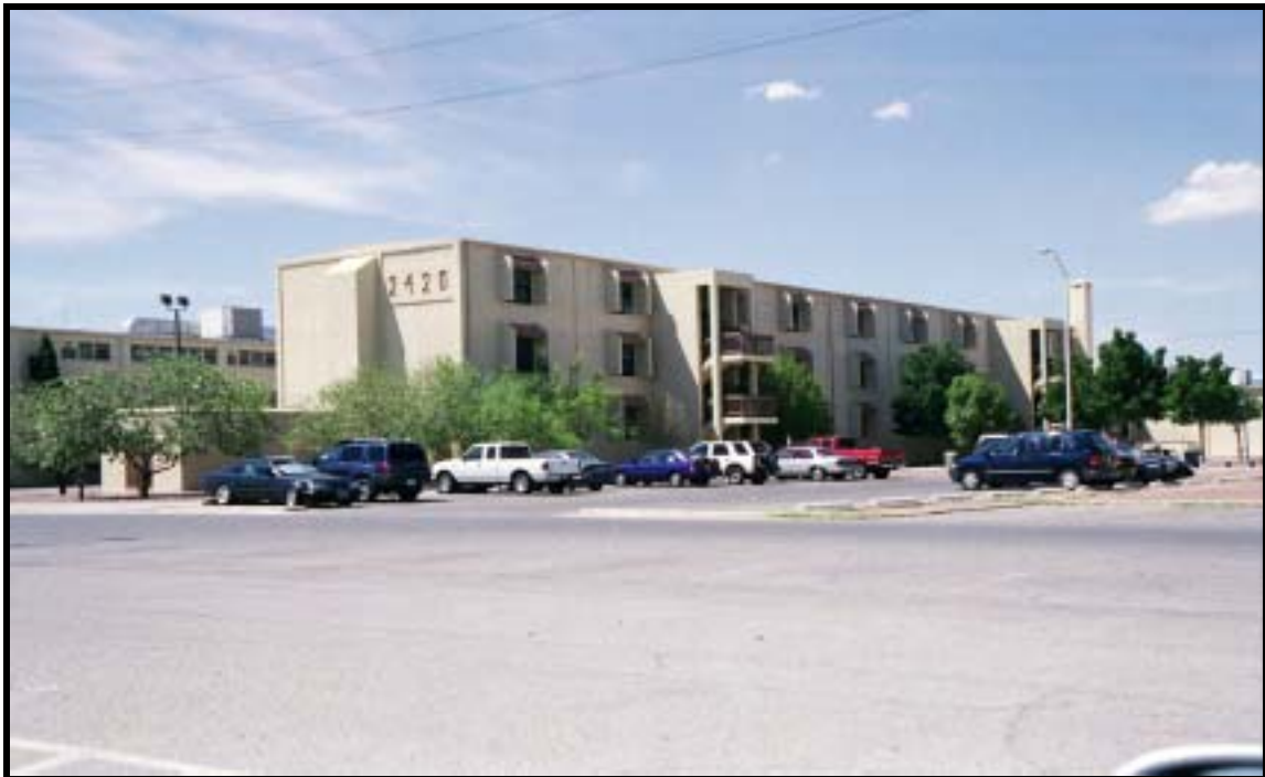
Figure 4.1.36 Extensive renovation to hammerhead barracks include new windows, window treatments, and exterior materials, Bldg. 2420 (1953), Ft. Bliss, view NW (RCG&A).
