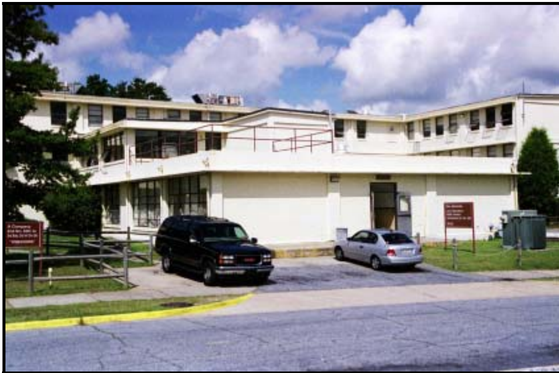
Figure 4.1.54 H-style, two-company barracks, Bldg. 9021 (1958), Kelley Hill, Ft. Benning, view NW (RCG&A)
