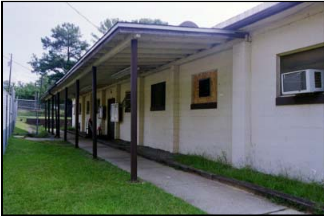
Figure 4.1.176 Semi-permanent dining facility, Bldg. 4702 (1967), Ft. Benning, view N (RCG&A).
