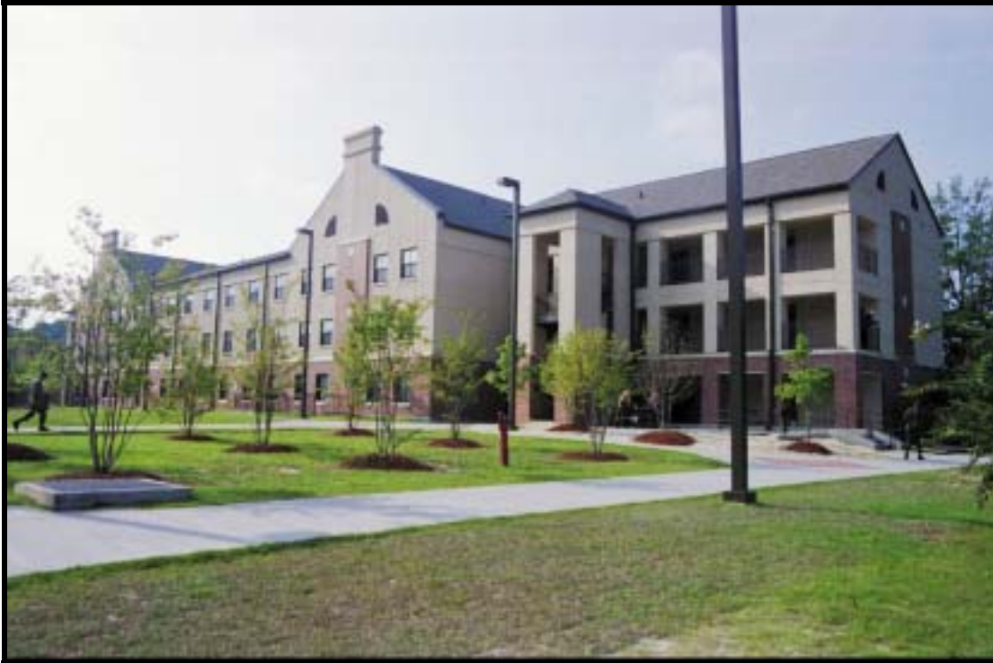
Figure 4.1.84 Renovated Rolling Pin, two-company barracks, Bldg. D-3545 (1971), Ft. Bragg, view NW (RCG&A).
