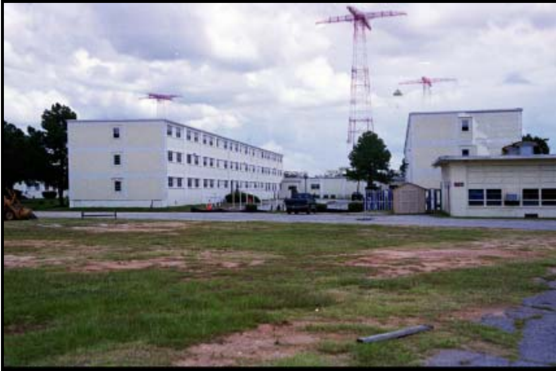
Figure 4.1.27 Double hammerhead barracks, Bldg. 2753 A&B (1954), Ft. Benning, view NE (RCG&A).
