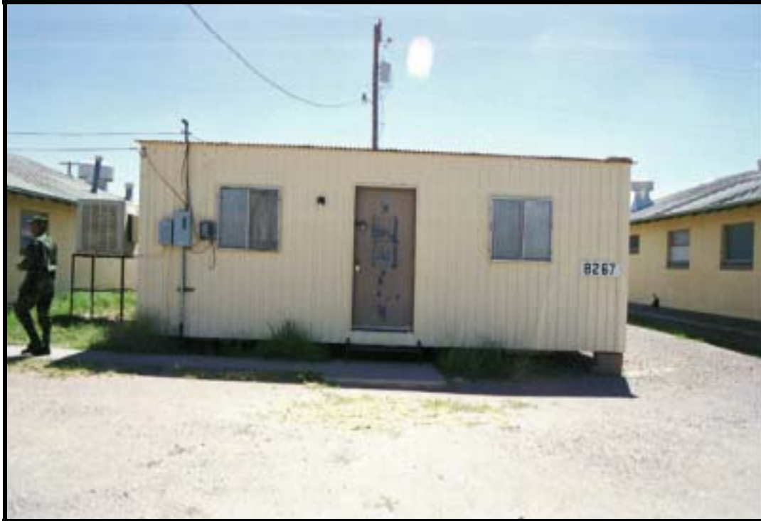
Figure 4.2.86 Mobilization BOQ, Bldg. 8267 (1983), Dona Ana Range, Ft. Bliss, view SW (RCG&A).
