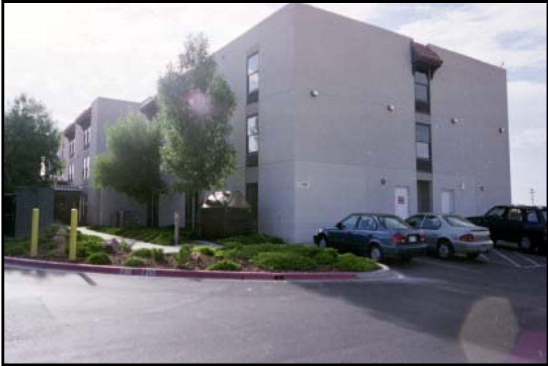
Figure 4.3.18 Transient quarter, The Inn at Ft. Bliss, Bldg. 1744 (1989), view SE (RCG&A).
