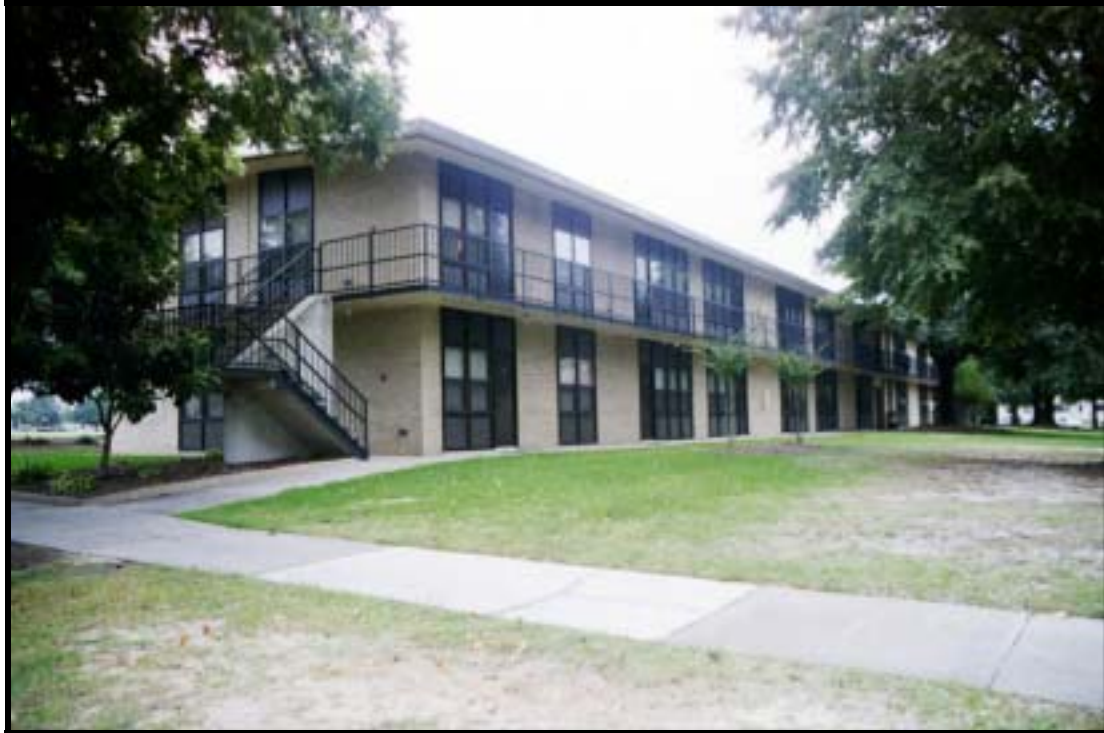
Figure 4.2.36 120-man motel type BOQ, Bldg. 1-1939 (1968), Ft. Bragg, view SE (RCG&A).
