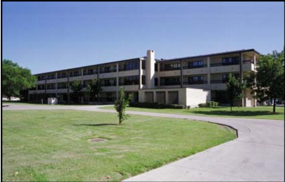
Figure 4.1.82 Renovated Rolling Pin, two-company barracks, Bldg. 41009 (1969), Ft. Hood, view SE (RCG&A).
