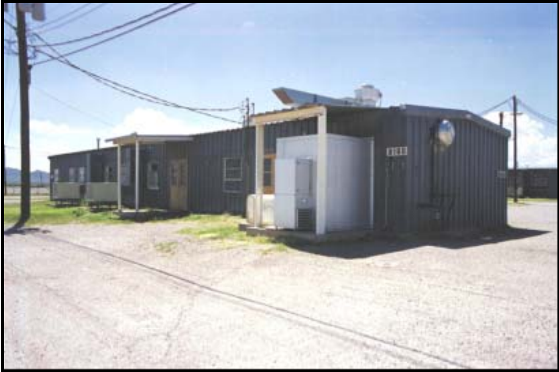
Figure 4.1.223 Mobilization dining facility, Bldg. 8160 (1966), Dona Ana Range, Ft. Bliss, view E (RCG&A).
