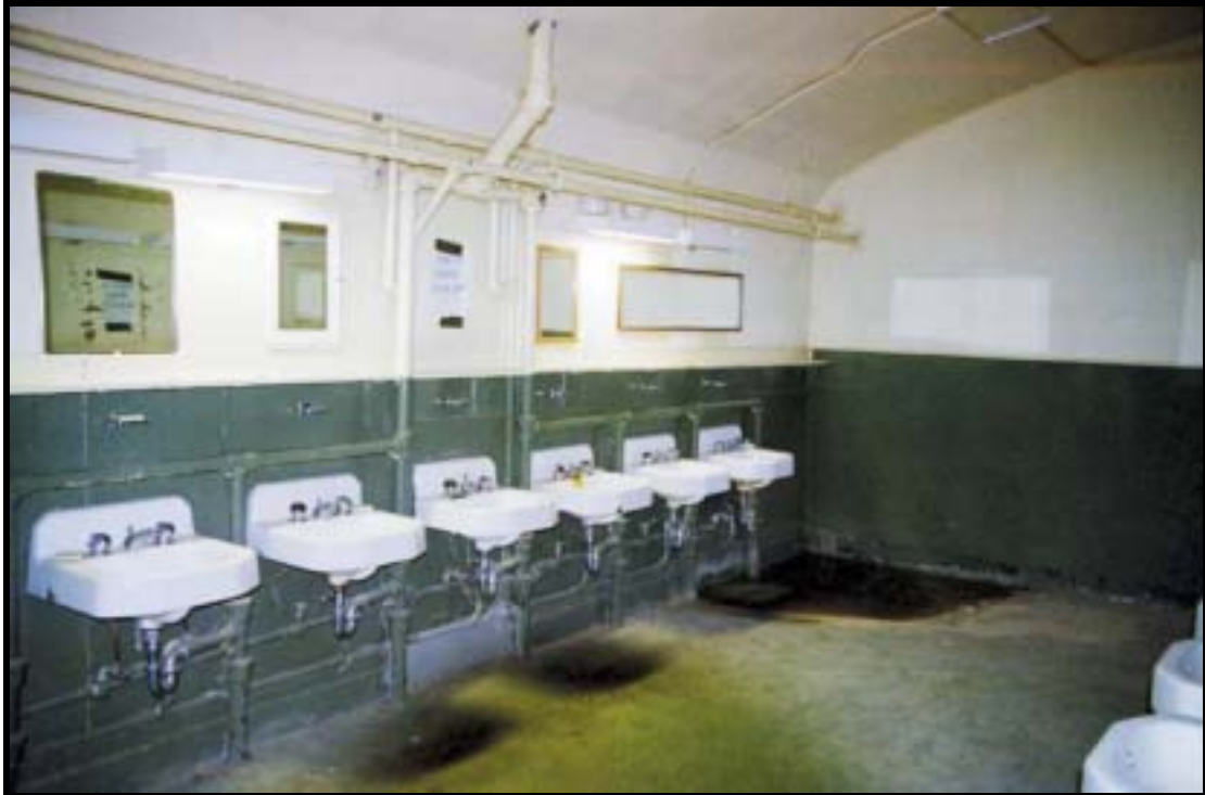
Figure 4.1.205 Interior of Bldg. 8627 (1959), Oro Grande Range, Ft. Bliss, view E (RCG&A).
