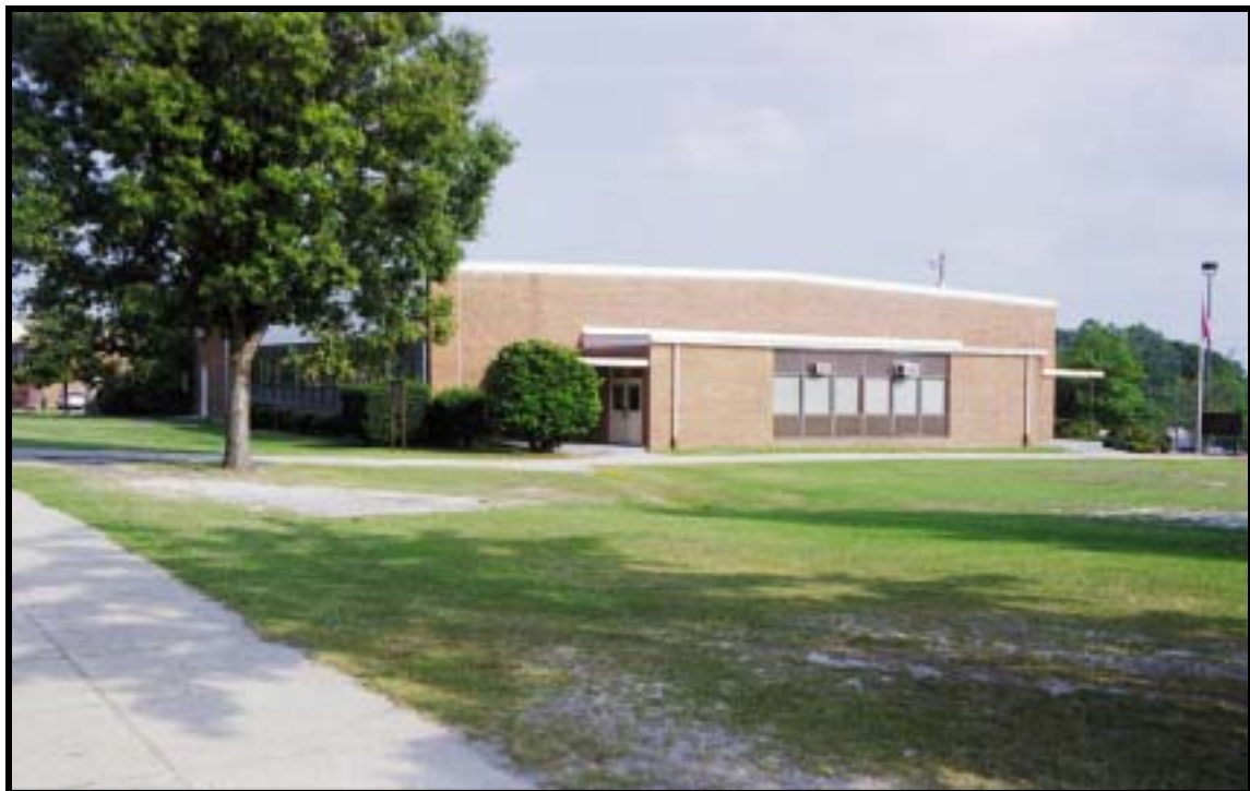
Figure 4.1.79 Rolling Pin dining facility, Bldg. D-3148 (1971), Ft. Bragg, view SE (RCG&A).
