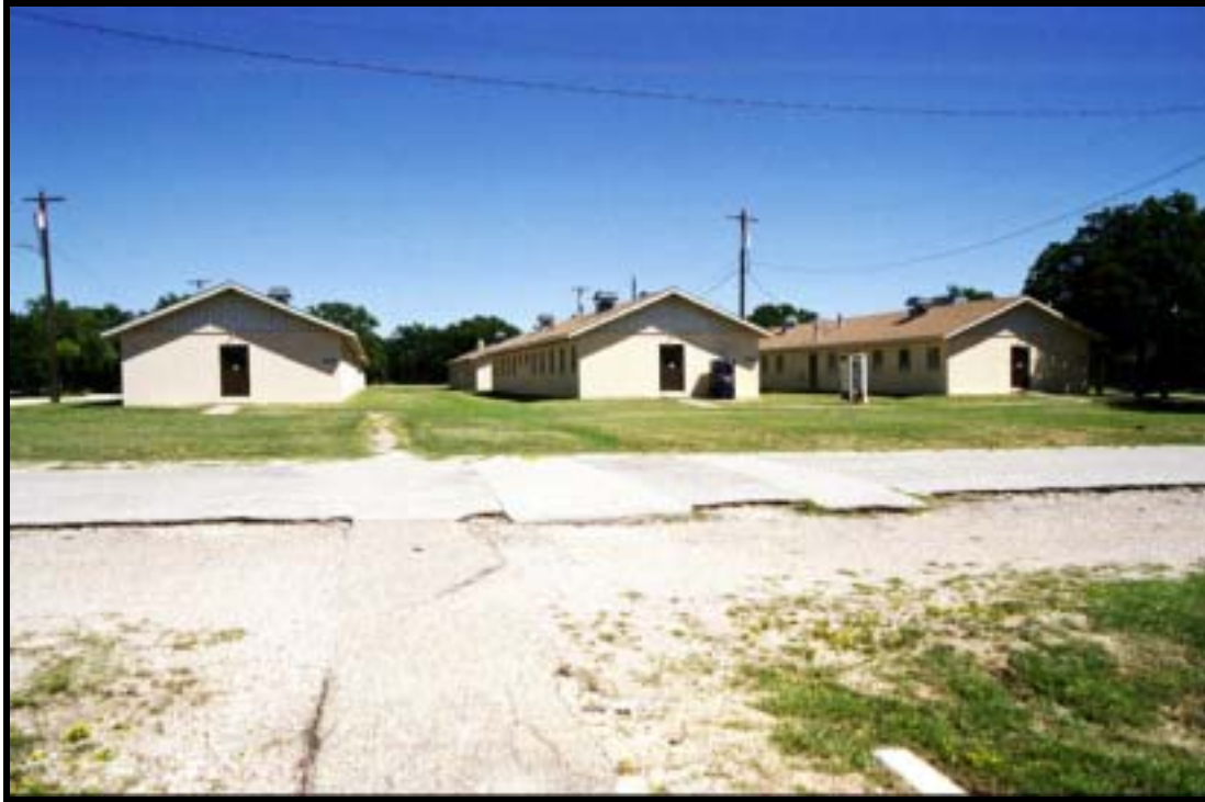
Figure 4.2.53 Army Reserve Annual Training UOQ, Bldg. 56354, 56352, 56350 (1979), Ft. Hood, view E (RCG&A).
