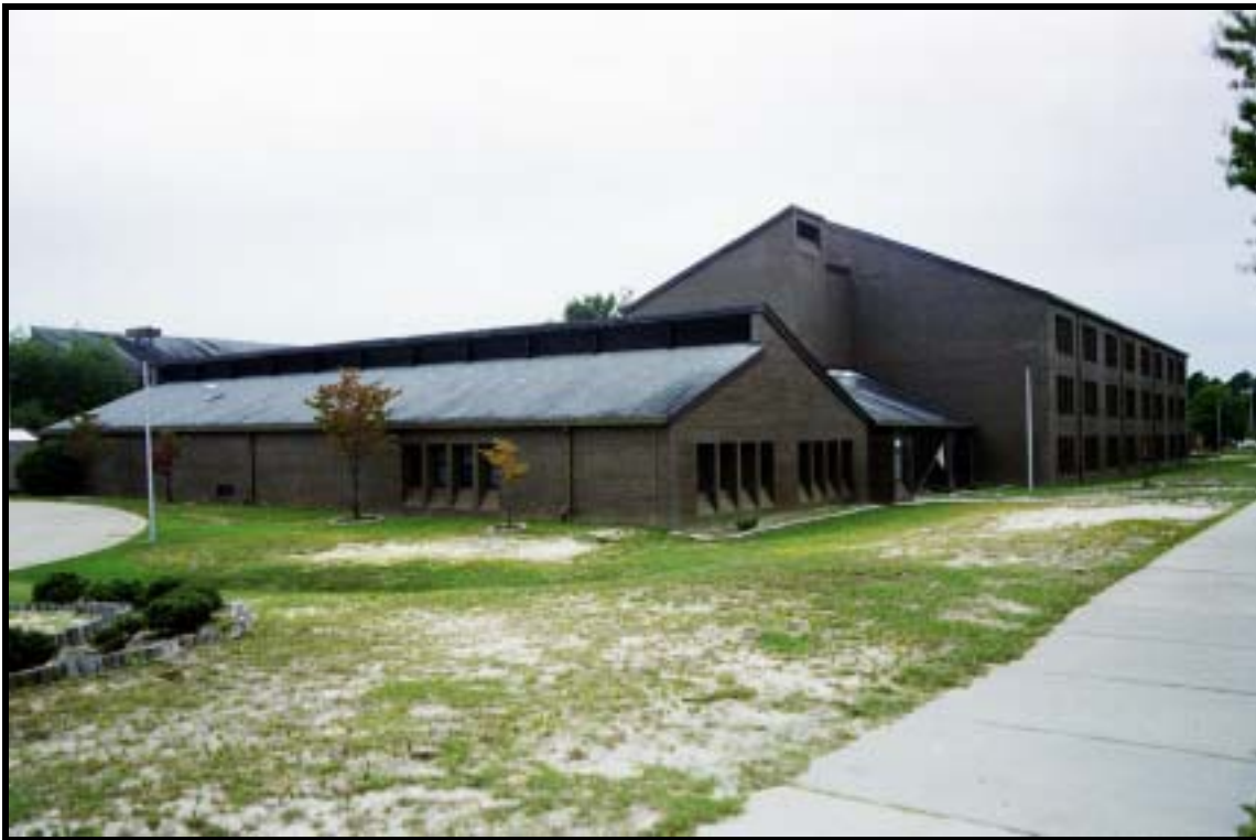
Figure 3.17 Quadrangle barracks, Bldg. M-4020 (1985), Ft. Bragg, view NE (RCG&A).
