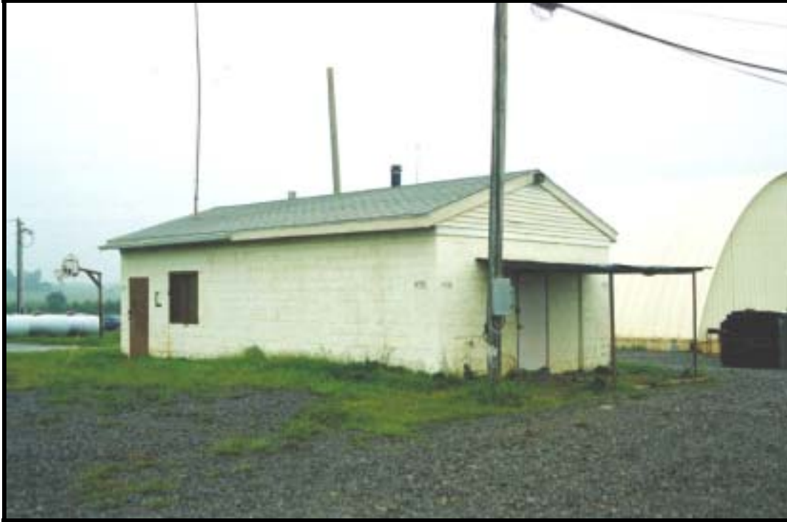
Figure 4.1.196 Hutment, Bldg. 9170 (1987), Ft. Knox, view NE (RCG&A).
