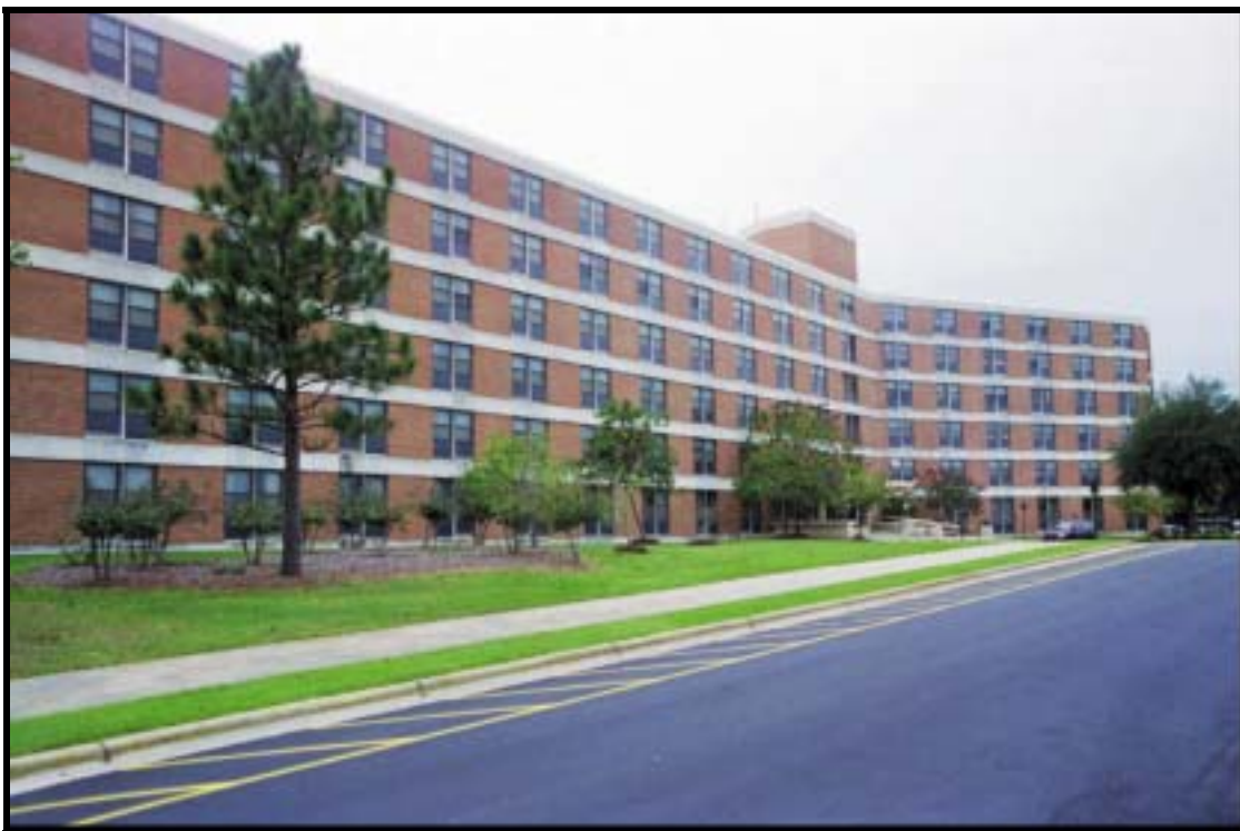
Figure 4.2.71 High Rise BOQ, Hardy Hall, Bldg. C-3703 (1966), Ft. Bragg, view NW (RCG&A).
