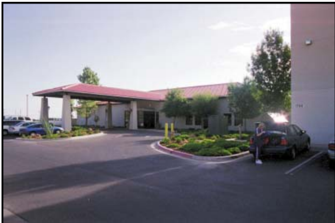
Figure 4.3.19 Transient quarter addition, The Inn at Ft. Bliss, Bldg. 1744 (1989), view NE (RCG&A).
