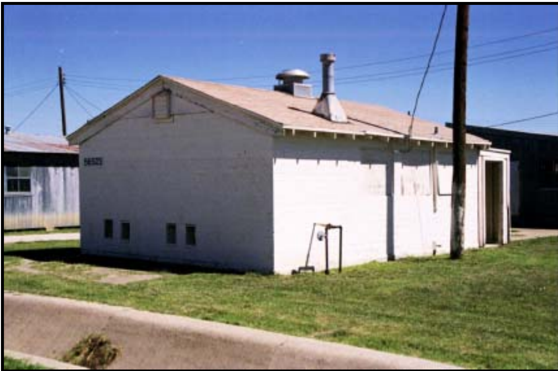
Figure 4.1.215 C-hut dining facility, Bldg. 56523 (1951), North Ft. Hood, view E (RCG&A).
