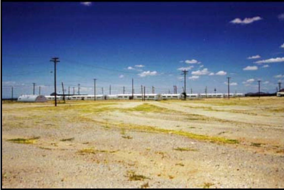
Figure 4.1.201 Overview of mobilization barracks, Oro Grande Range, Ft. Bliss, view N (RCG&A).
