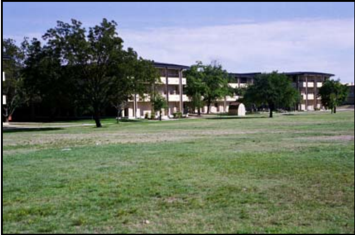
Figure 4.1.63 Renovated H-style, two-company barracks, Bldg. 14023 (1958), Ft. Hood, view SE (RCG&A).
