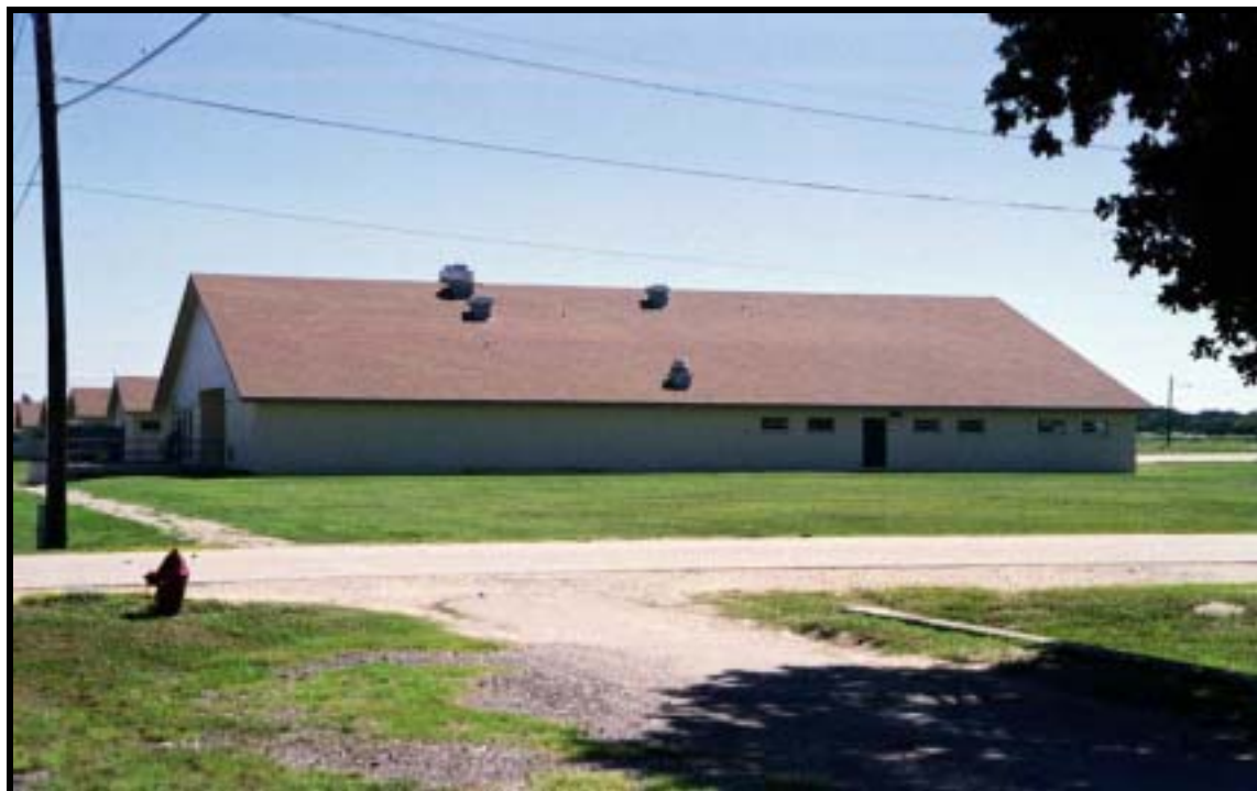
Figure 4.1.126 Army Reserve Annual Training dining facility, Bldg. 56440 (1979), North Ft. Hood, view S (RCG&A).
