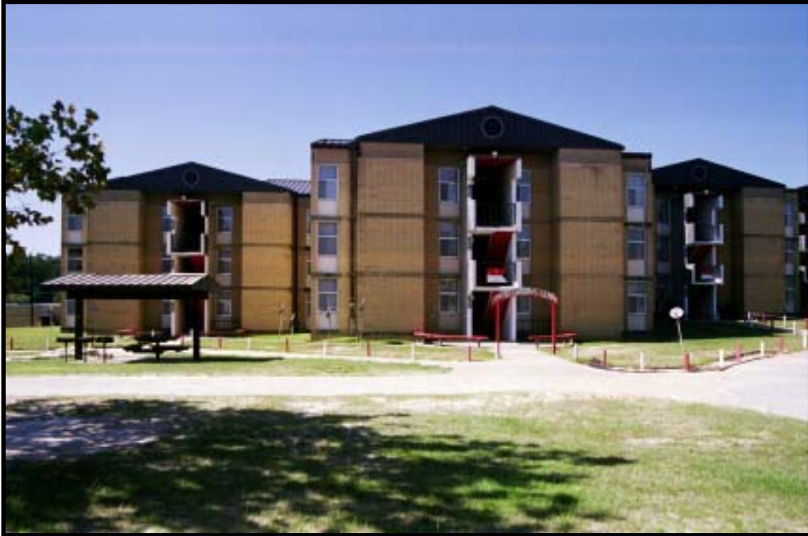
Figure 4.107 LBC&W barracks, Bldg. 1054 (1979), Ft. Polk, view NW (RCG&A).
