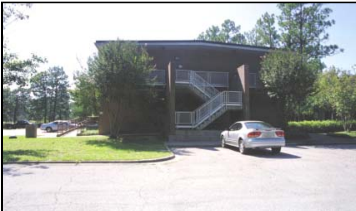
Figure 4.2.40 Motel-type BOQ, Bldg. 332 (1973), Ft. Polk, view SW (RCG&A).
