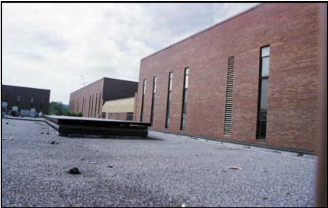
Figure 4.1.142 Starship barracks, Bldg. 3105 (1988), Ft. Benning, view S (RCG&A).
