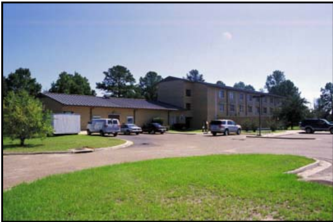
Figure 4.1.169 MEDDAC barracks, Bldg. 293 (1988), Ft. Polk, view SE (RCG&A).
