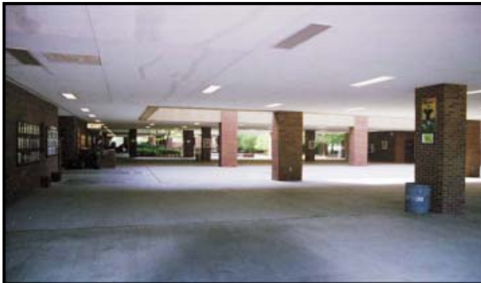
Figure 4.1.140 Starship barracks, Bldg. 3105 (1988), cadre area, Ft. Benning, view SE (RCG&A).
