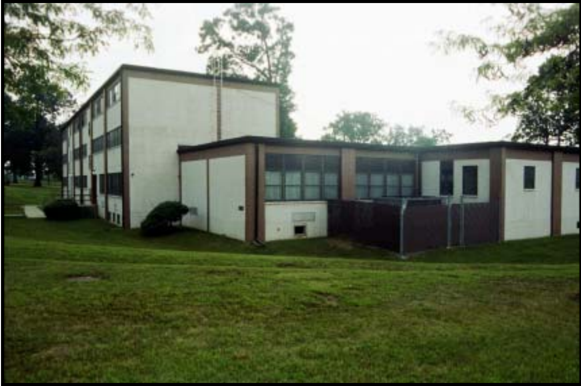
Figure 4.1.22 105-man hammerhead barracks, Bldg. 296 (1954), Ft. Knox, view S (RCG&A).
