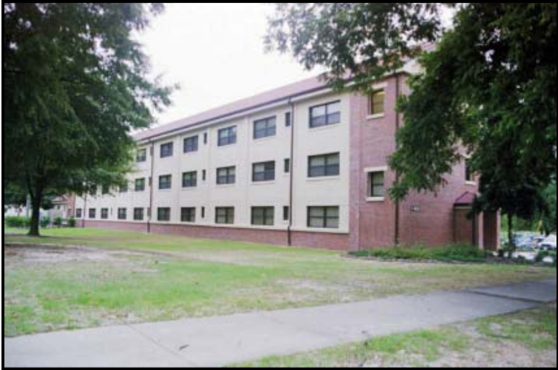
Figure 4.2.18 Renovated three-story, hammerhead BOQ, Bldg. 1-1938 (1955), Ft. Bragg, view SW (RCG&A).
