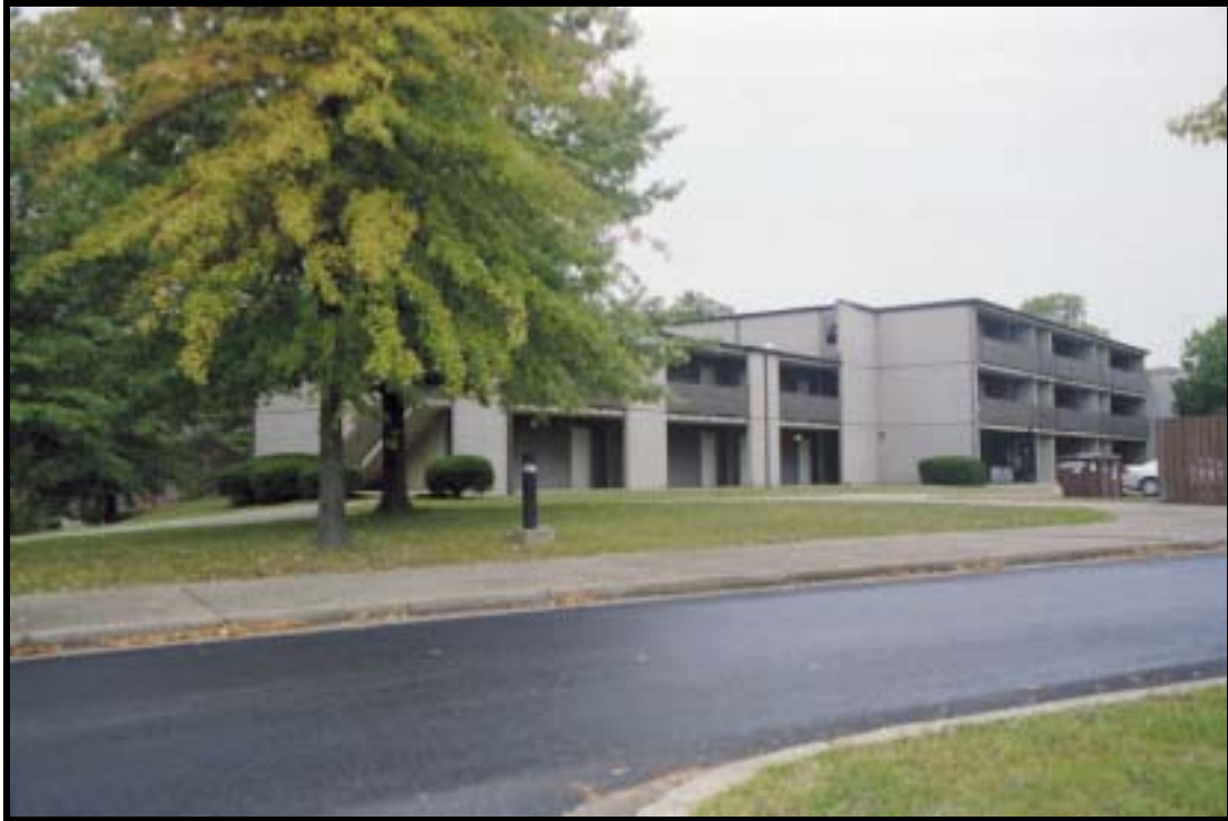
Figure 4.2.44 Apartment-type BOQ, Bldg. 2601 (1974), Ft. Knox, view NW (RCG&A).
