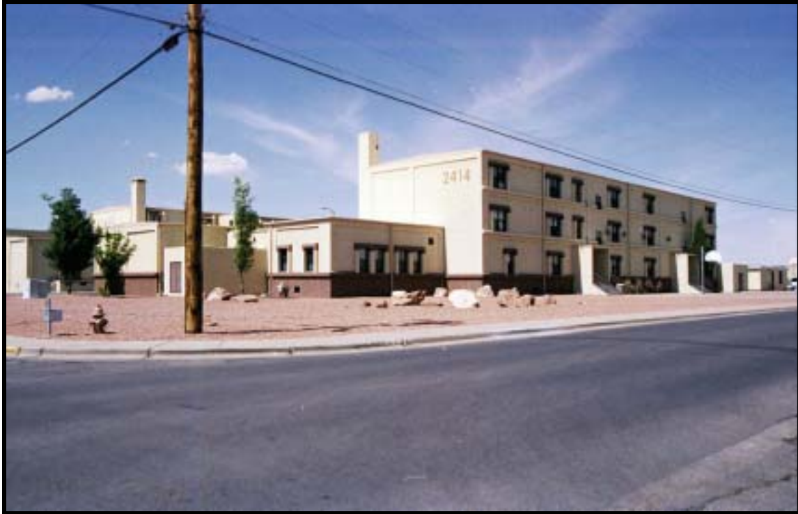
Figure 4.1.35 Alterations to 105-man hammerhead barracks include new windows and exterior materials, Bldg 2414 (1953), Ft. Bliss, view NW (RCG&A).
