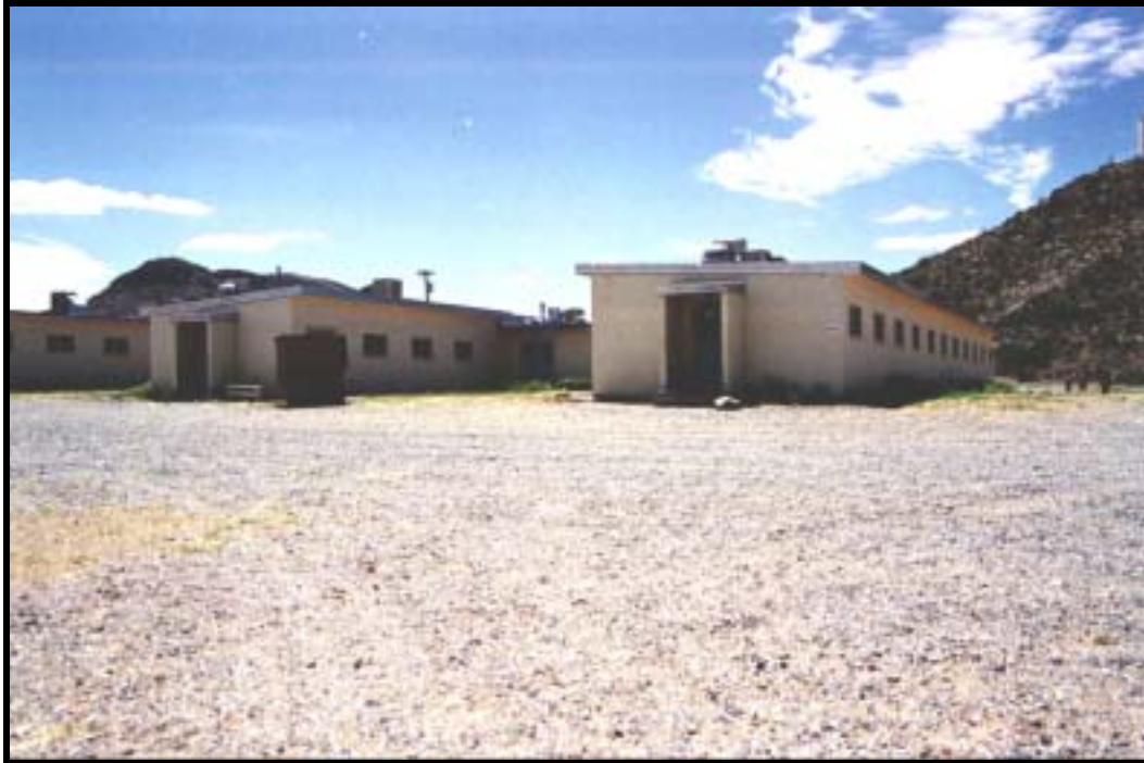
Figure 4.1.186 Semi-permanent 80-man “H” barracks, Bldg. 8682 (1961), Oro Grande Range, Ft. Bliss, view S (RCG&A).
