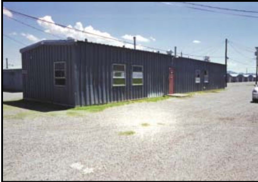
Figure 4.1.226 Mobilization latrine, Bldg. 8128 (1966), Dona Ana Range, Ft. Bliss, view E (RCG&A).
