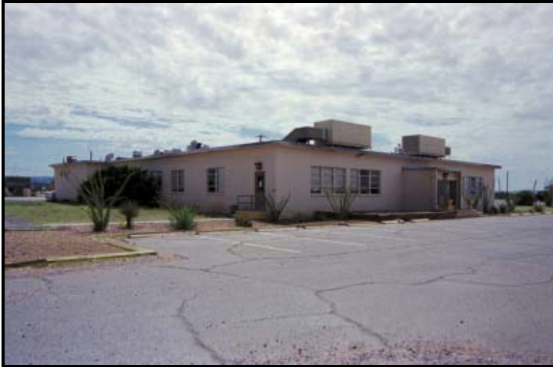
Figure 4.1.194 Semi-permanent dining facility, Bldg. 9510 (1957), McGregor Range, Ft. Bliss, view SE (RCG&A).
