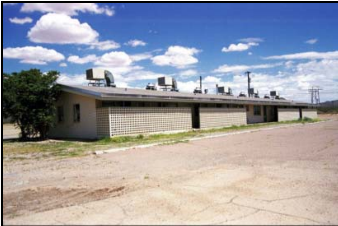
Figure 4.2.85 Semi-permanent 16-man BOQ, Bldg. S-8610 (1961), Oro Grande Range, Ft. Bliss, view NE (RCG&A).
