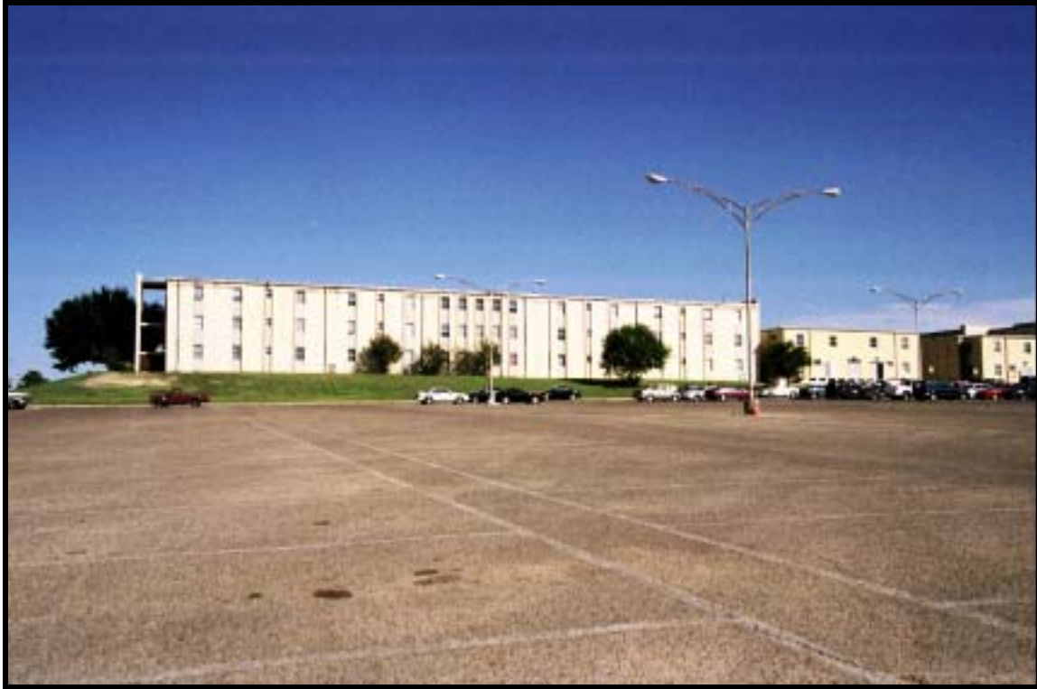
Figure 4.1.91 A-style barracks, Bldg. 34006 (1974), Ft. Hood, view E (RCG&A).
