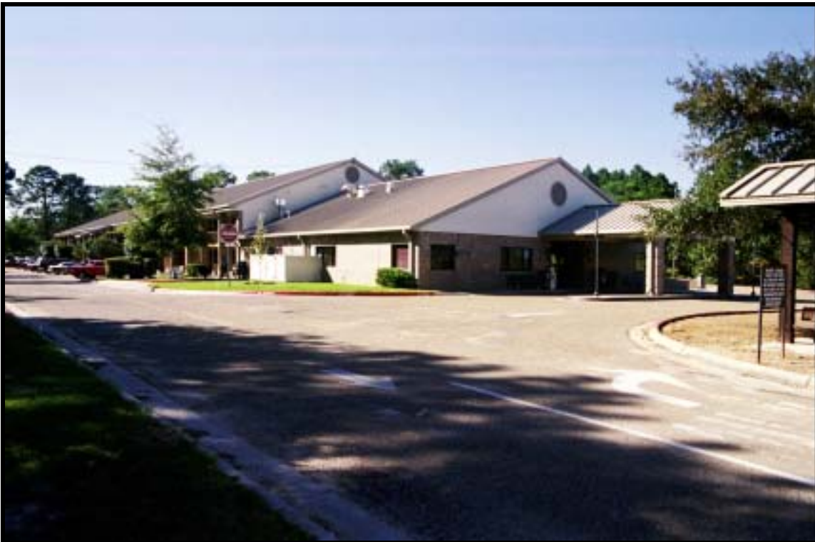
Figure 3.30 Transient quarter, Guest House, Bldg. 522 (1988), Ft. Polk, view NW (RCG&A).
