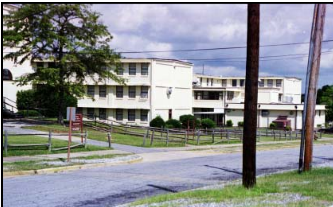
Figure 4.1.55 Detail of mess wing, H-style, two-company barracks, Bldg. 9021 (1958), Kelley Hill, Ft. Benning, view W (RCG&A).
