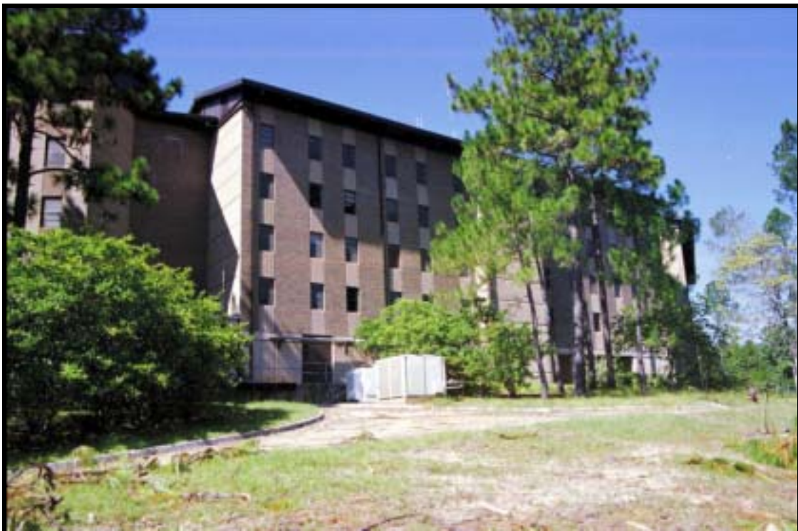
Figure 4.2.79 High Rise BOQ, Woodfill Hall, Bldg. 350 (1979), Ft. Polk, view NW (RCG&A).
