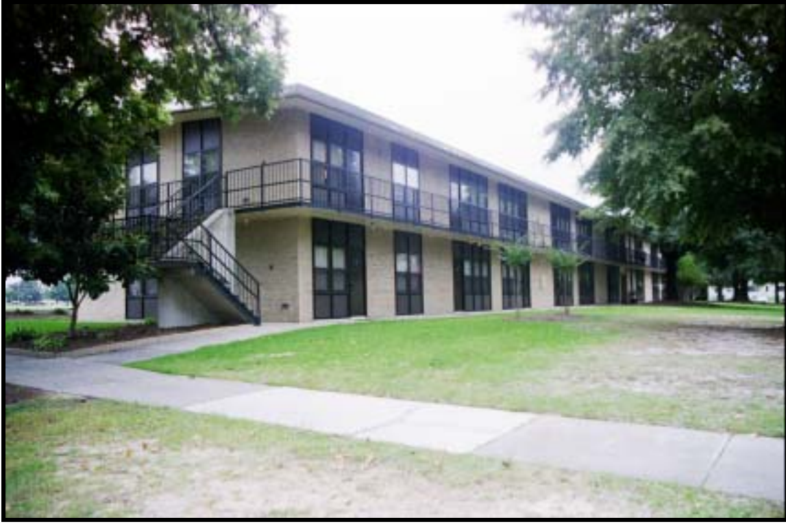
Figure 3.22 120-man motel-type BOQ, Bldg. 1-1939 (1968), Ft. Bragg, view SE (RCG&A).
