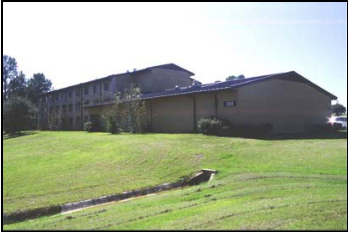
Figure 4.1.168 MEDDAC barracks, Bldg. 293 (1988), Ft. Polk, view SW (RCG&A).
