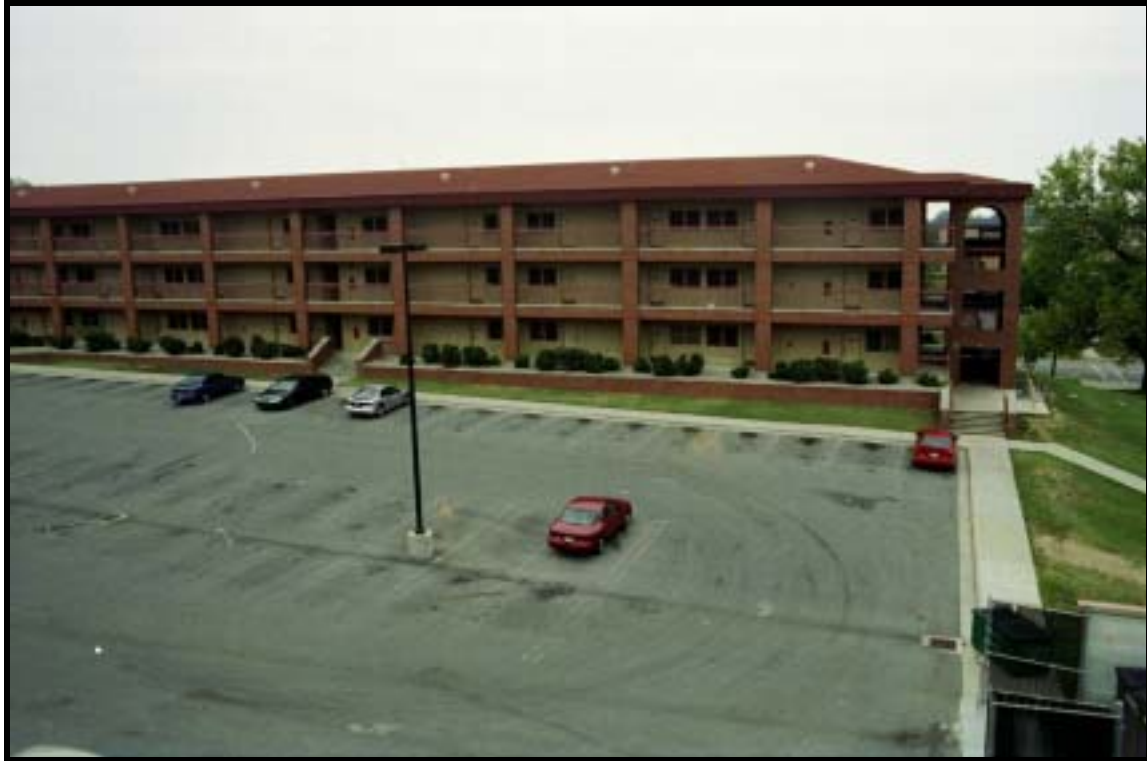
Figure 4.1.41 Totally renovated hammerhead barracks, Bldg. 1484 (1953), Ft. Knox, view N (RCG&A).
