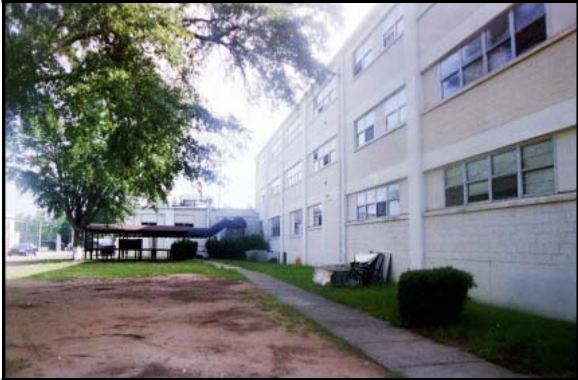
Figure 4.1.12 225-man hammerhead barracks, Bldg. 2838 (1954), Ft. Benning, view N (RCG&A).
