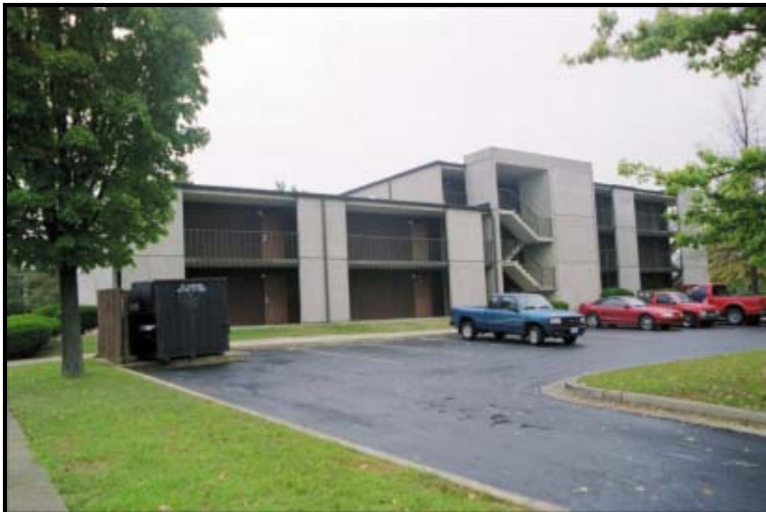
Figure 4.2.49 Apartment-type BOQ, Bldg. 2606 (1974), Ft. Knox, view NW (RCG&A).
