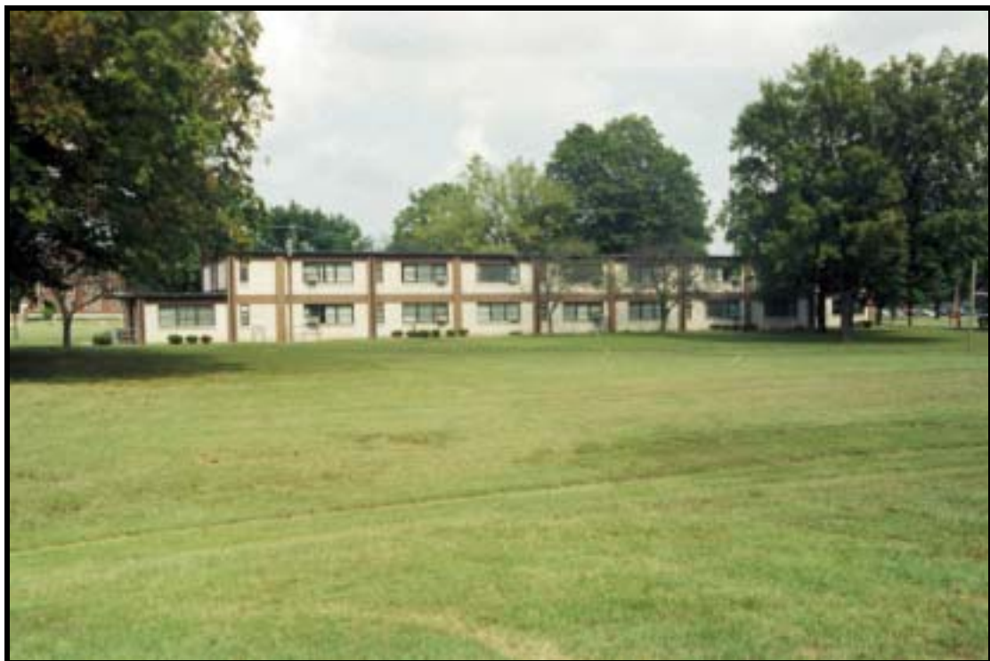
Figure 4.2.11 Two-story, hammerhead BOQ, Bldg. 1394 (1954), Ft. Knox, view NE (RCG&A).
