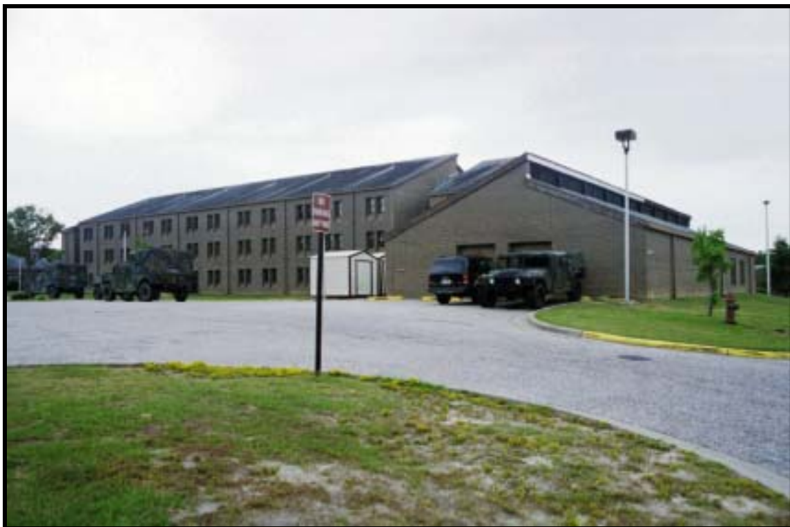
Figure 4.1.160 Quadrangle barracks, Bldg. M-3519 (1987), Ft. Bragg, view SE (RCG&A).
