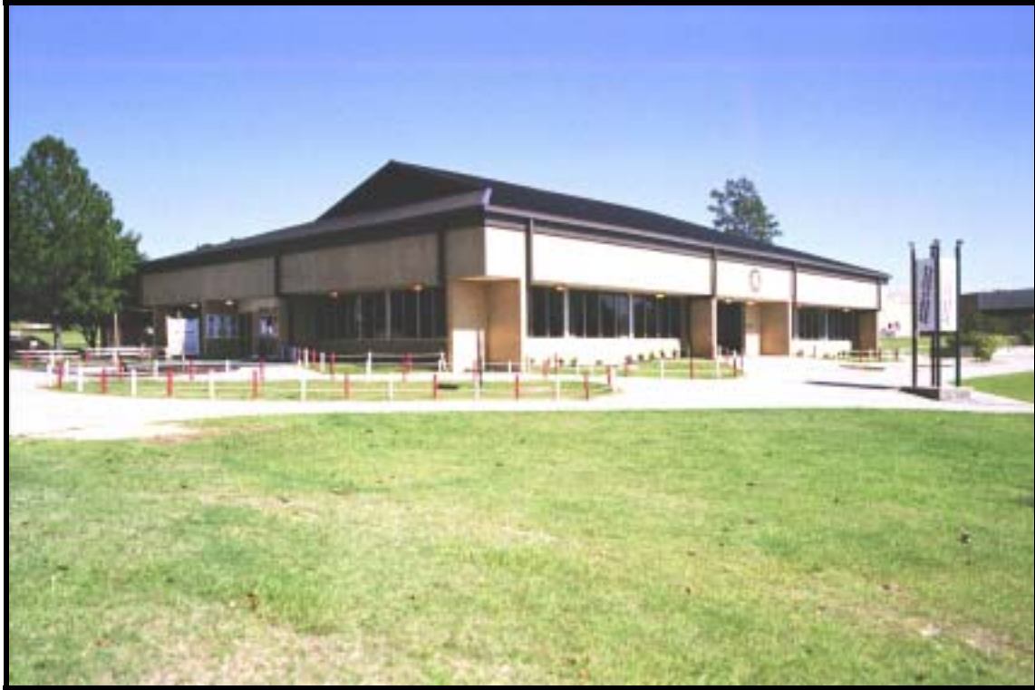
Figure 4.1.112 LBC&W dining facility, Ft. Polk, view E (RCG&A).
