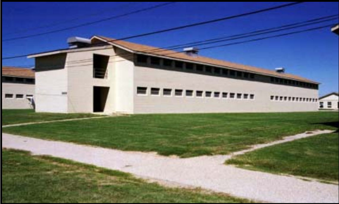
Figure 4.1.123 Two-story, Army Annual Reserve Training barracks, Bldg. 56436 (1979), North Ft. Hood, view N (RCG&A).
