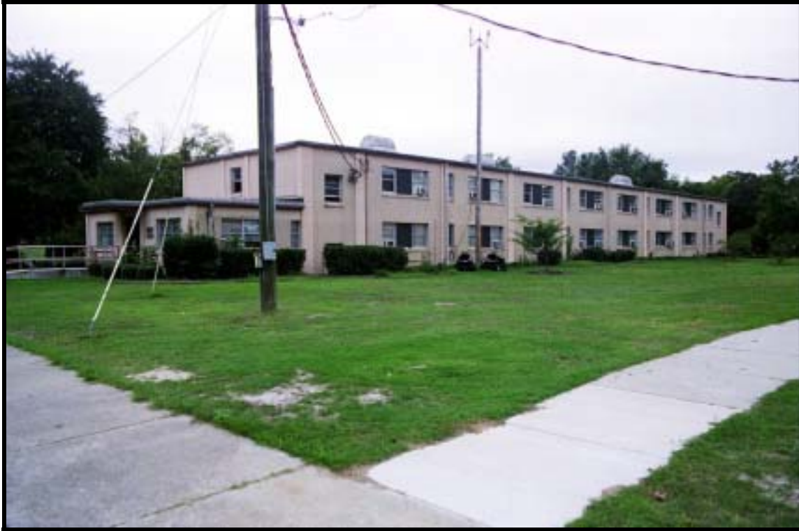
Figure 3.20 Two-story, hammerhead BOQ converted to offices, Bldg. 1-2732 (1953), Ft. Bragg, view SW (RCG&A).
