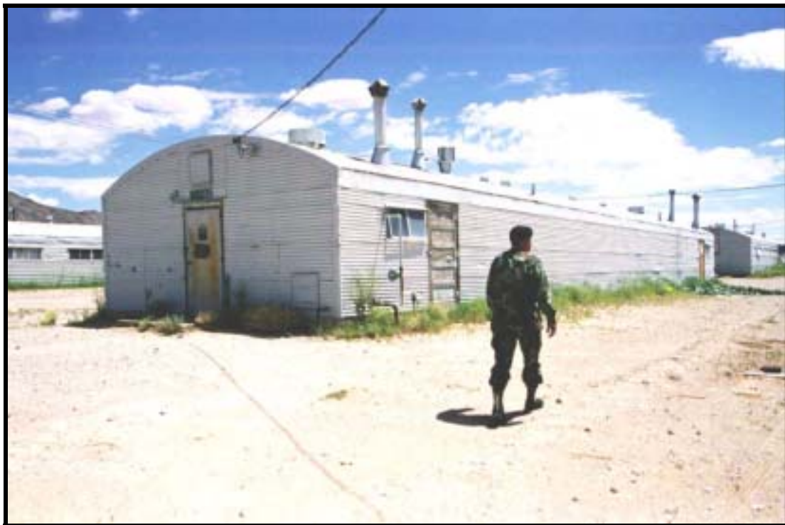
Figure 4.1.204 Mobilization latrine, Bldg. 8627 (1959), Oro Grande Range, Ft. Bliss, view E (RCG&A).
