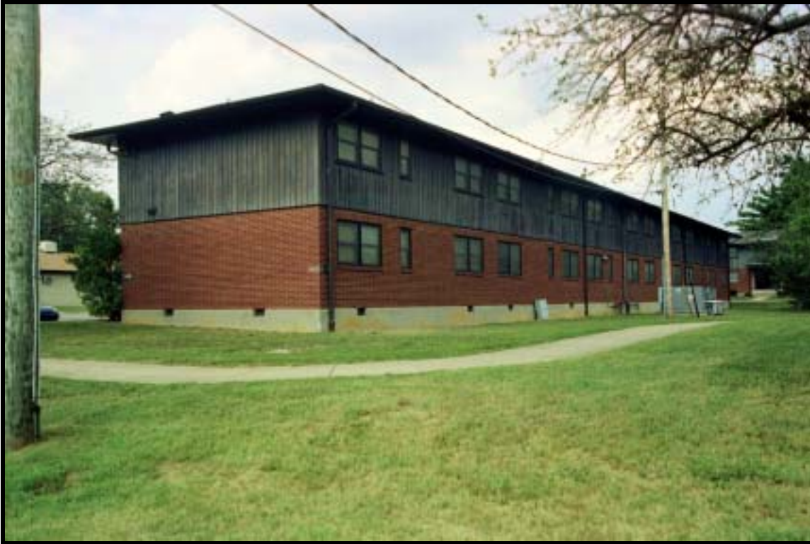
Figure 4.2.30 Two-story, apartment type BOQ, Bldg. 2446 (1962), Ft. Knox, view NW (RCG&A).
