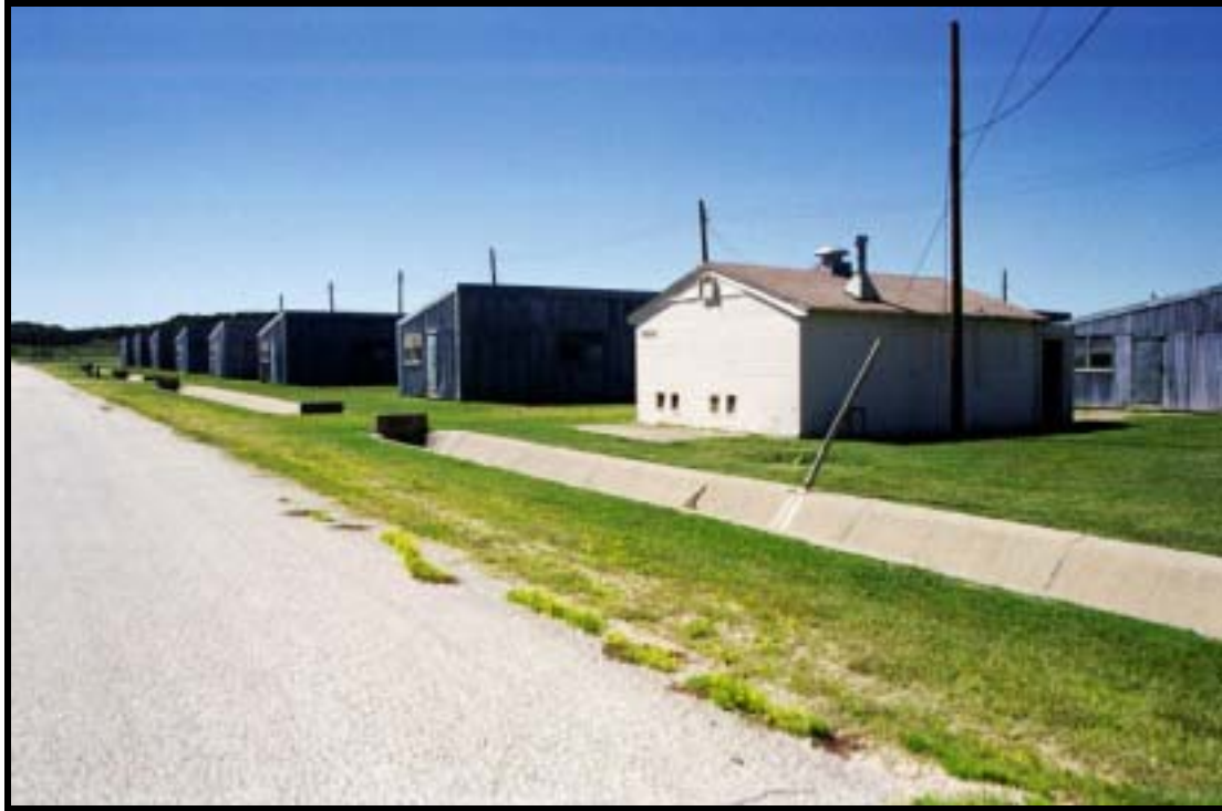
Figure 4.1.212 C-hut dining facility, Bldg. 56534 (1951), North Ft. Hood, view W (RCG&A).
