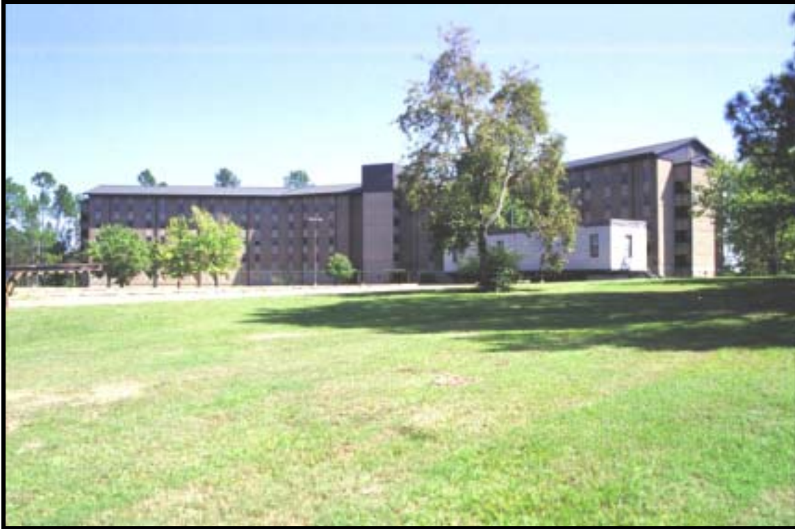
Figure 4.2.76 High Rise BOQ, Woodfill Hall, Bldg. 350 (1979), Ft. Polk, view E (RCG&A).
