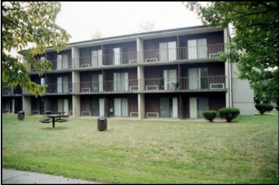
Figure 4.2.50 Apartment-type BOQ, Bldg. 2602 (1974), Ft. Knox, view W (RCG&A).
