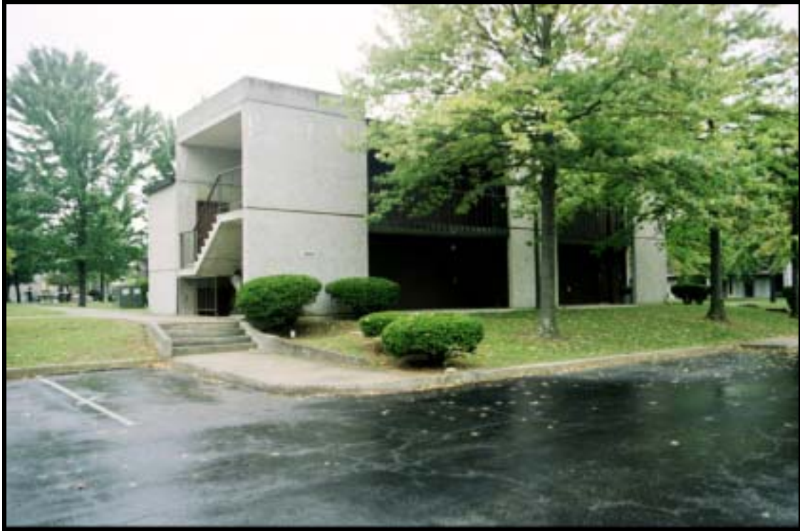
Figure 4.2.46 Apartment-type BOQ, Bldg. 2604 (1974), Ft. Knox, view SW (RCG&A).
