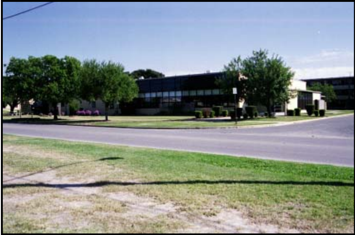
Figure 4.1.78 Rolling Pin dining facility, Bldg. 41007 (1969), Ft. Hood, view SE (RCG&A).
