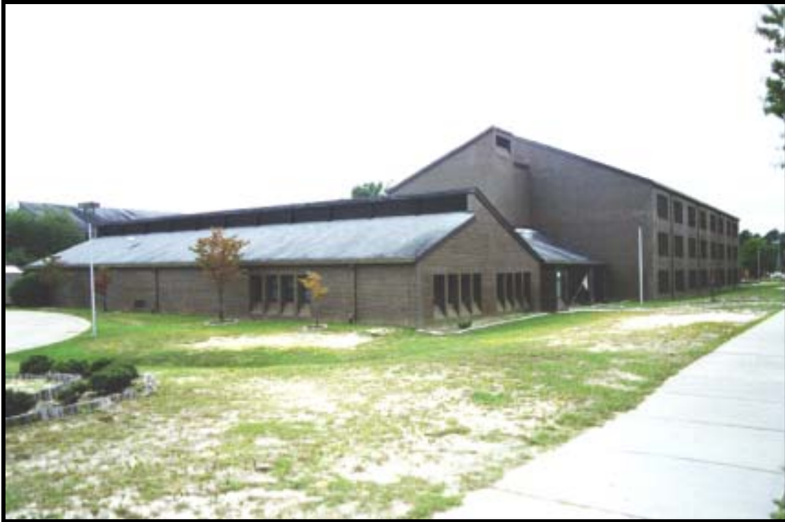
Figure 4.1.157 Quadrangle barracks, Bldg. M-4020 (1985), Ft. Bragg, view NE (RCG&A).
