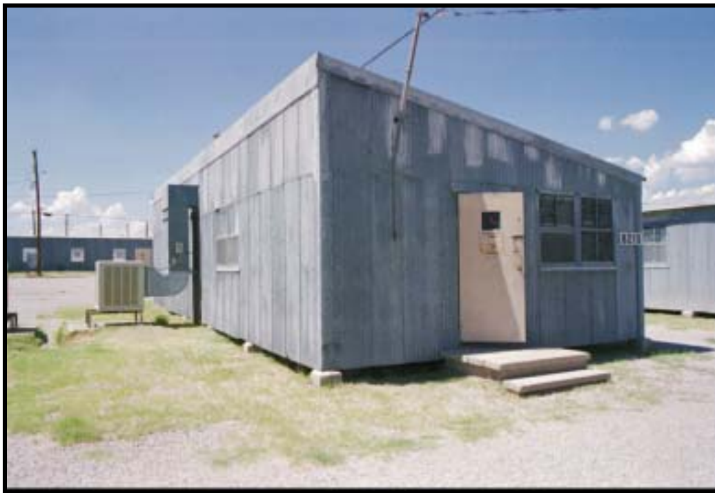
Figure 4.1.219 C-hut, Bldg. 8215 (1966), Dona Ana Range, Ft. Bliss, view NW (RCG&A).
