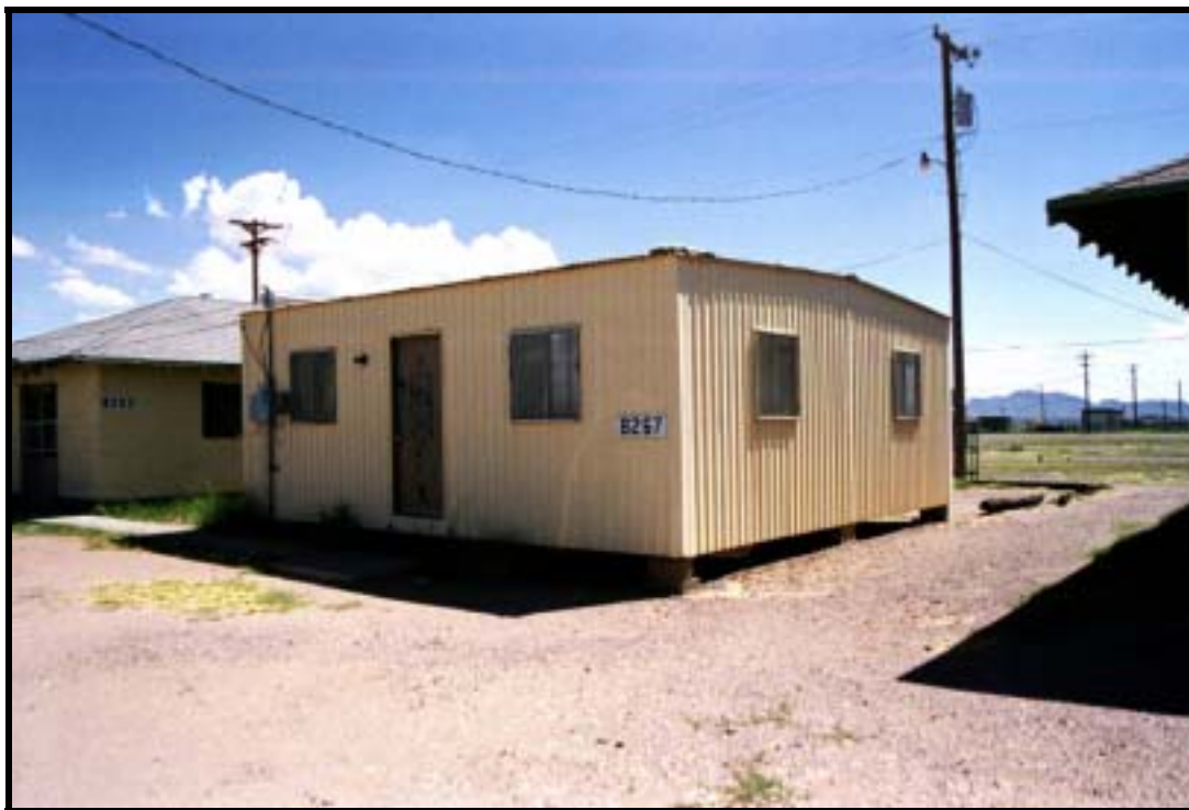
Figure 4.2.87 Mobilization BOQ, Bldg. 8267 (1983), Dona Ana Range, Ft. Bliss, view S (RCG&A).
