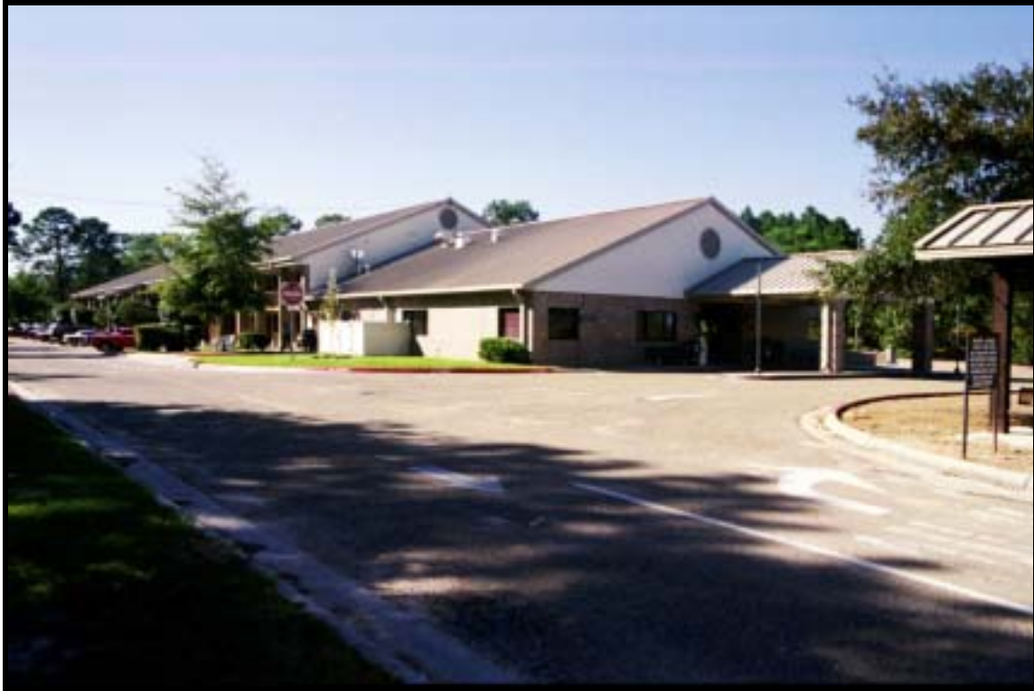
Figure 4.3.13 Transient quarter, Guest House, Bldg. 522 (1988), Ft. Polk, view NW (RCG&A).
