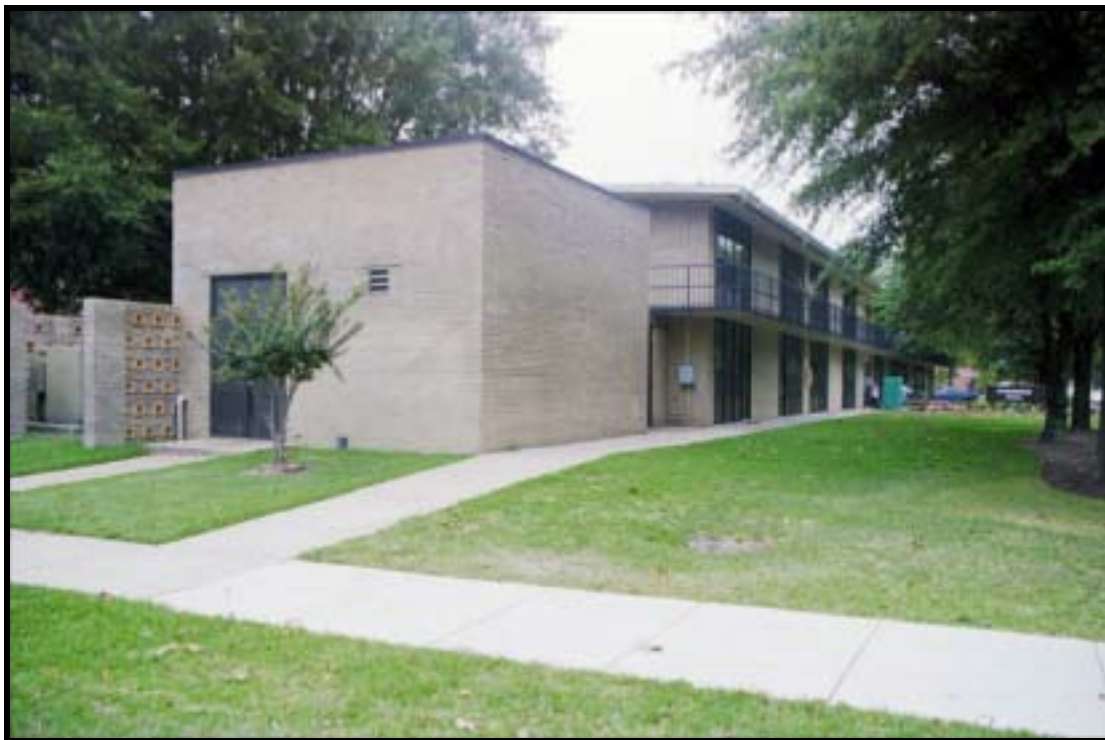
Figure 4.2.37 120-man motel-type BOQ, Bldg. 1-1939 (1968), Ft. Bragg, view NW (RCG&A).
