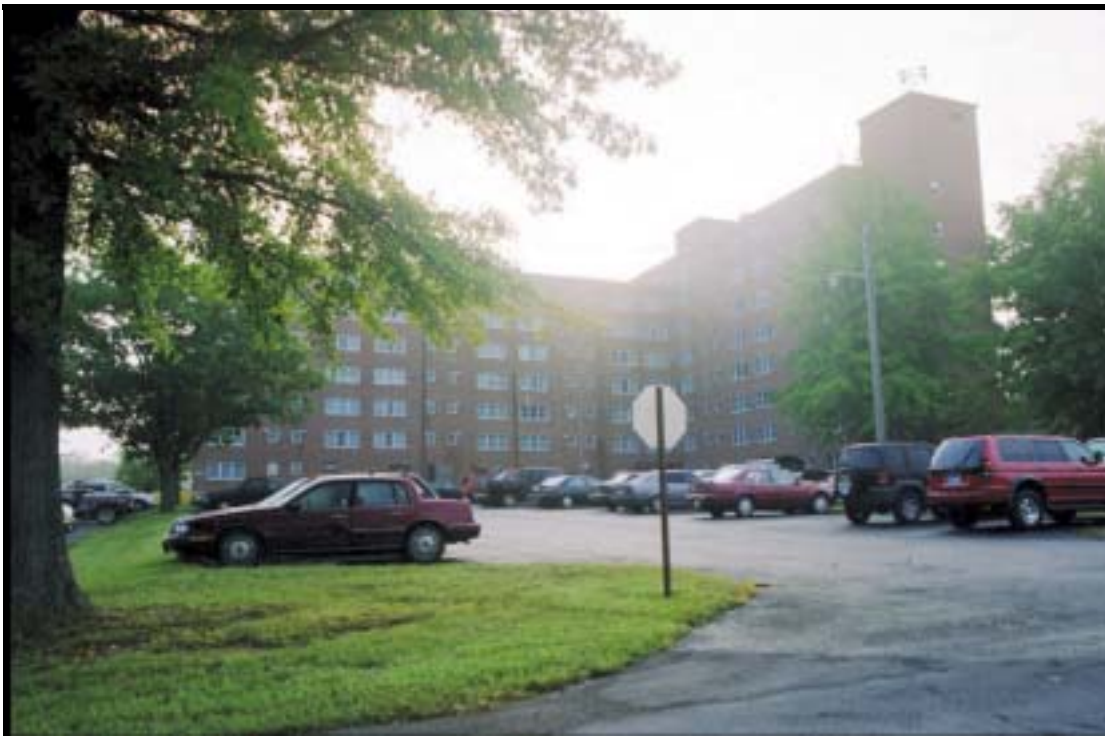
Figure 4.2.59 High Rise BOQ, New Garden Apartments, Bldg. 4770 (1958), Ft. Knox, view SE (RCG&A).
