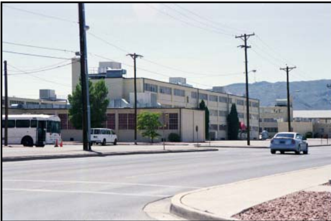
Figure 4.1.15 225-man hammerhead barracks, Bldg. 1001 (1956), Ft. Bliss, view SW (RCG&A).
