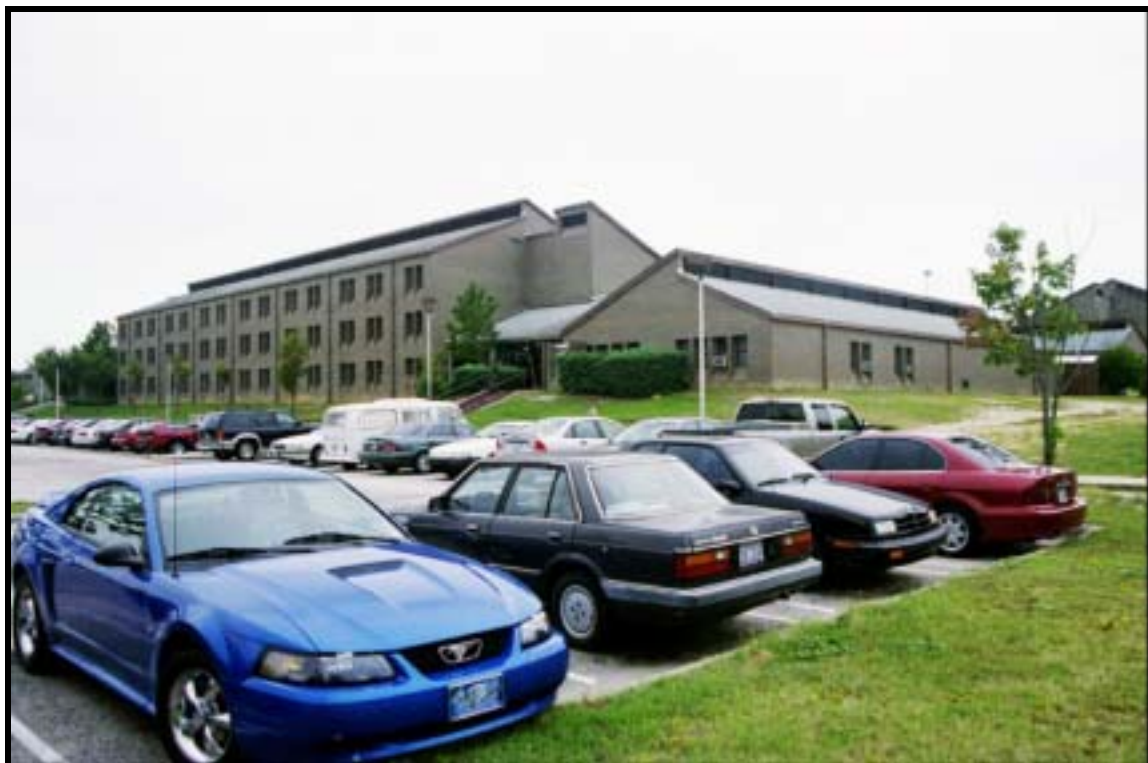
Figure 4.1.158 Quadrangle barracks, Bldg. M-3213 (1987), Ft. Bragg, view NE (RCG&A).
