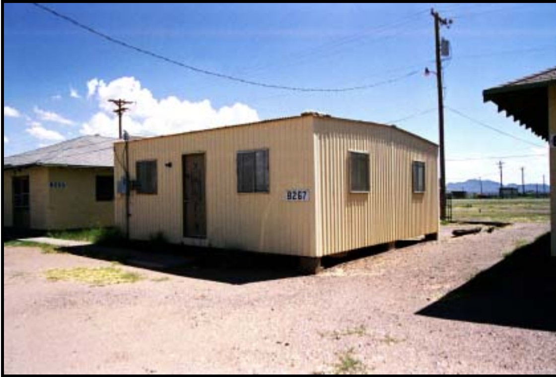
Figure 3.27 Mobilization BOQ, Bldg. 8267 (1983), Dona Ana Range, Ft. Bliss, view S (RCG&A).
