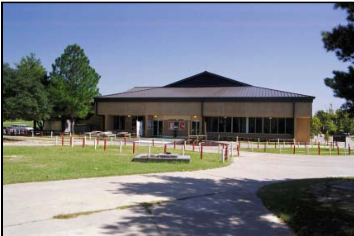
Figure 4.1.113 LBC&W dining facility, Ft. Polk, view SE (RCG&A).
