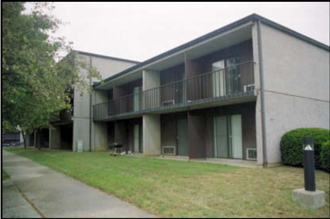
Figure 4.2.48 Apartment-type BOQ, Bldg. 2606 (1974), Ft. Knox, view NE (RCG&A).
