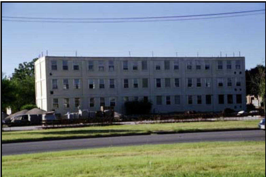
Figure 4.1.62 Renovating H-style, two-company barracks, Bldg. 9211 (1958), Ft. Hood, view S (RCG&A).
