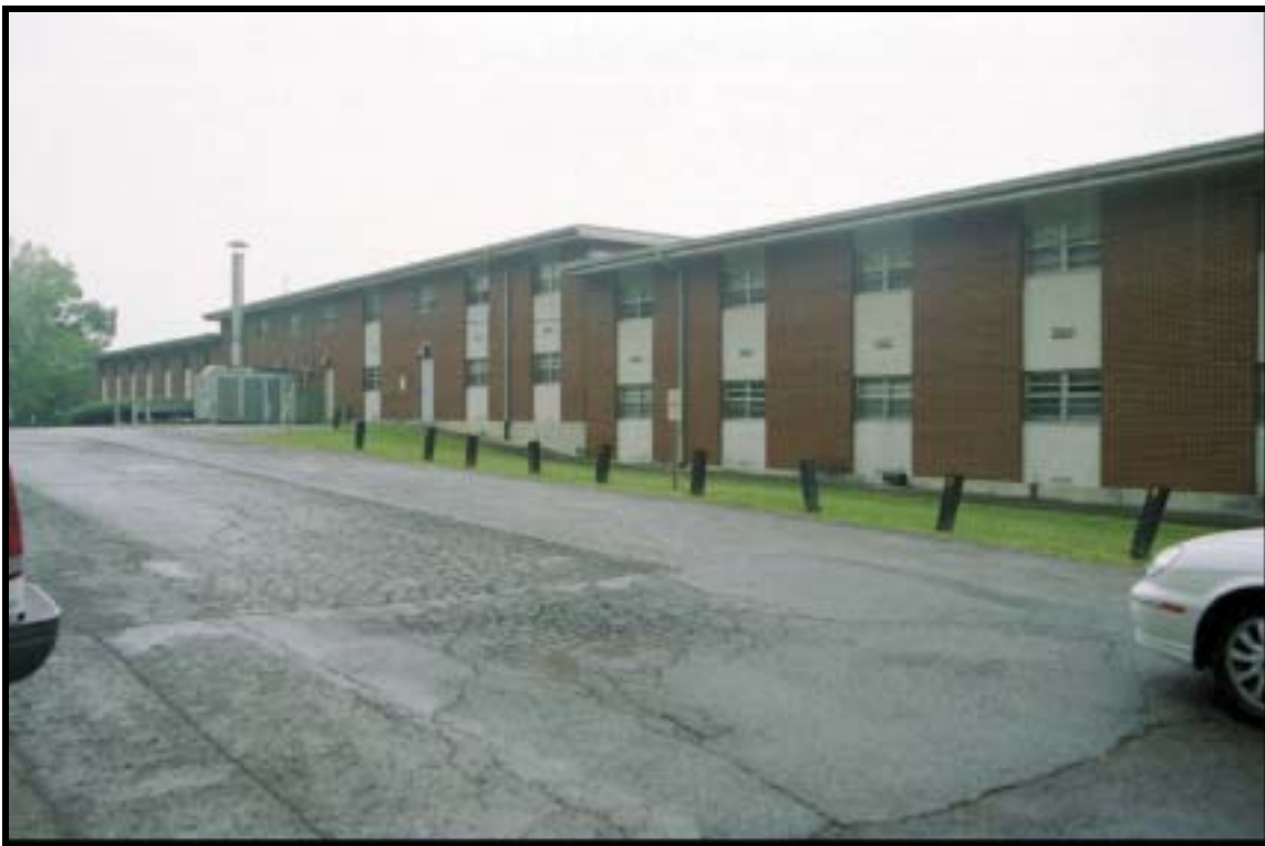
Figure 4.3.7 Transient quarter, Guest House, Bldg. 6597 (1970), Ft. Knox, view S (RCG&A).
