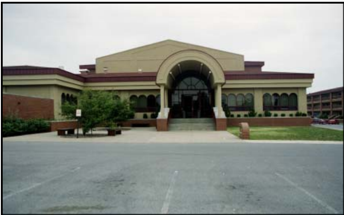
Figure 4.1.40 Totally renovated hammerhead barracks, Bldg. 1483 (1953), Ft. Knox, view E (RCG&A).
