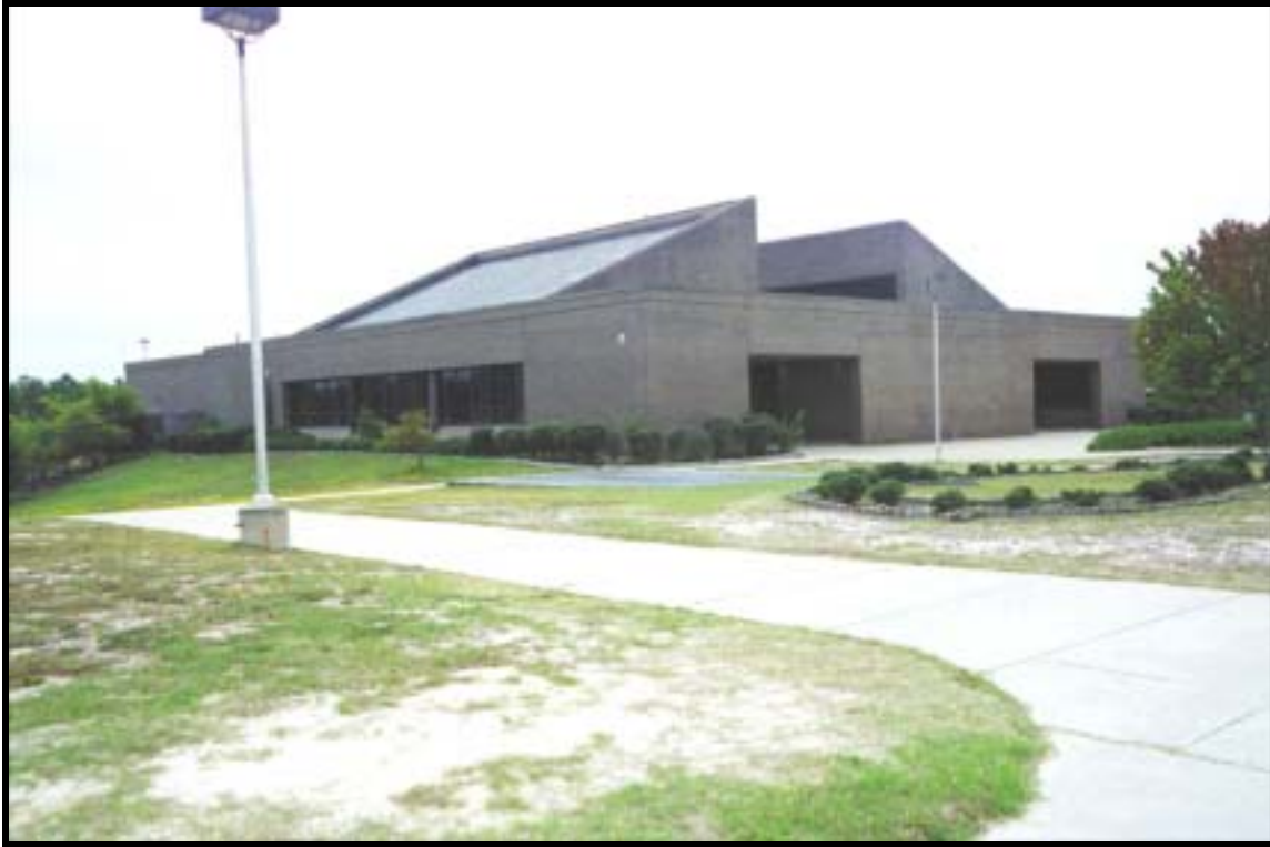
Figure 4.1.161 Quadrangle dining facility, Bldg. M-4746, Ft. Bragg, view SW (RCG&A).
