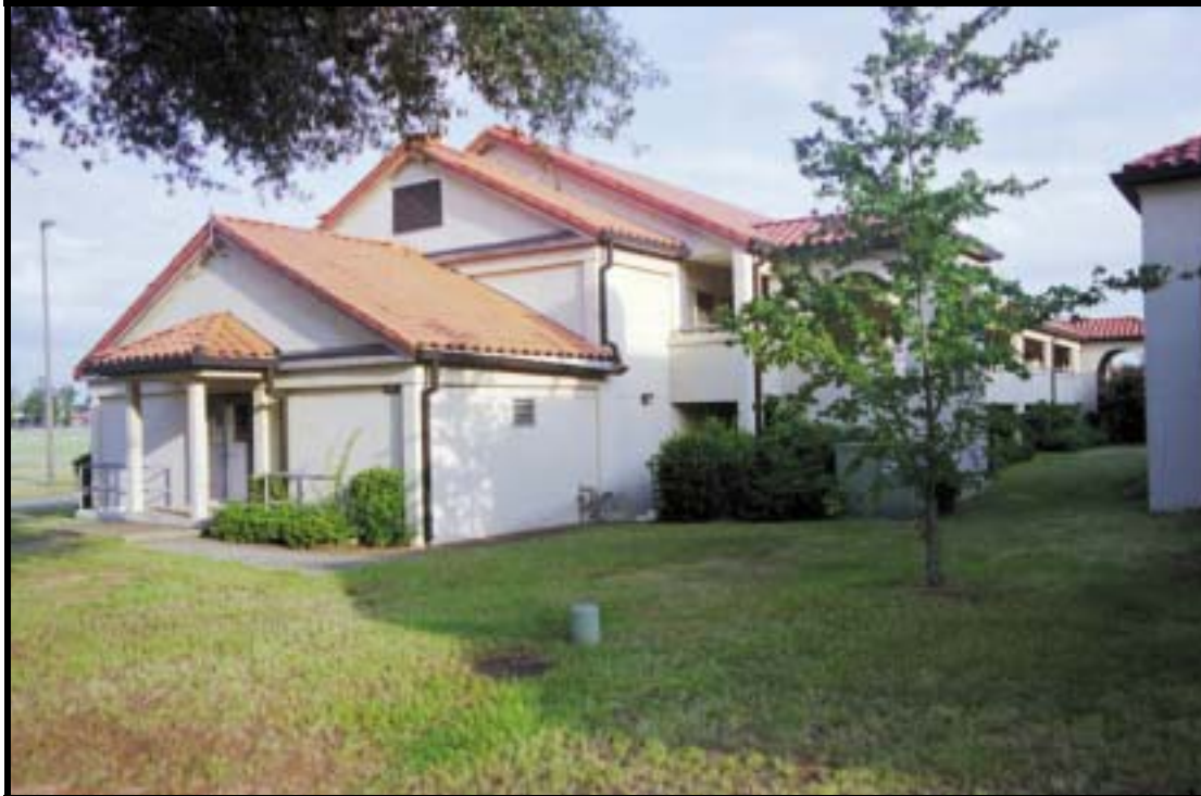
Figure 4.2.20 Renovated two-story, hammerhead UOQ, Bldg. 974 (1953), Ft. Benning, view NW (RCG&A).
