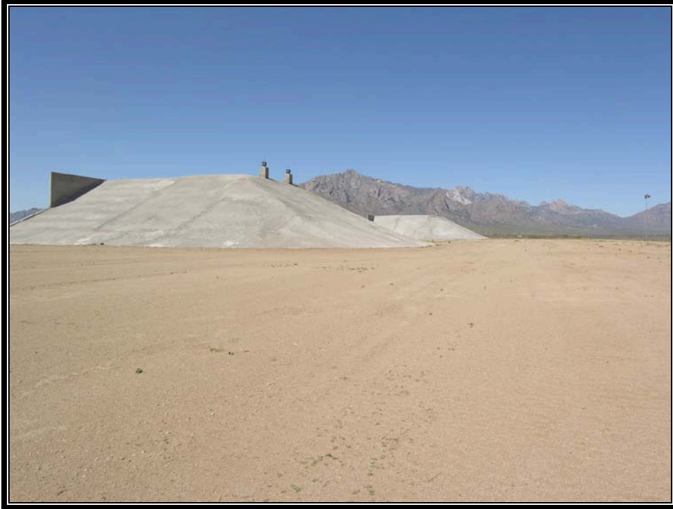
Plate 8.11 Rear of guided missile magazines showing concrete laid over earth fill (Courtesy U.S. Army, 2007)
