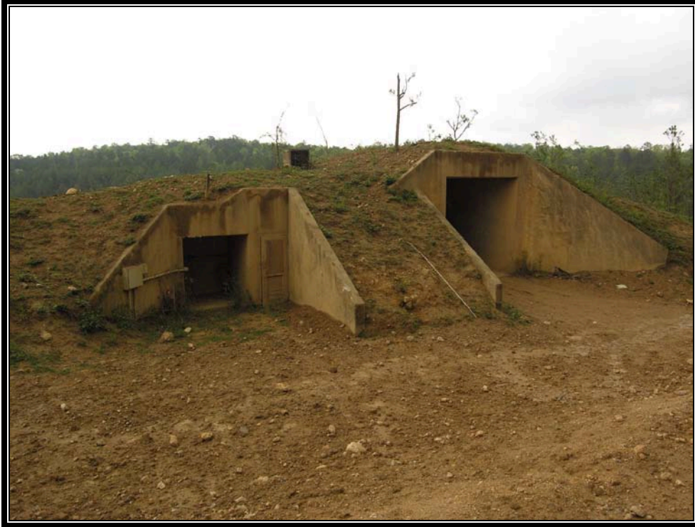
Plate 7.26 Typical personnel safety area at demolition area (Courtesy U.S. Army, 2007)
