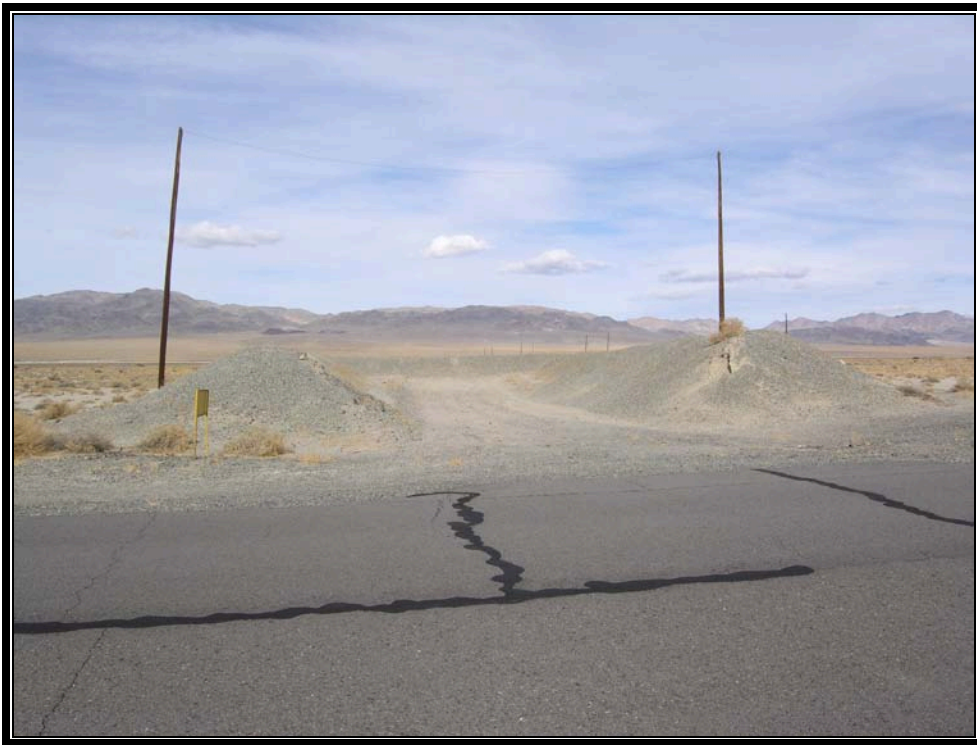
Plate 5.2 Typical open storage area with lightning protection (Courtesy U.S. Army, 2007)
