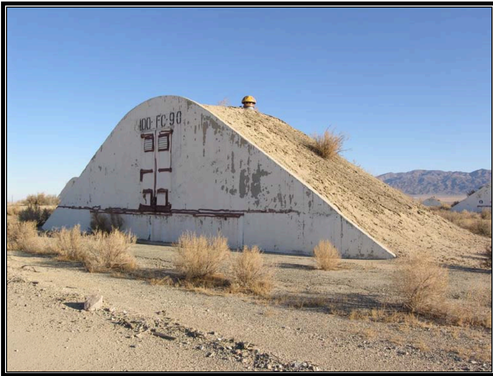
Plate 5.4 Typical fuze and detonator magazine (Courtesy U.S. Army, 2007)
