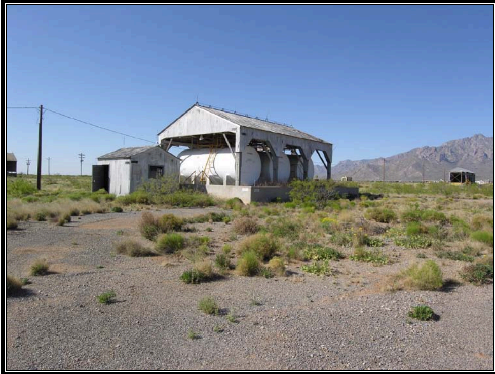
Plate 7.12 Typical liquid propellant storage building. The tanks are replacements (Courtesy U.S. Army, 2007)
