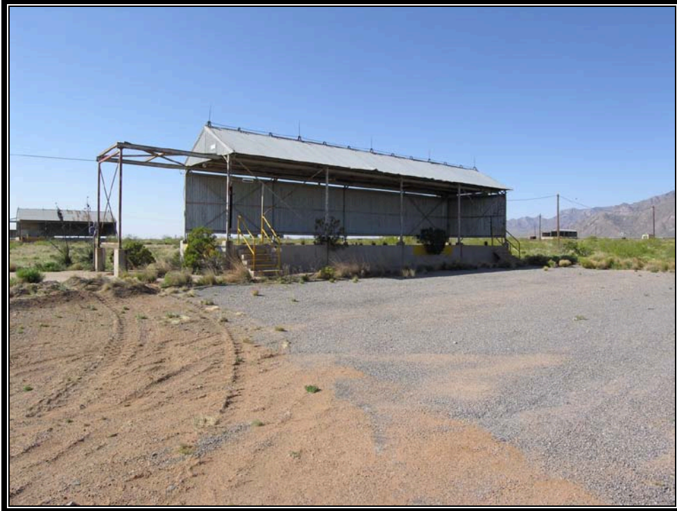
Plate 6.11 Liquid propellant storage building (Courtesy U.S. Army, 2007)
