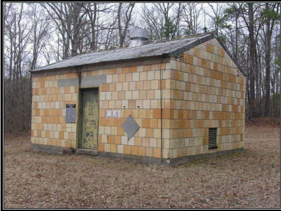
Plate 7.14 Typical aboveground ammunition storehouse (Courtesy U.S. Army, 2007)
