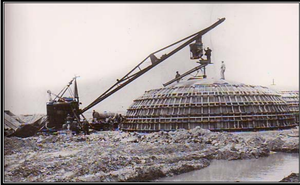
Plate 6.3 Corbetta Beehive under construction (Courtesy U.S. Army)
