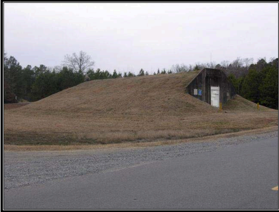
Plate 6.34 Typical igloo storage with truncated walls of the Huntsville type (Courtesy U.S. Army, 2007)
