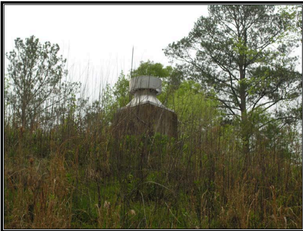
Plate 7.31 Ventilator at rear of typical Stradley magazine (Courtesy U.S. Army, 2007)
