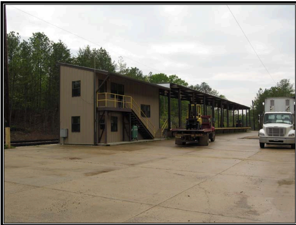
Plate 7.27 Typical explosives transfer building and loading dock showing enlarged office building and modified canopy over dock (Courtesy U.S. Army, 2007)
