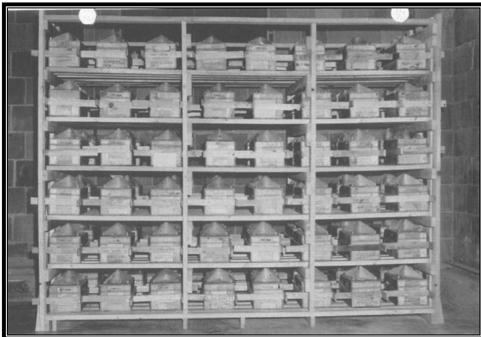
Plate 7.7 Rack designed for storage of NIKE missile batteries (Sierra Ordnance Depot 1955:n.p.)
