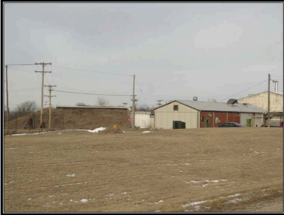
Plate 5.5 Typical earth-barricaded ready magazine, left (Courtesy U.S. Army, 2007)
