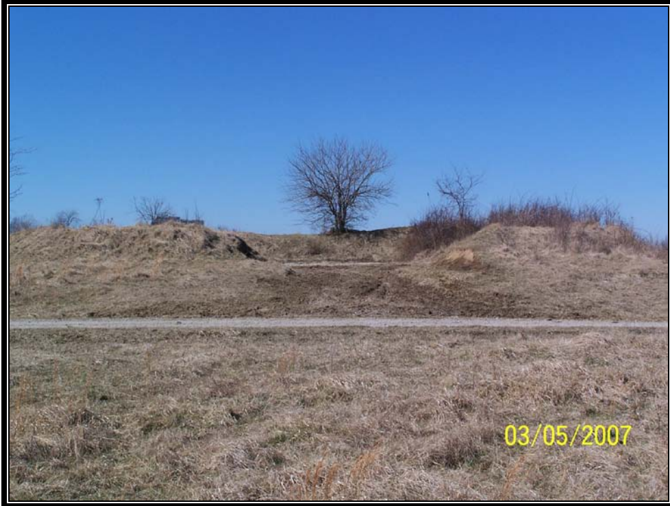
Plate 5.1 Typical open storage area (Courtesy U.S. Army, 2007)
