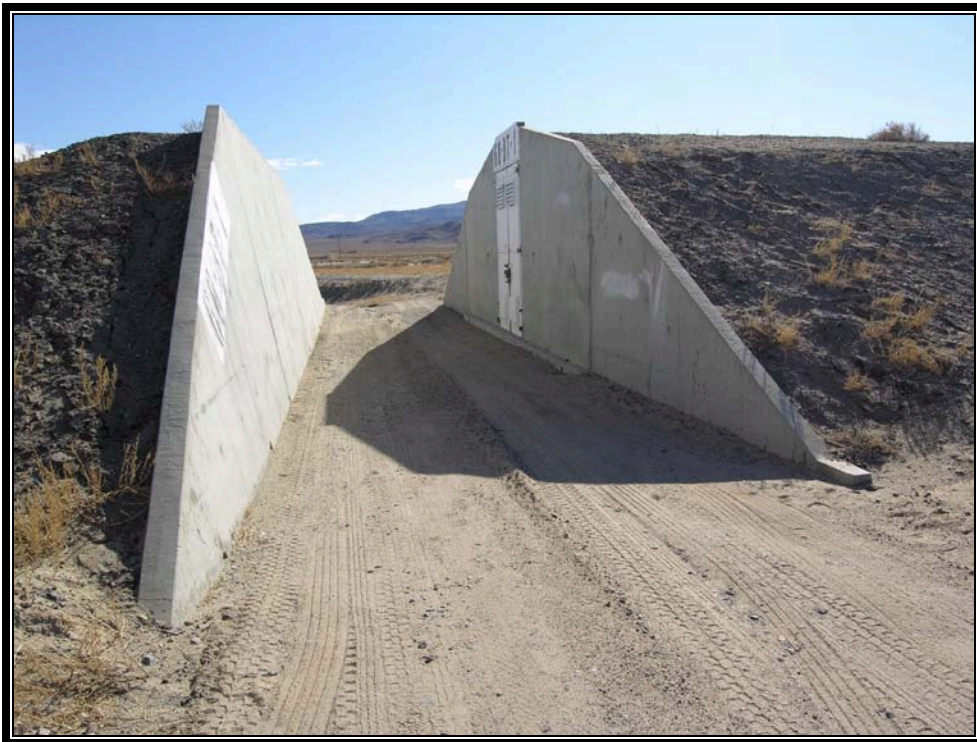
Plate 6.17 Typical concrete barricade opposite magazine entrance (Courtesy U.S. Army, 2007)
