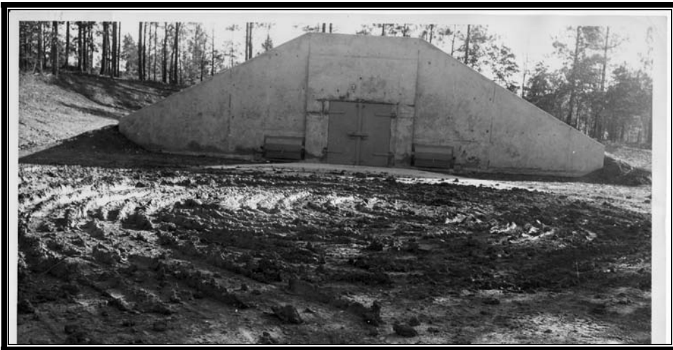
Plate 6.35 New igloo storage, ca. 1953 (Courtesy U.S. Army)
