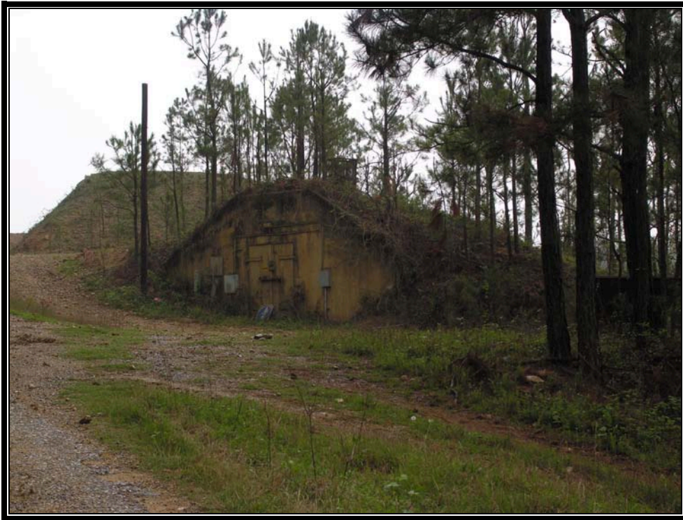
Plate 7.25 Typical installation-level magazine for fuze and detonator storage (Courtesy U.S. Army, 2007)
