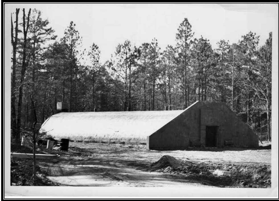
Plate 6.32 Typical newly-constructed igloo storage, ca. 1953 (Courtesy U.S. Army)
