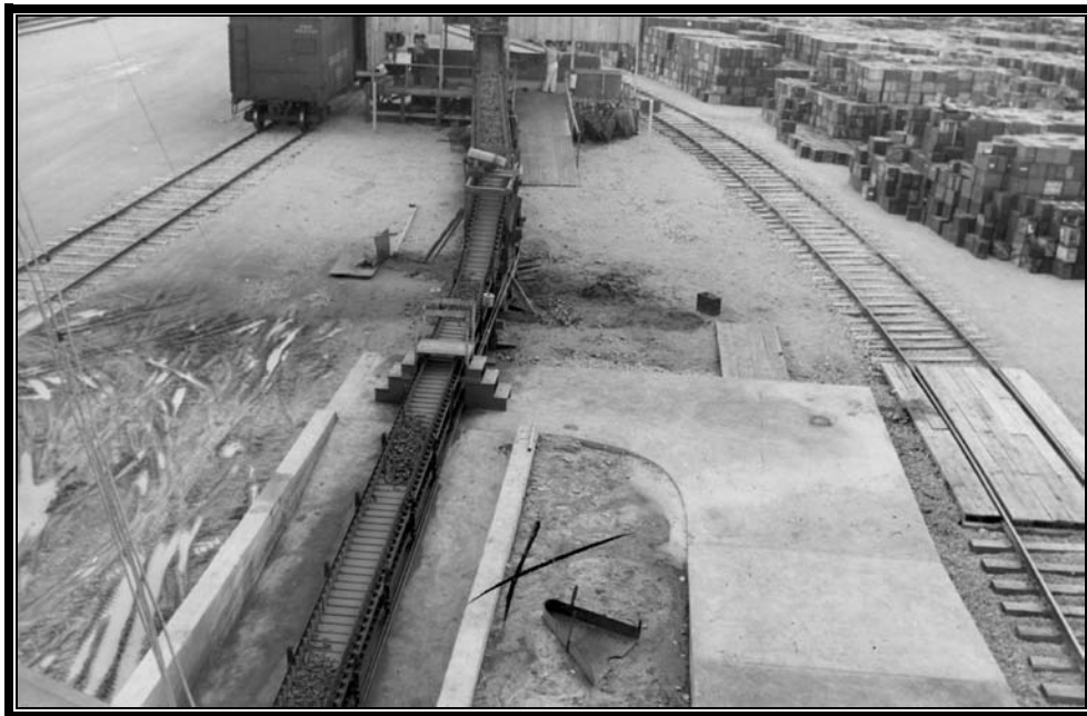
Plate 7.21 Typical conveyor leading to popping plant where brass casings were heated to remove any residual explosive, ca. 1945. Note large volume of ammunition boxes to right of image (Courtesy U.S. Army)
