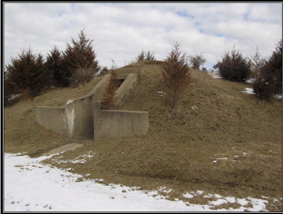
Plate 6.5 Typical hillside magazine, also referred to as frost proof (Courtesy U.S. Army, 2007)
