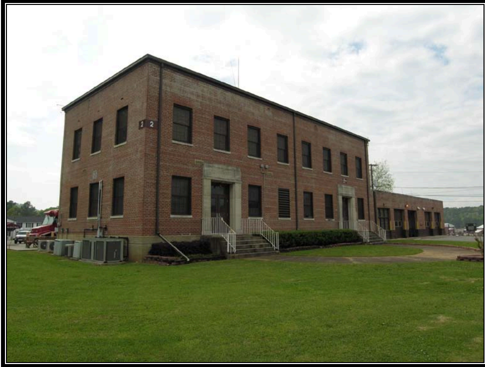
Plate 7.24 Typical World War II era dispensary, guard house, and fire station (Courtesy U.S. Army, 2007)
