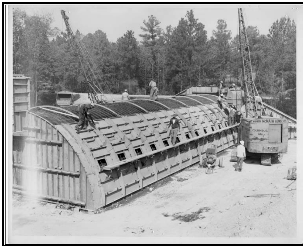
Plate 6.2 Igloo construction, ca. 1953 (Courtesy U.S. Army, 2007)
