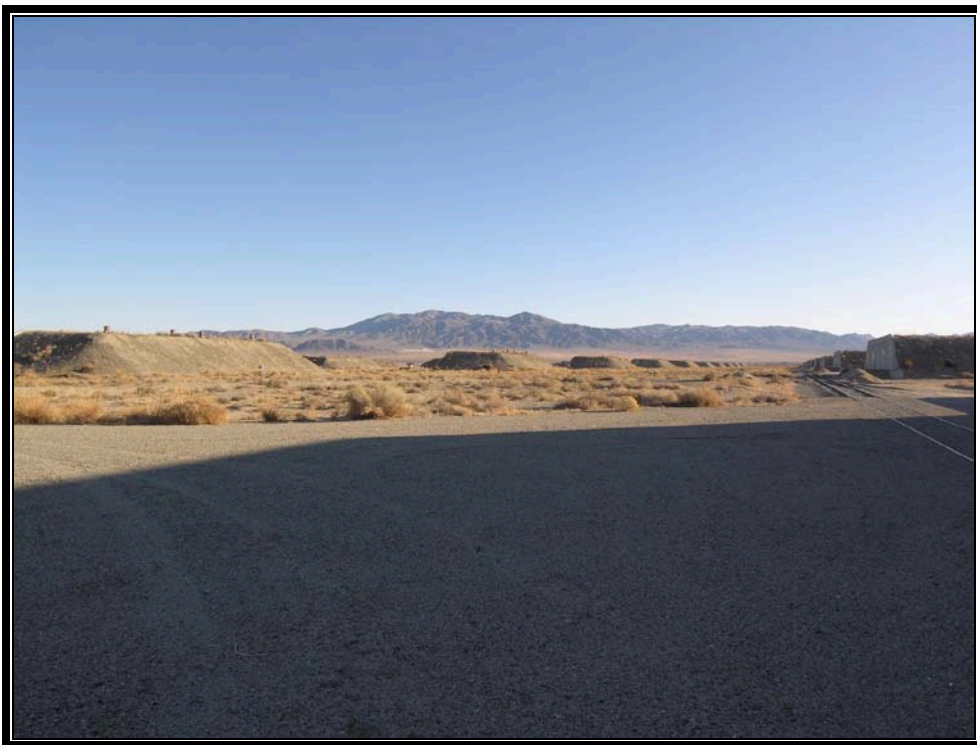
Plate 6.37 Typical earth-covered, rectangular smokeless powder magazines (Courtesy U.S. Army, 2007)
