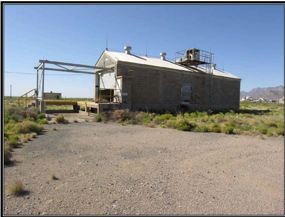
Plate 6.12 Liquid propellant storage building, note lightning rods (Courtesy U.S. Army, 2007)
