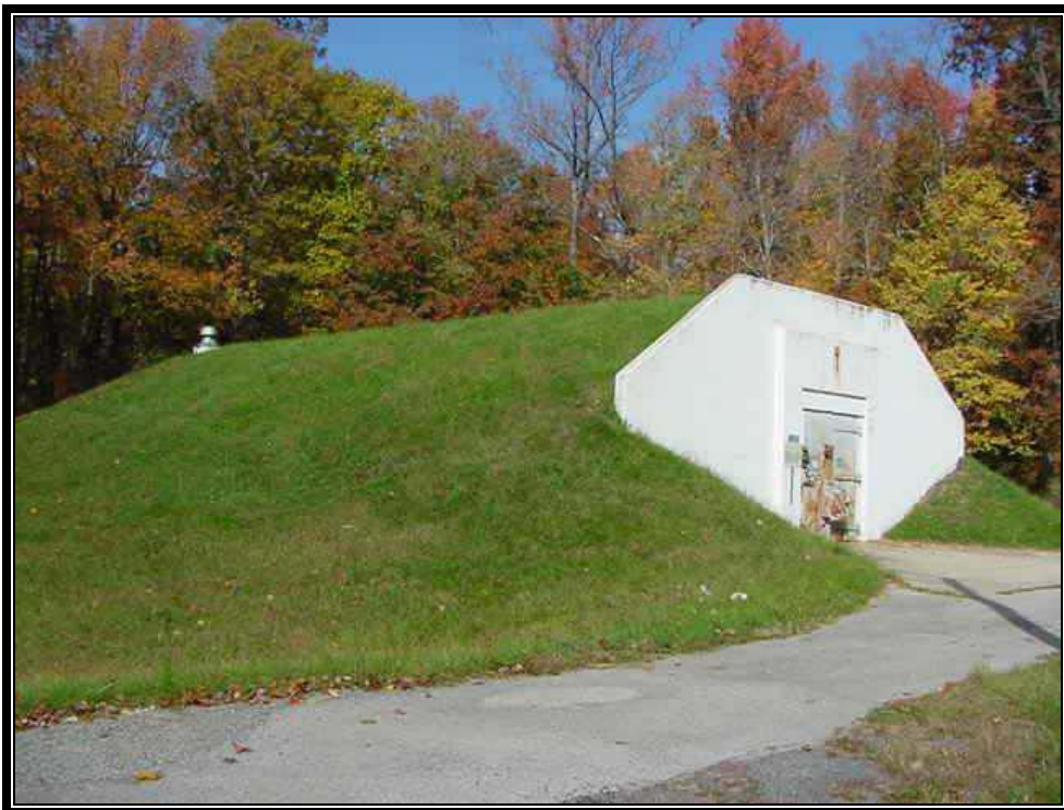
Plate 7.11 Typical igloo storage (Courtesy U.S. Army, 2007)
