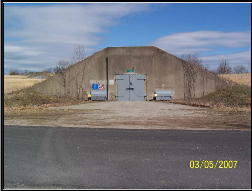
Plate 6.36 Typical igloo storage with long wing walls (Courtesy U.S. Army, 2007)
