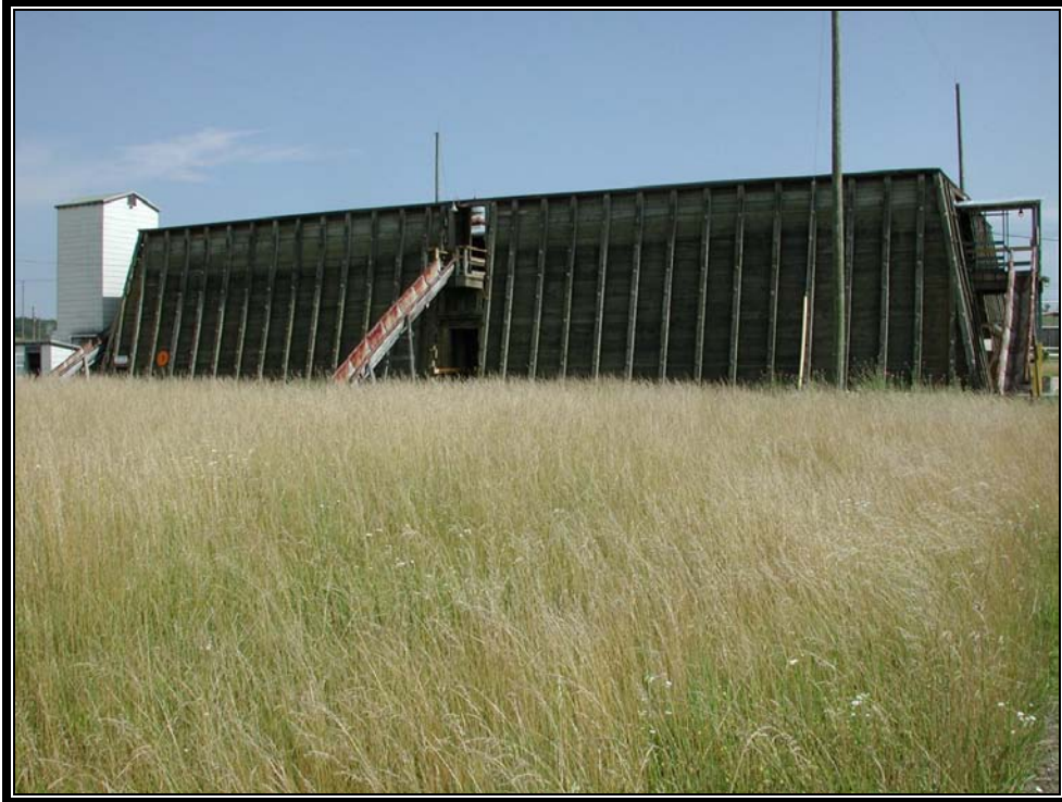
Plate 6.16 Typical smokeless powder storage building surrounded by rampauno barricade (Courtesy U.S. Army, 2007)
