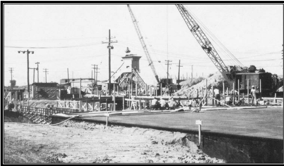
Plate 6.6 Construction of subterranean magazine (Courtesy U.S. Army)
