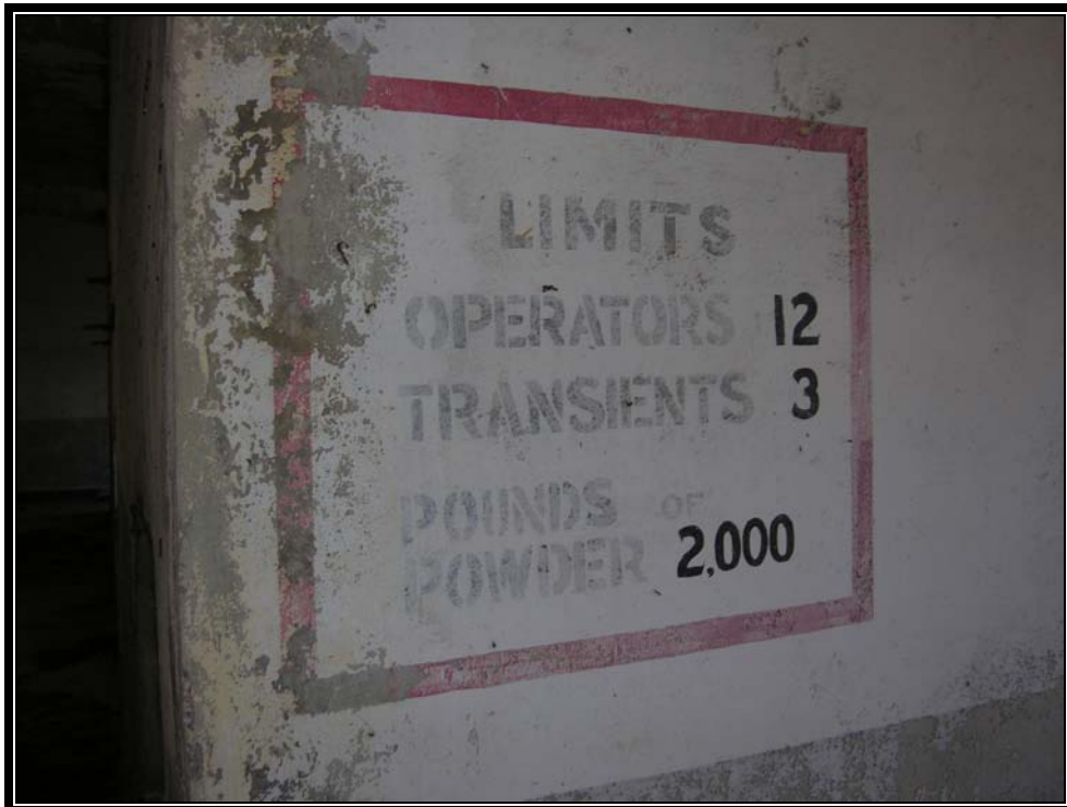
Plate 6.25 Typical signage indicating limits on numbers of operating personnel, transient personnel, and maximum amount of explosives allowed in an area (Courtesy U.S. Army, 2007)
