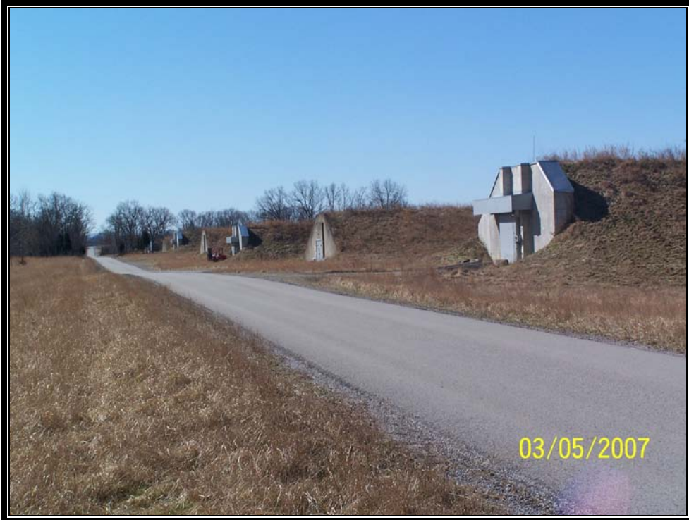
Plate 6.38 Typical igloo storage constructed during 1953 showing original, Huntsville types with new igloos built between (Courtesy U.S. Army, 2007)
