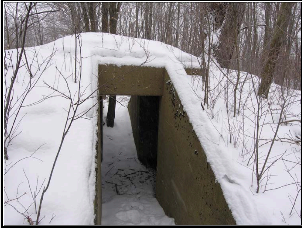
Plate 7.22 Typical safety shelter, or foxhole (Courtesy U.S. Army, 2007)
