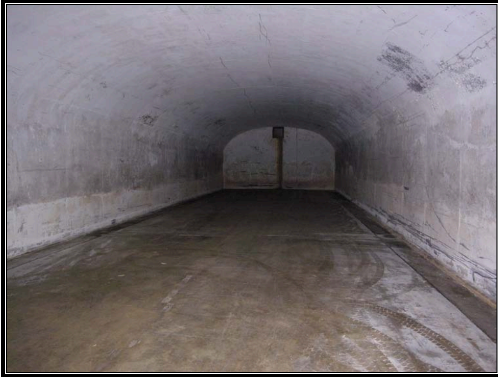
Plate 7.28 Typical interior of Stradley magazine (Courtesy U.S. Army, 2007)
