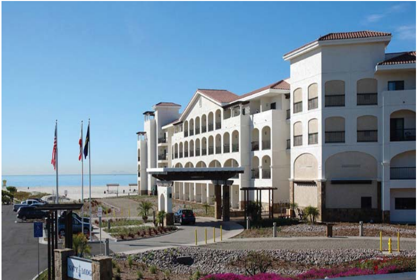
Navy Lodge, North Island Naval Air Station
