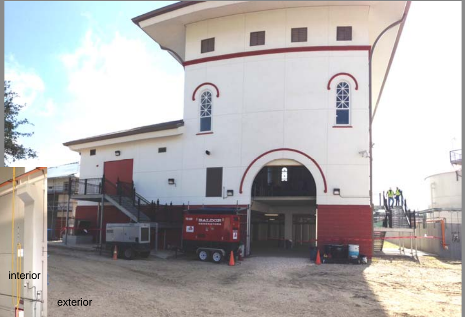
Orleans 15-megawatt New Generator Building Storm Proofing
