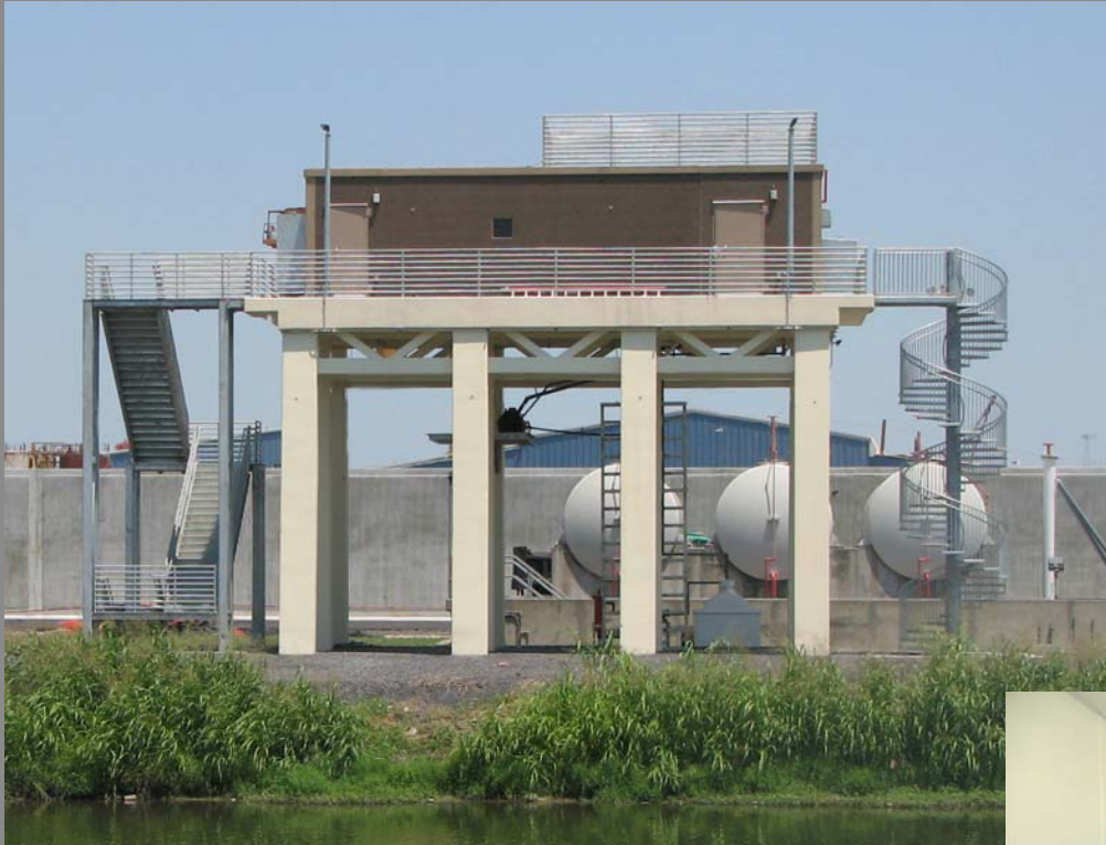
Hero Canal Pump Station New Safe Room, exterior and interior
