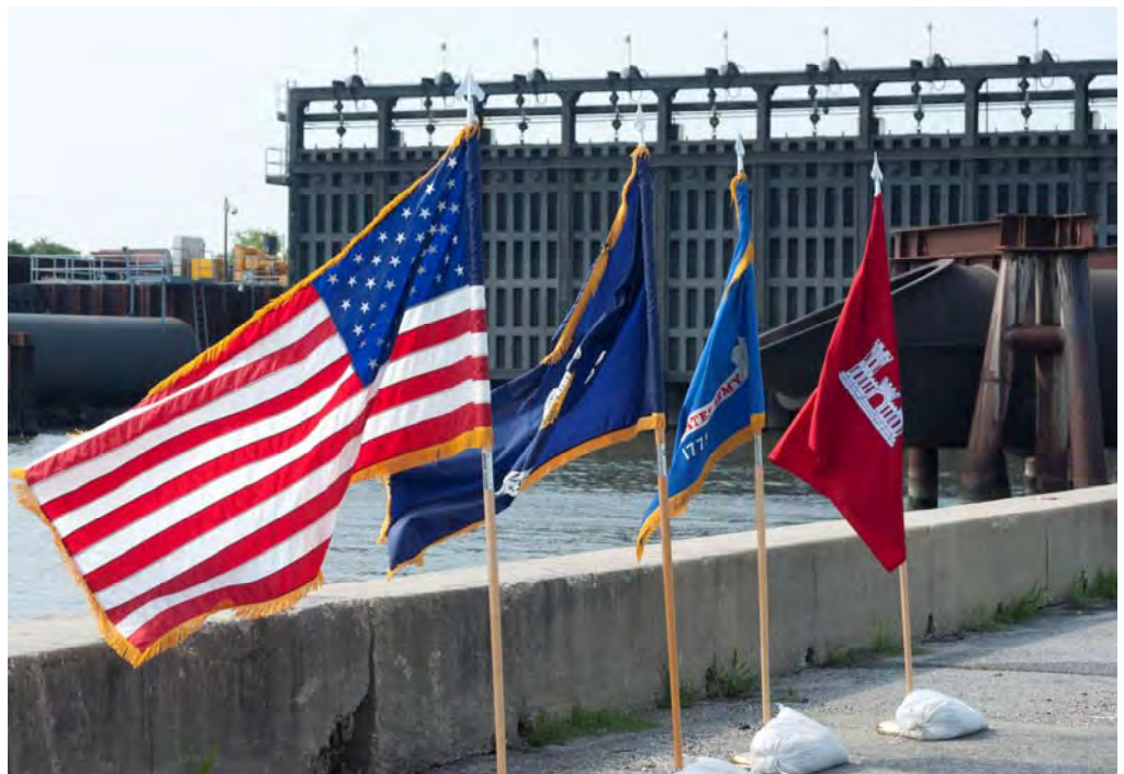
Ceremonial flags at the 17th Street Outfall Canal mark the location for the groundbreaking activities that announced the start of construction for the Permanent Canal Closures and Pumps, one of the largest contracts in the HSDRR USACE Photo by Patti Geistfeld
