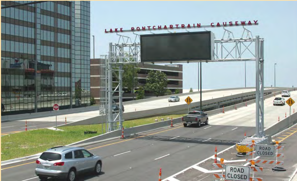
The historic canopy lights at the Lake Pontchartrain Causeway Bridge were reinstalled on June 10. It was the final touch to a $43 million HSDRRS construction project that had some very interesting aspects to it.
