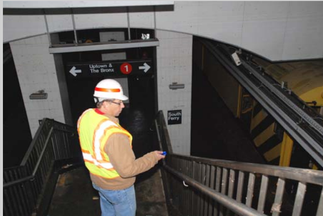
Mark Gonski, New Orleans District, inspects a flooded subway station in Manhattan as part of the Corps' unwatering efforts.
