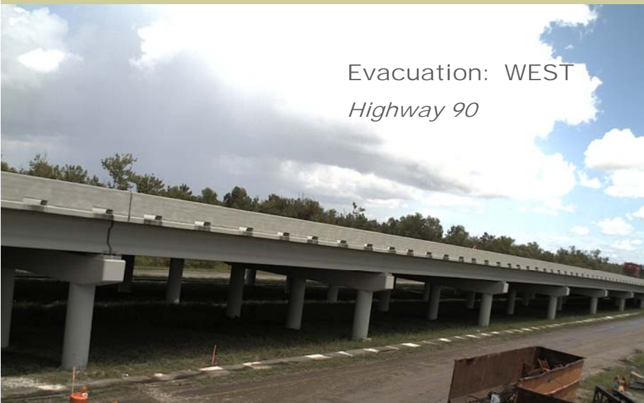
This is the new Hwy. 90 bridge that passes over a new floodwall which is part of the recently completed Western Tie-In section of the HSDRRS. USACE Photos
