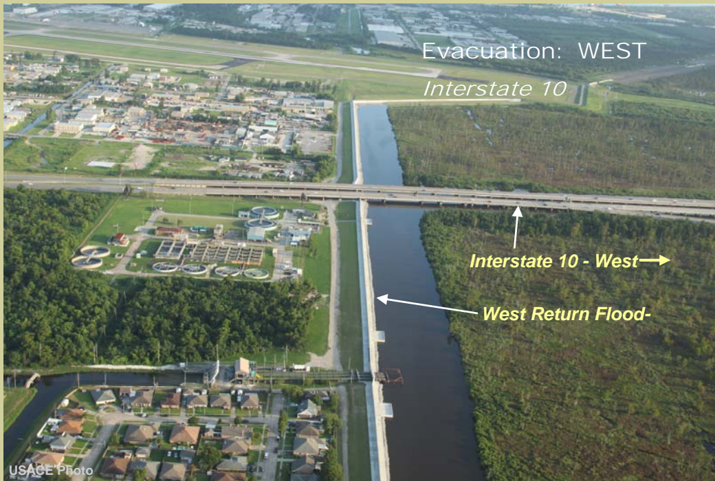
Vehicles travelling west during a tropical storm evacuation will pass over the West Return Floodwall, a concrete T-wall that straddles the Jefferson Parish/St. Charles Parish line.
