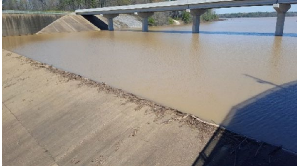
Lake Arkabutla overtopped March 31. Project Office personnel continue 24-hour surveillance of the dam and spillway to monitor conditions. The lake will be drawn down slowly and deliberately over the next several months in order to regain storage capacity.
