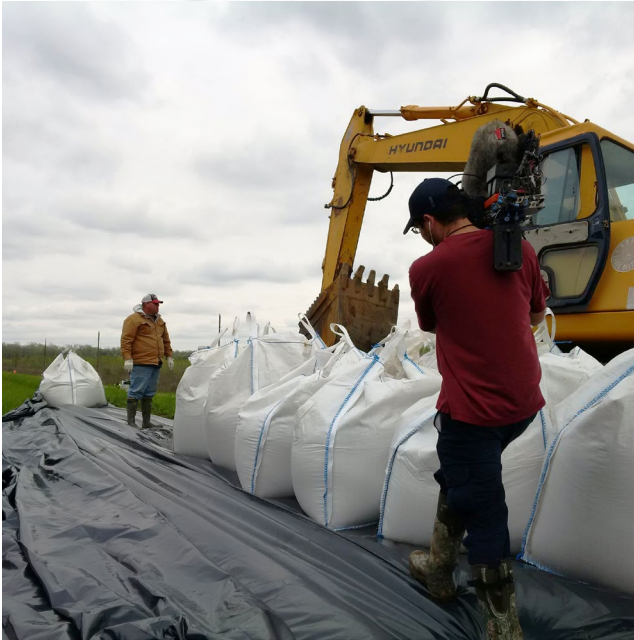
Workers place and reinforce super sacks in Brouillette, Louisiana, along the Red River Mar. 17.
