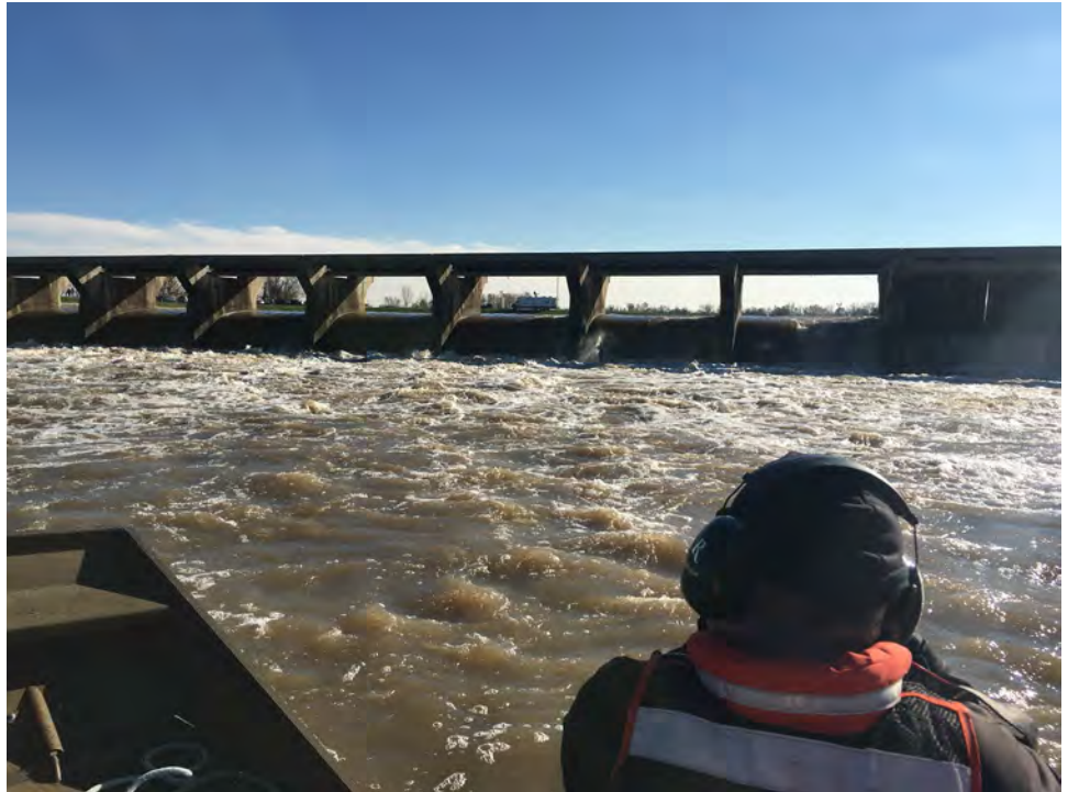
Opening of the Bonne Carre' Spillway in Louisiana, Jan. 10.
