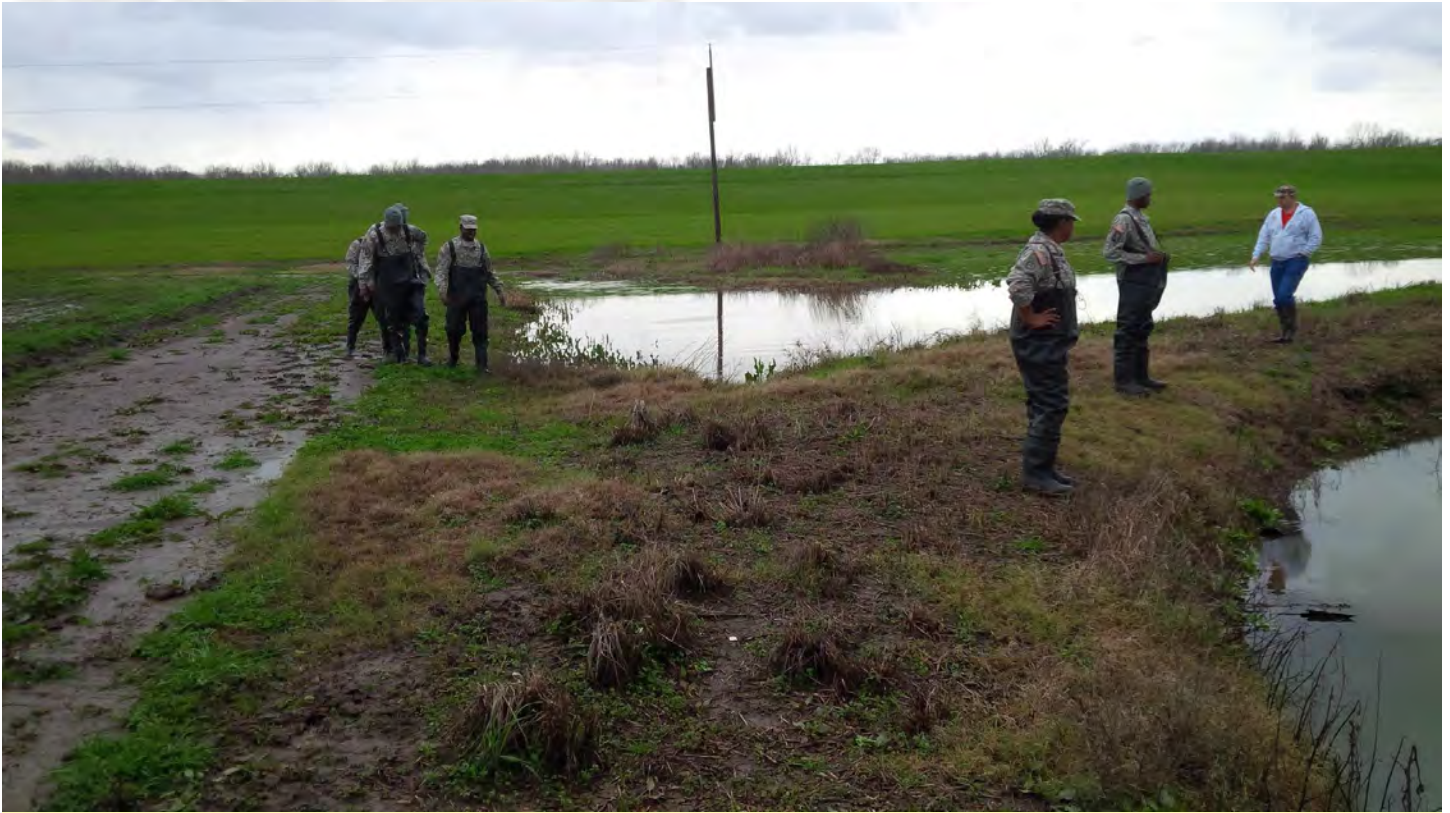
Boots on the ground: Soldiers from the Louisiana National Guard patrolling levees alongside the Corps of Engineers and local authorities to help spot any signs of trouble. Here, troops and Corps personnel inspect damage from cattle on a levee near Davis Island and a sand boil near Hodge.
