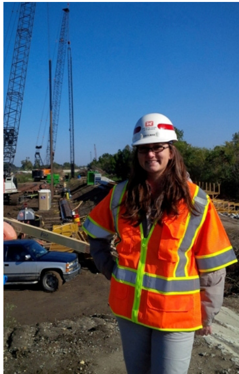
Pictured is Lacie Davilman, Project Engineer Team Leader, New Orleans Area Office.
