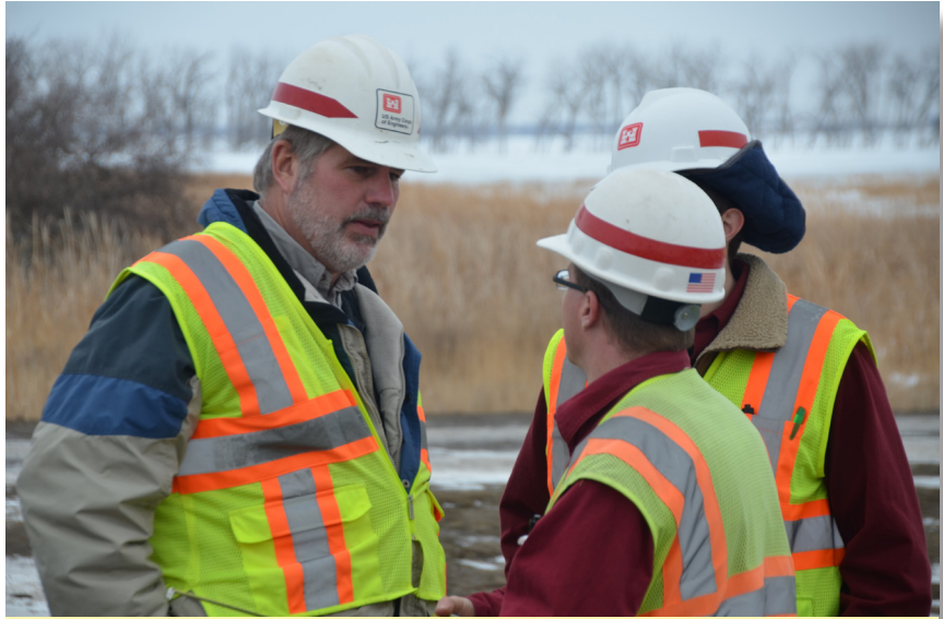
Pictured above —Loren Nishek (left), St. Paul District senior project engineer, at a construction site in Devils Lake, N.D. Photo by Patrick Moes, St. Paul District
