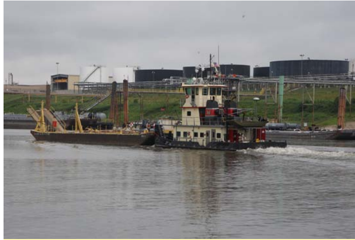
Pictured is the Vicksburg District's Mat Sinking Unit.
