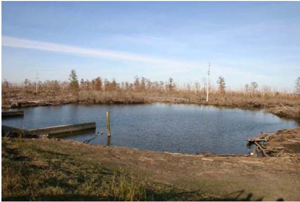
Figure 3. Station Sed 10 at Pump Station Meraux 4
