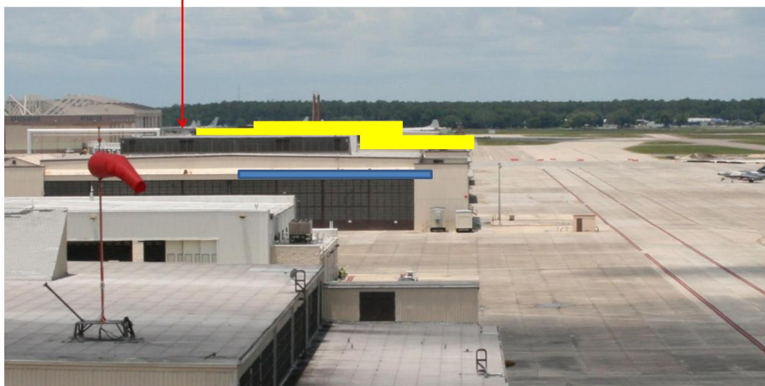
Figure 2-3: Removal of Hangars 113, 114, and 115 increases visibility of ramp areas and taxiway (yellow indicates visual obstruction which would be removed)
