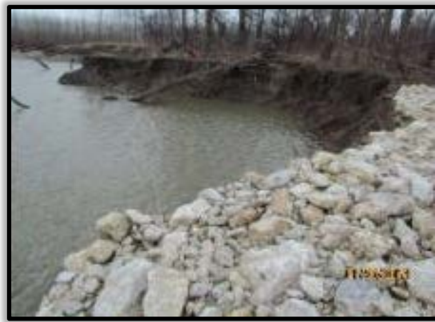
Revetment and dike damage
